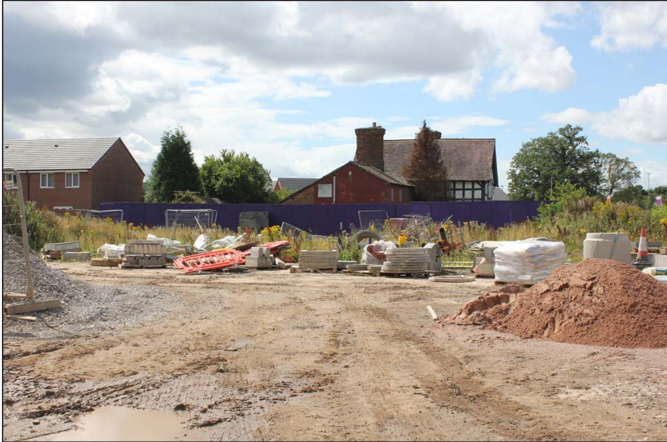
Plate 03: Proposed development area northeast of Yew Tree Farm grade II Listed Building, from the northeast.
