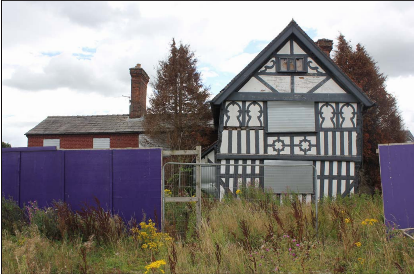
Plate 01: Yew Tree Farm grade II Listed Building, from the northwest.
