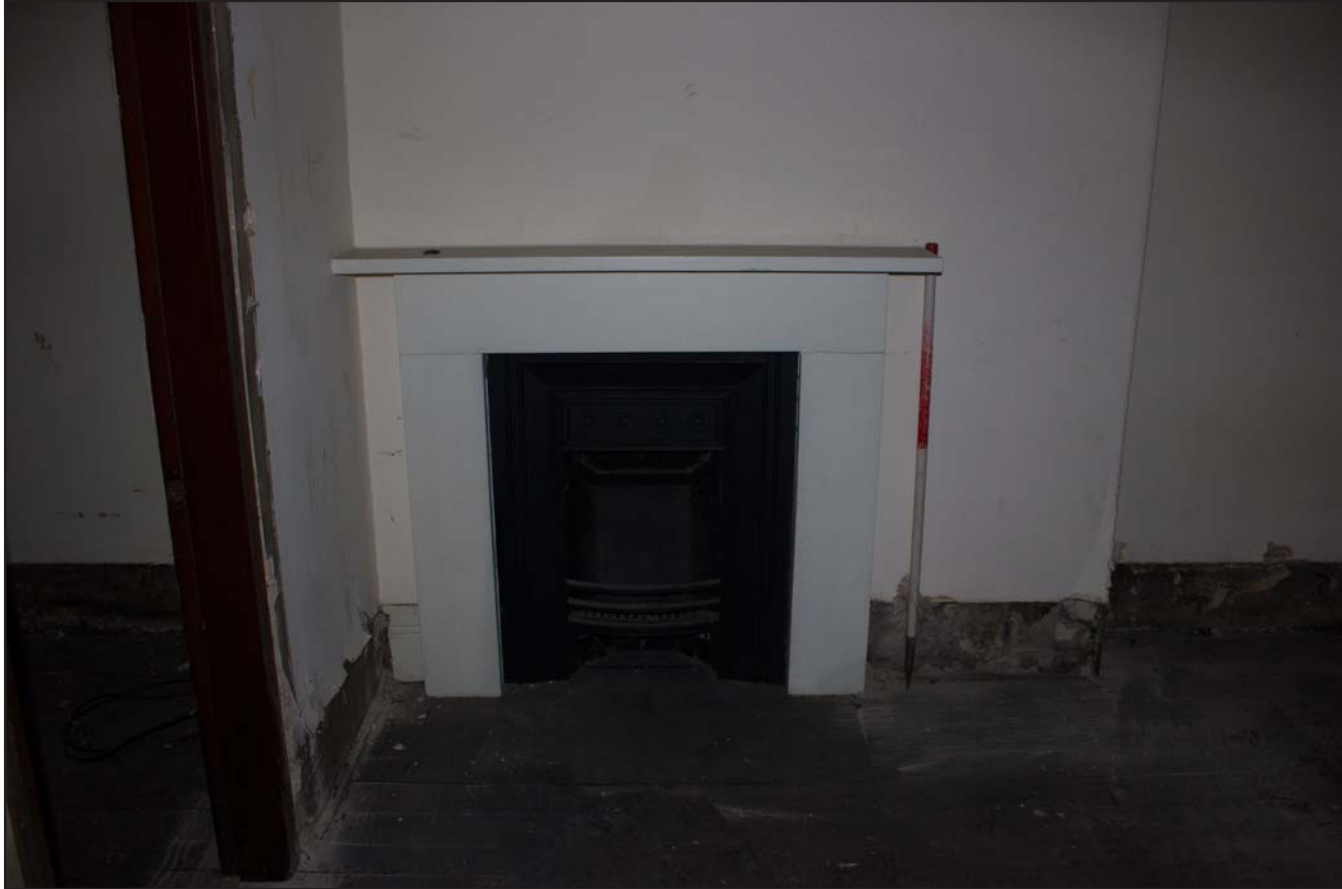
Plate 75: Second Floor Room 4 showing fireplace, from the west. Scale 1.0m.
