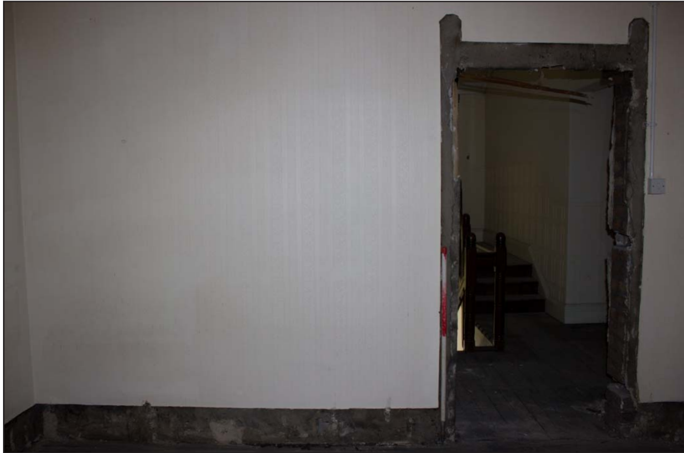
Plate 71: Second Floor Room 3, from the south. Scale 1.0m.
