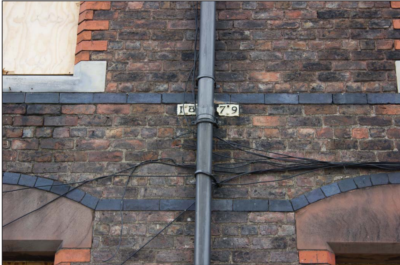
Plate 05: Principle southern external elevation showing date strap, from the south.
