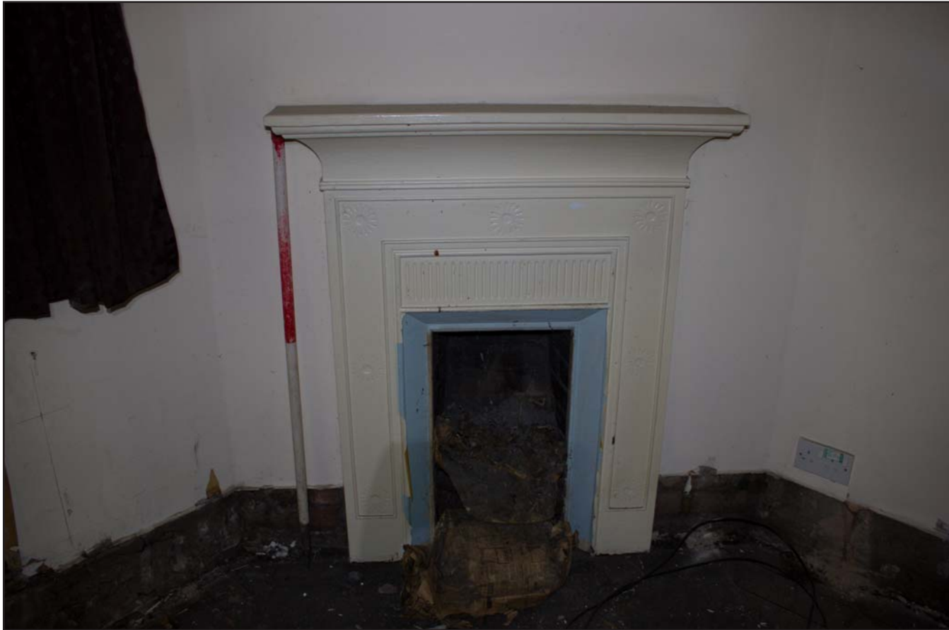
Plate 59: First Floor Store showing fireplace, from the southwest. Scale 1.0m.
