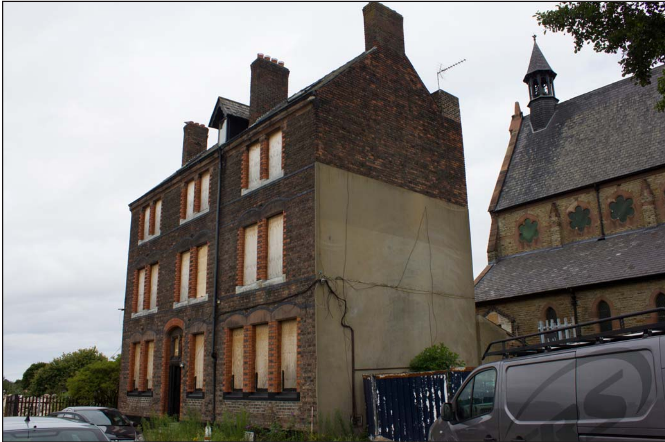
Plate 13: Eastern and southern external elevations, from the southeast. Scale 1.0m.
