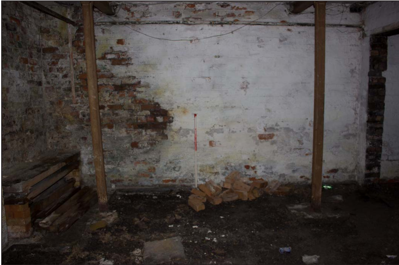
Plate 22: Cellar B5, from the south. Scale 1.0m.
