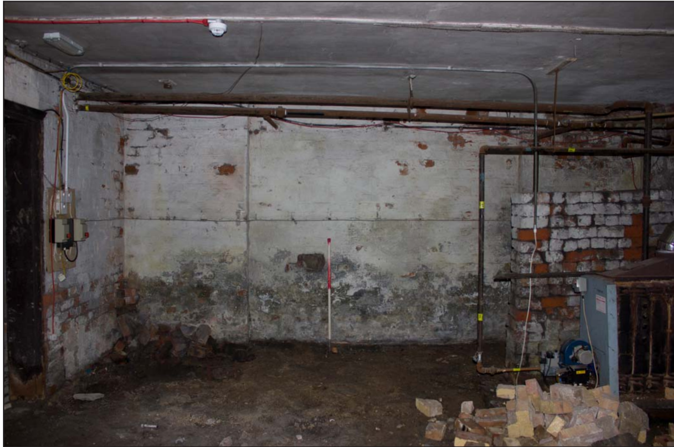
Plate 16: Cellar B2, from the south. Scale 1.0m.
