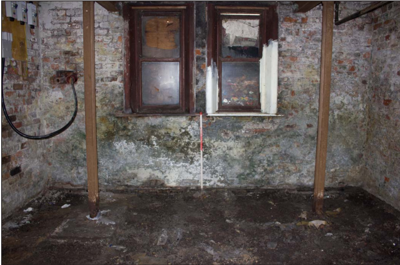
Plate 21: Cellar B5, from the north. Scale 1.0m.
