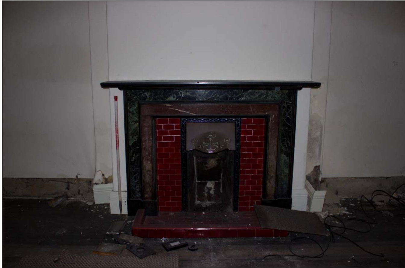
Plate 36: Ground floor Office 2 showing fireplace, from the west. Scale 1.0m.
