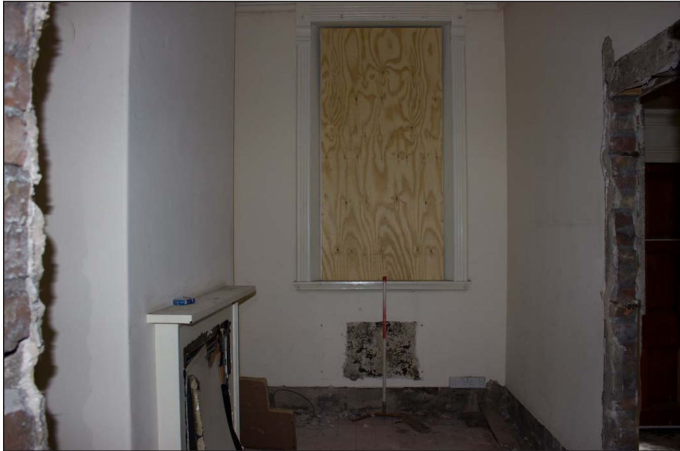
Plate 26: Ground floor Store 1, from the north. Scale 1.0m.
