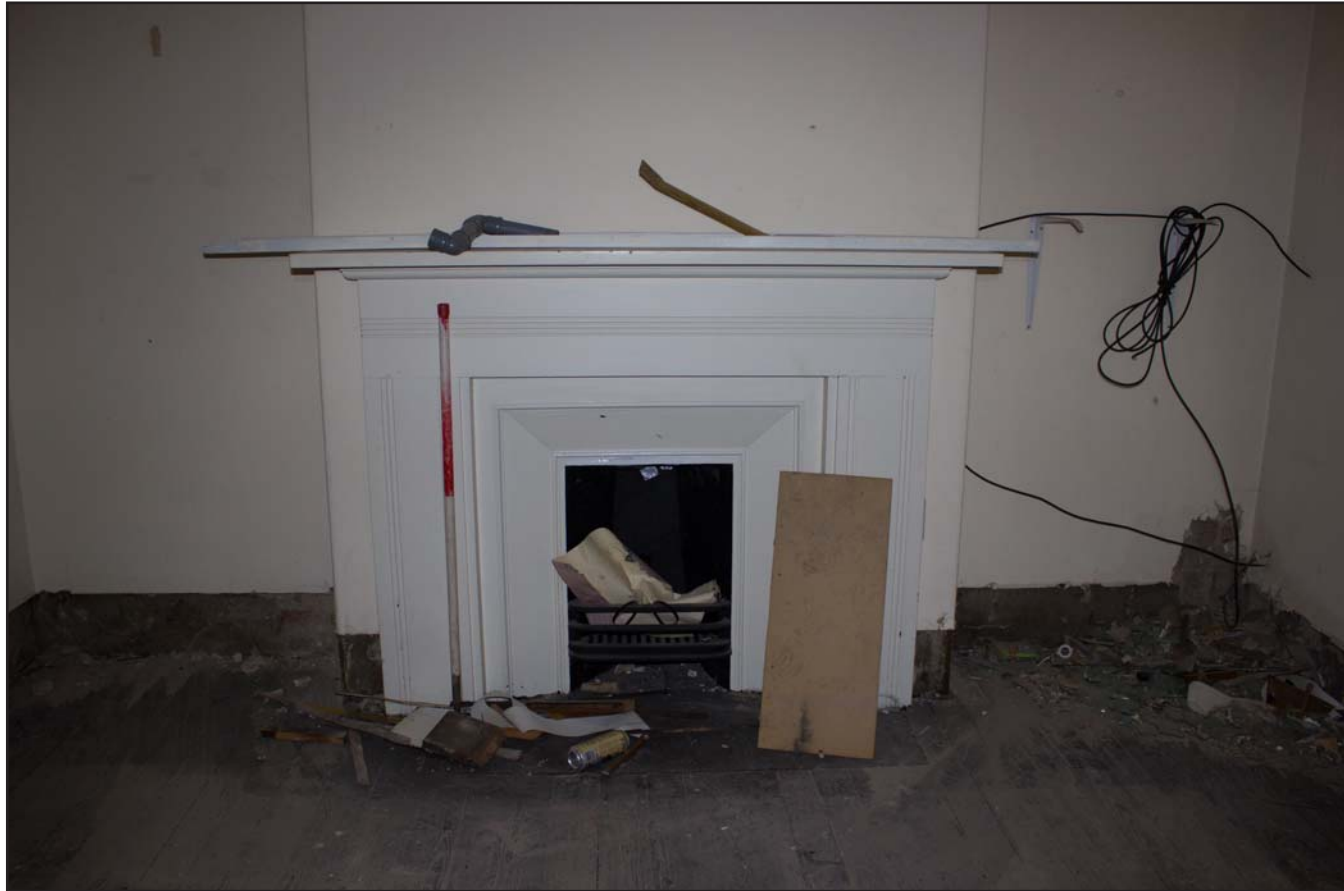
Plate 54: First Floor Room 10 showing fireplace, from the west. Scale 1.0m.
