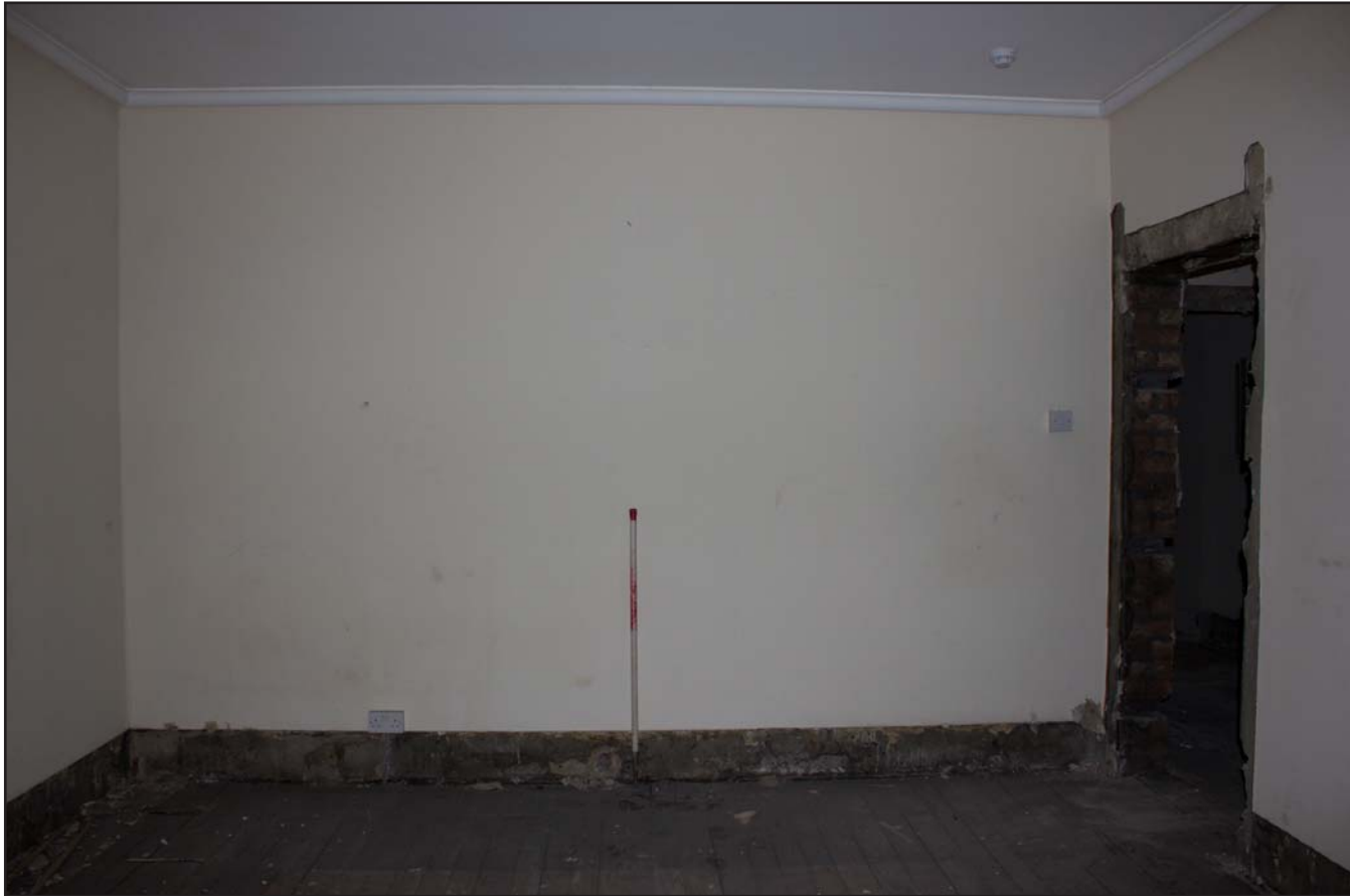
Plate 65: Second Floor Room 1, from the south. Scale 1.0m.
