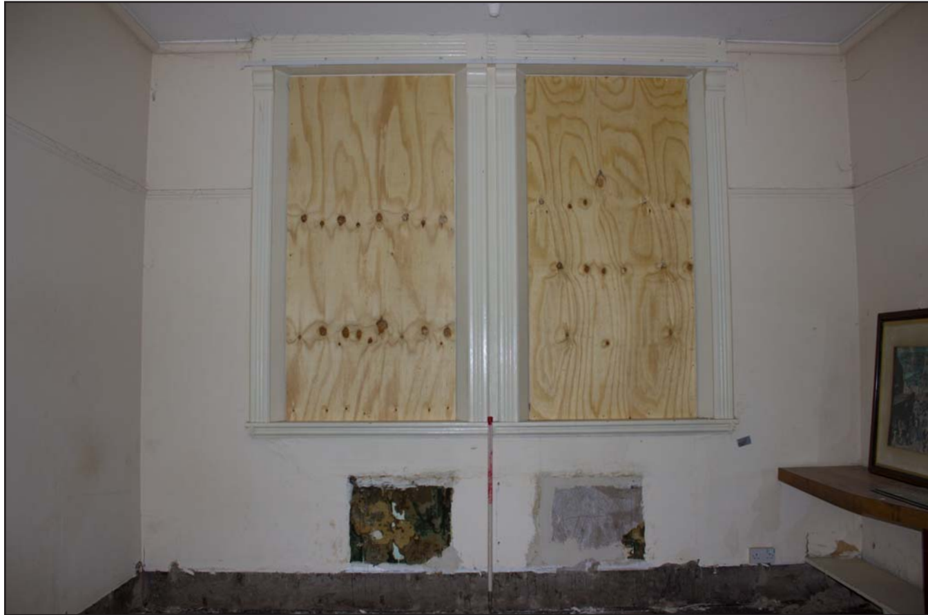
Plate 32: Ground floor Office 1, from the north. Scale 1.0m.
