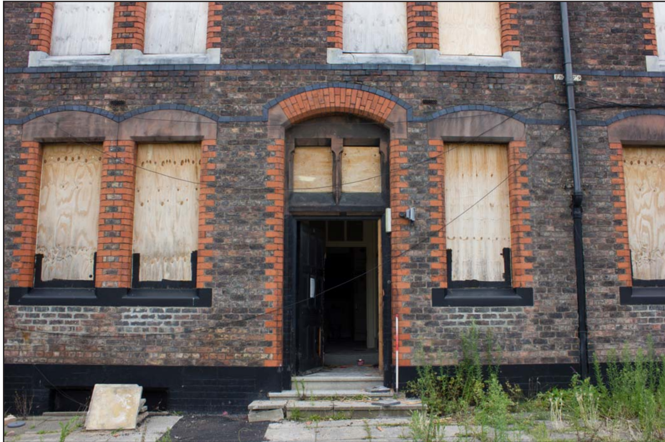
Plate 04: Southern principle external elevation showing ground floor entrance, from the south. Scale 1.0m.
