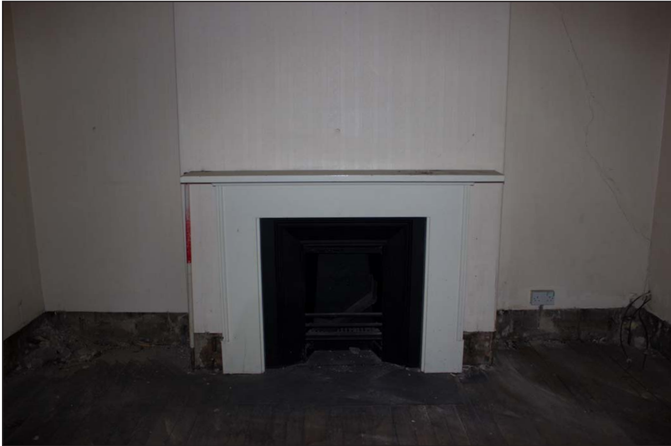
Plate 72: Second Floor Room 3 showing fireplace, from the west. Scale 1.0m.
