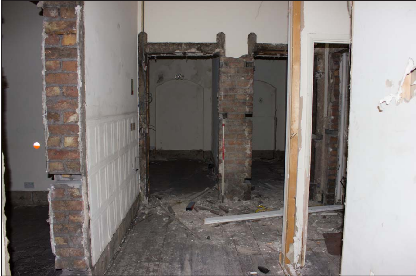
Plate 44: First Floor Landing, from the east. Scale 1.0m.
