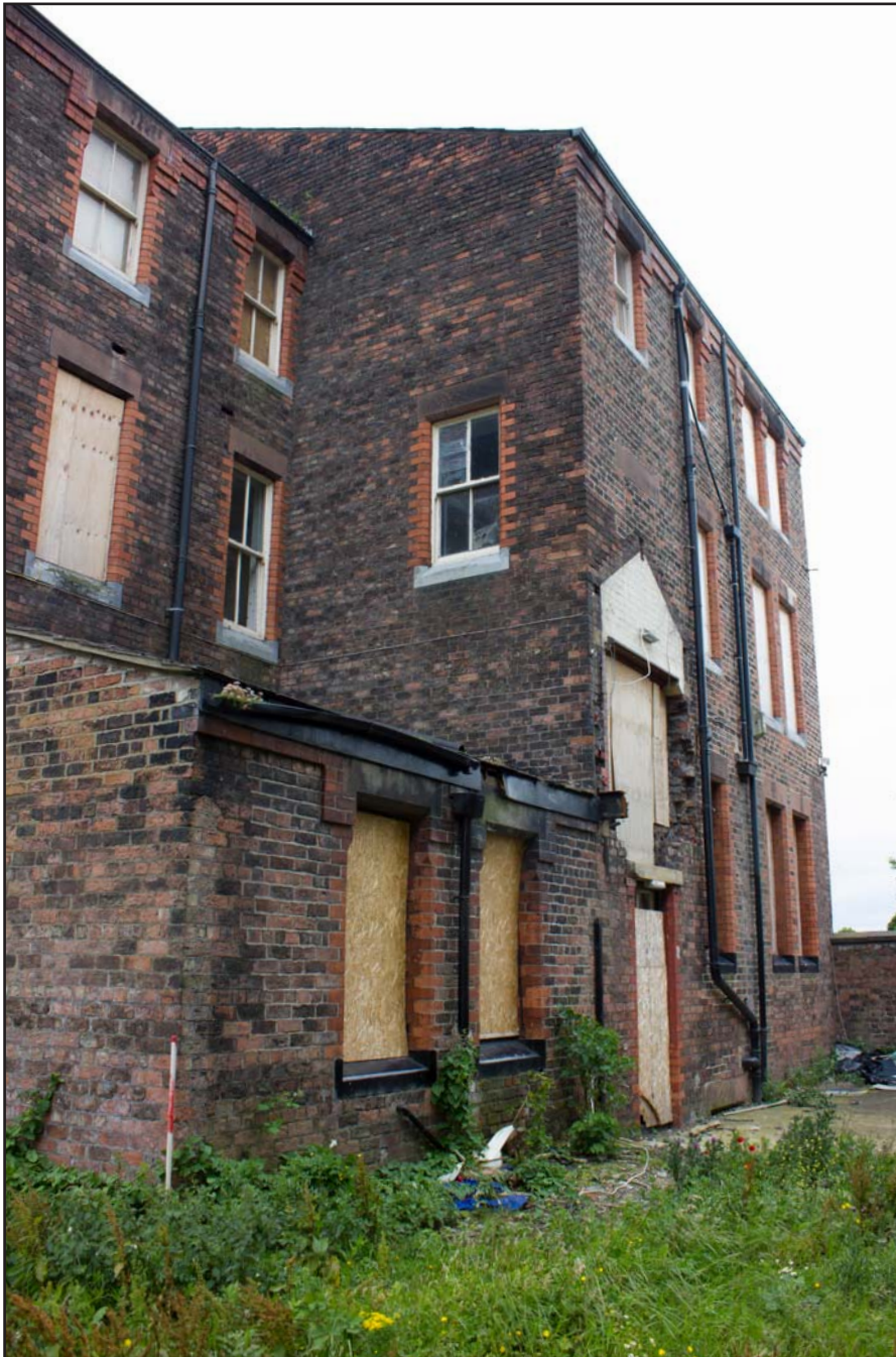
Plate 10: Northern external elevation, from the north-northeast. Scale 1.0m.
