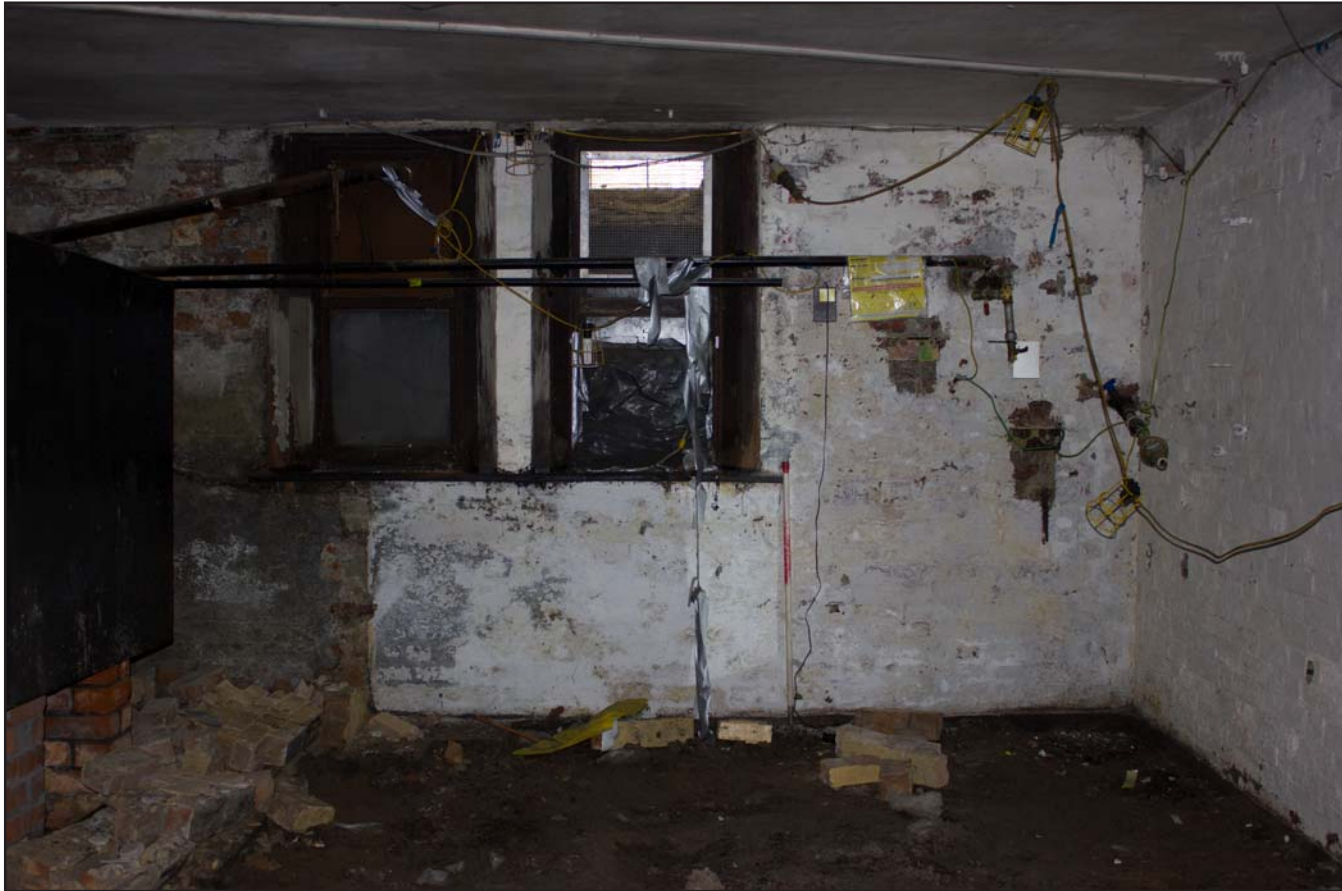
Plate 15: Cellar B2, from the north. Scale 1.0m.
