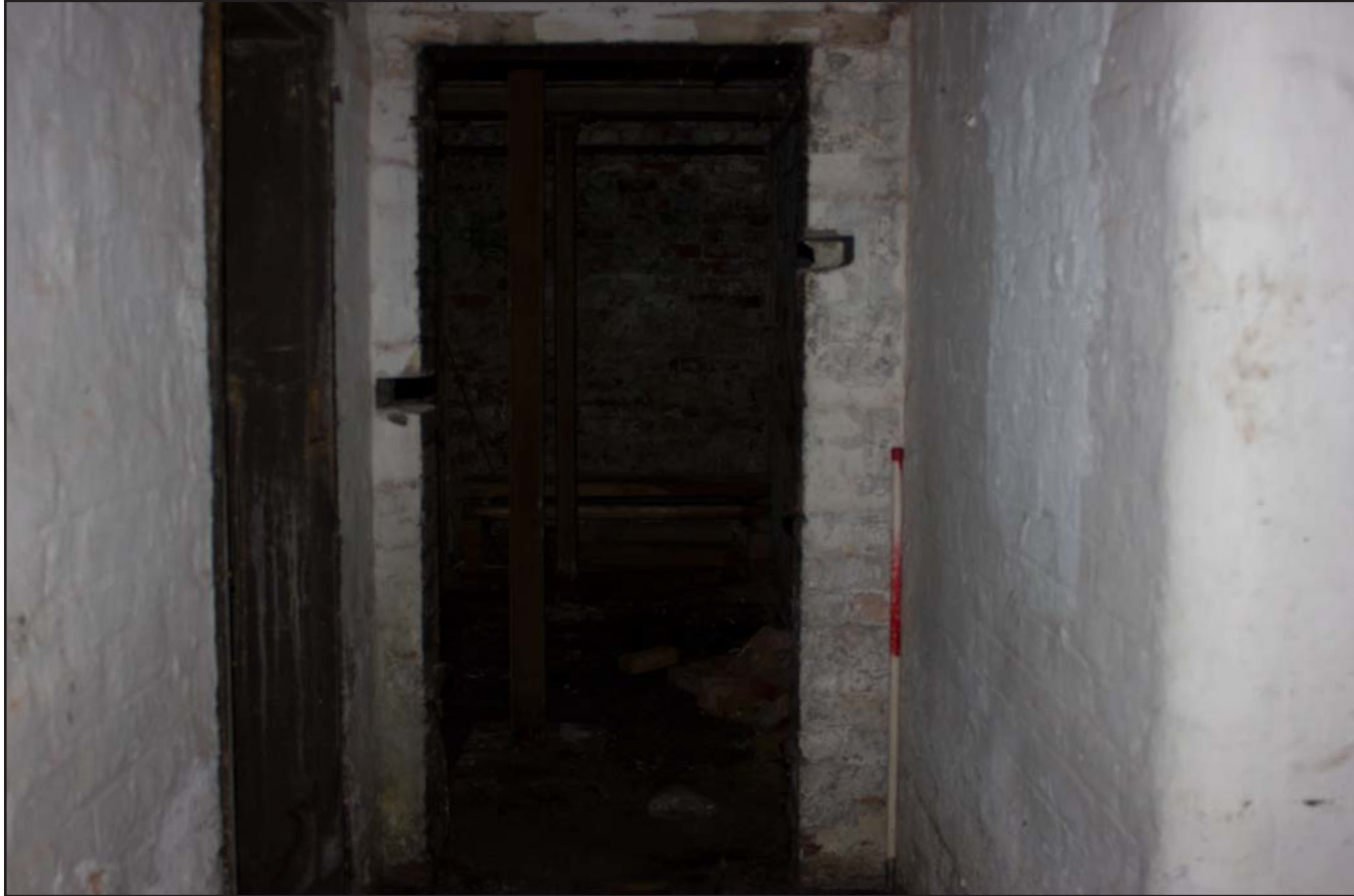
Plate 14: Cellar B1, from the east. Scale 1.0m.
