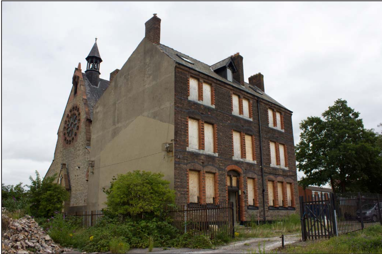
Plate 06: Southern and western external elevations, from the southwest. Scale 1.0m.
