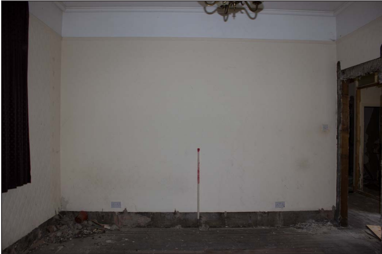
Plate 56: First Floor Room 11, from the east. Scale 1.0m.
