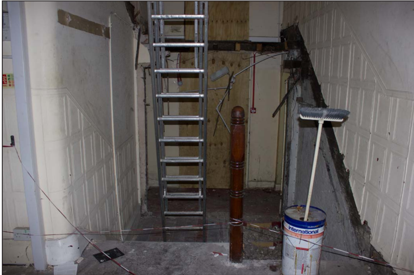
Plate 31: Ground floor Stairwell, from the south.
