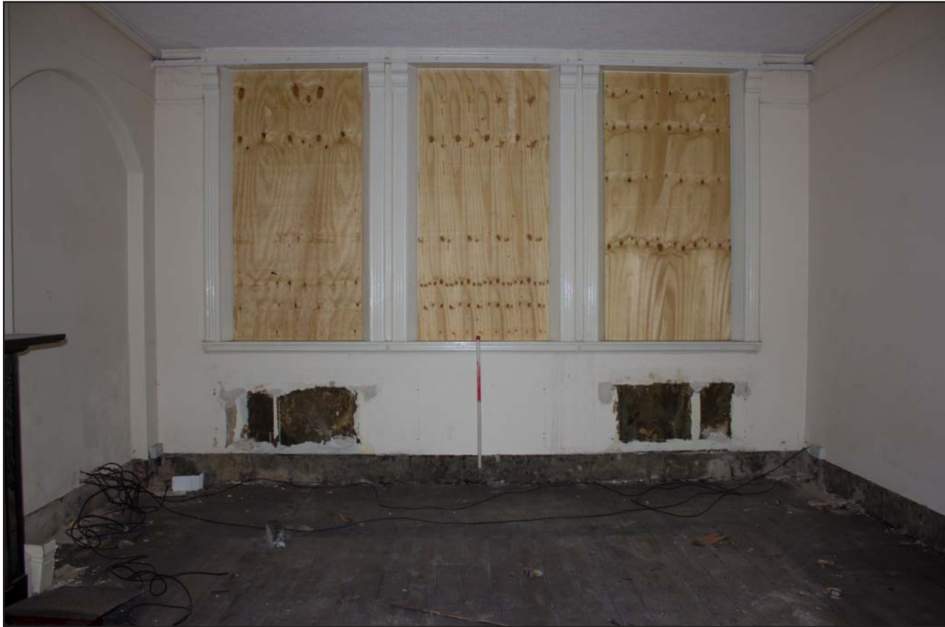
Plate 34: Ground floor Office 2, from the north. Scale 1.0m.
