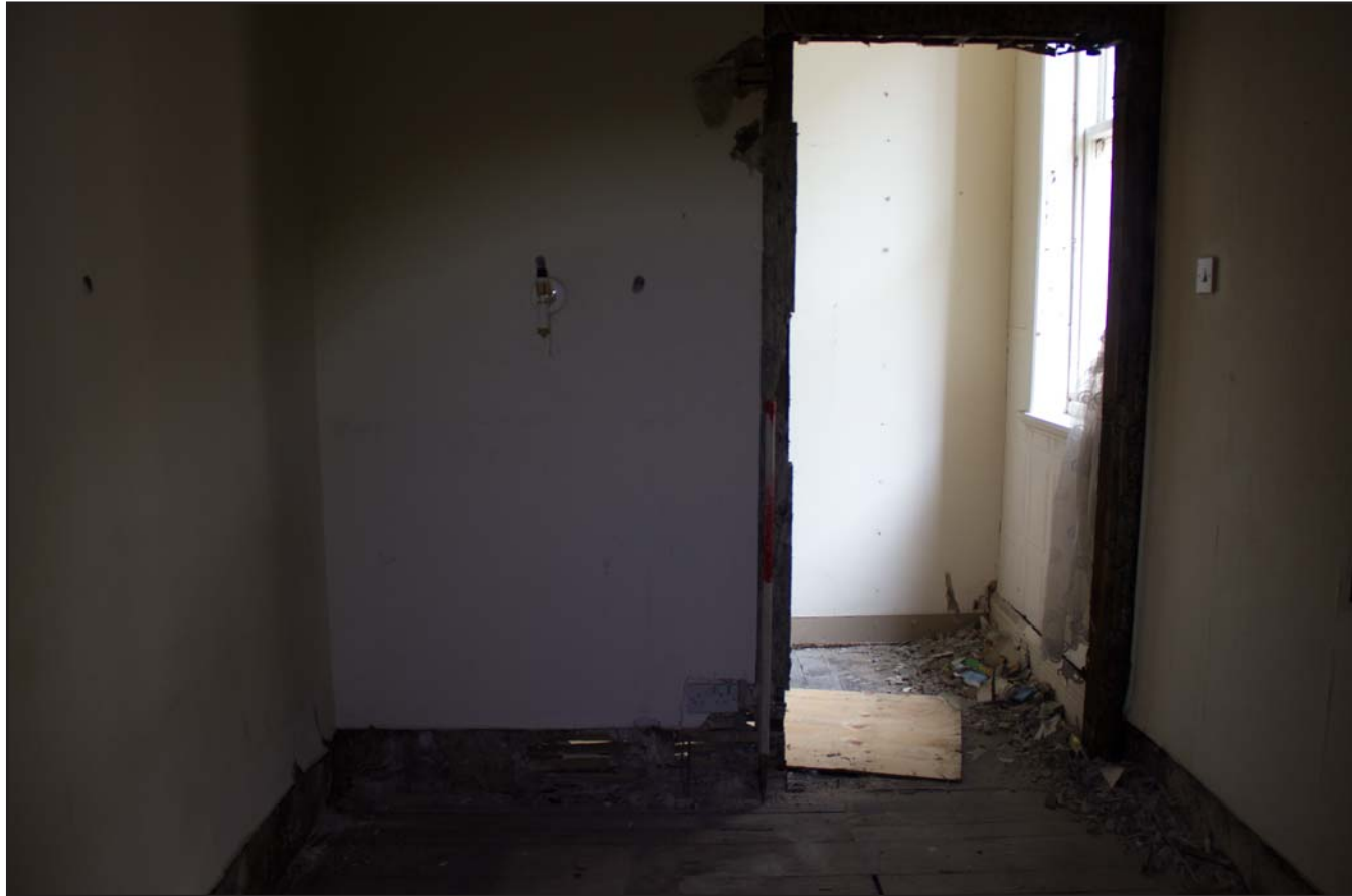
Plate 58: First Floor Store, from the east. Scale 1.0m.
