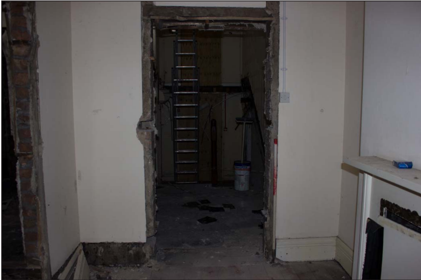
Plate 27: Ground floor Store 1, from the south. Scale 1.0m.
