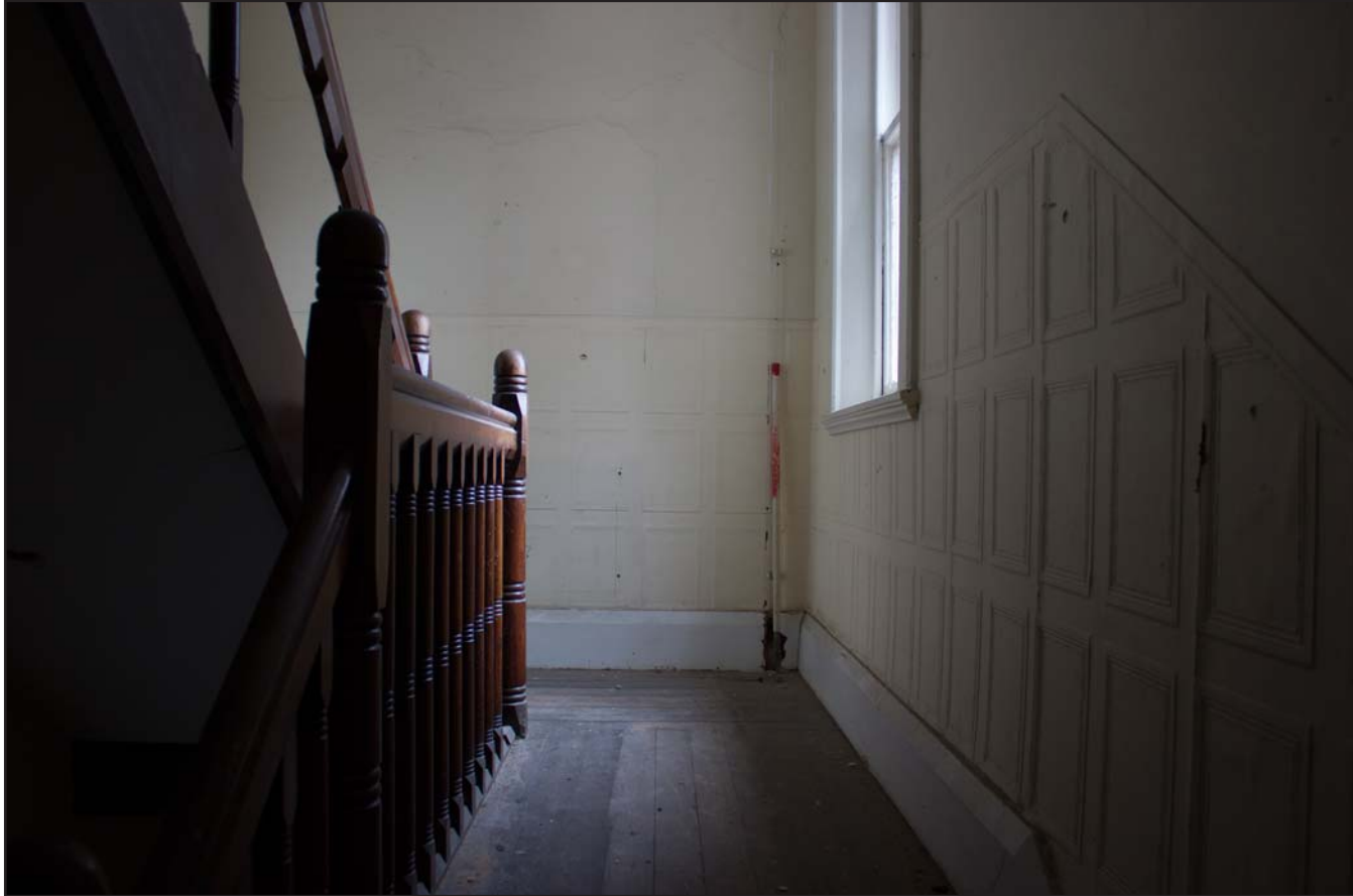
Plate 46: First Floor Stairwell, from the south. Scale 1.0m.
