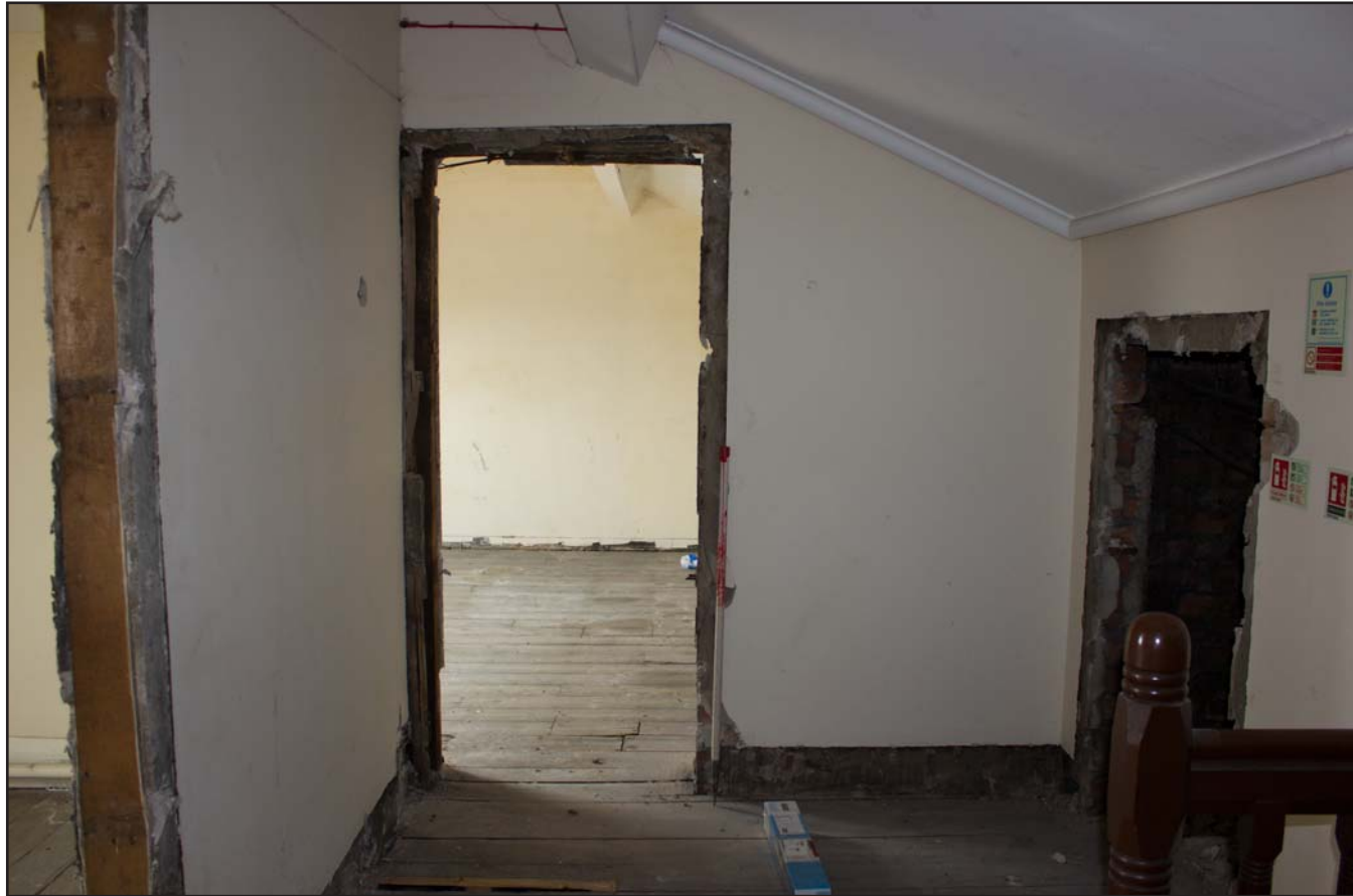
Plate 80: Third Floor Landing, from the east. Scale 1.0m.
