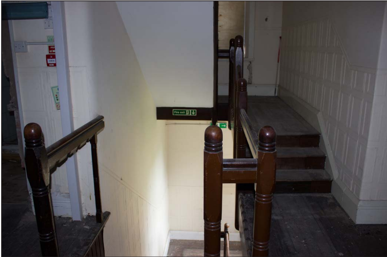
Plate 63: Second Floor Stairwell, from the south. Scale 1.0m.
