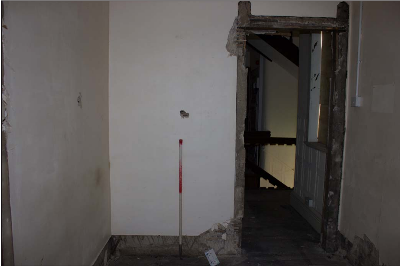
Plate 77: Second Floor Store, from the east. Scale 1.0m.
