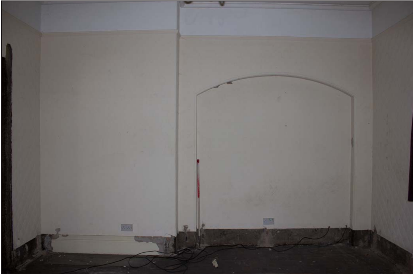
Plate 55: First Floor Room 11, from the west. Scale 1.0m.
