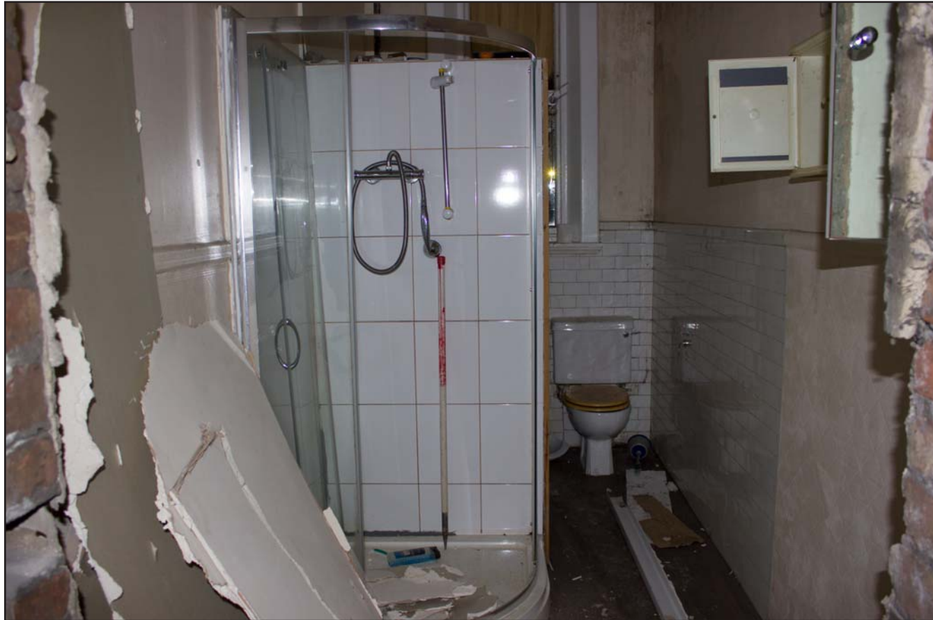
Plate 60: First Floor WC, from the south. Scale 1.0m.
