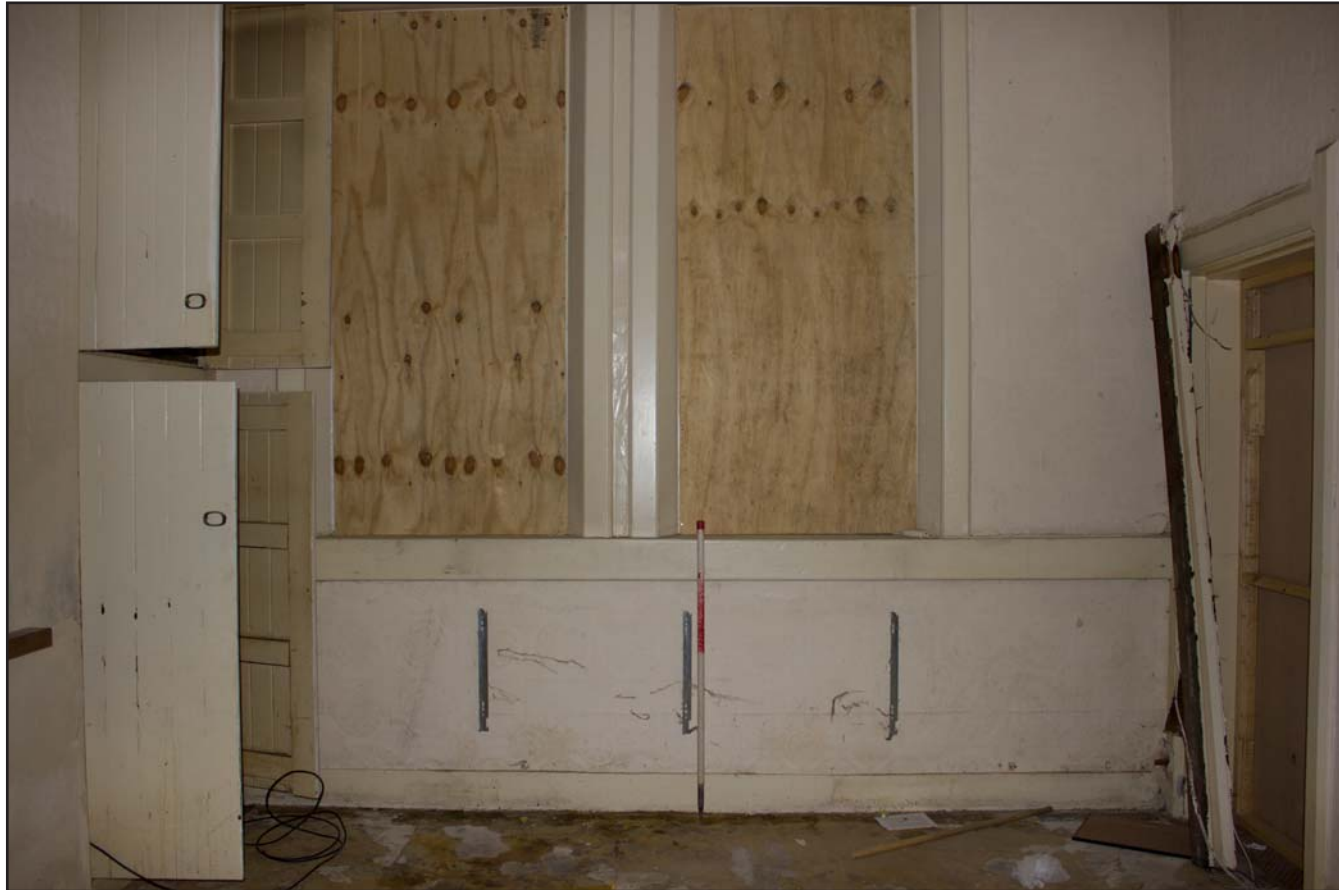
Plate 38: Ground floor Store 2, from the south. Scale 1.0m.
