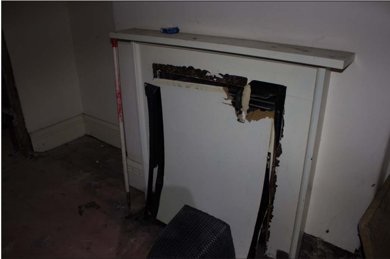
Plate 28: Ground floor Store 1 showing fireplace, from the southwest. Scale 1.0m.
