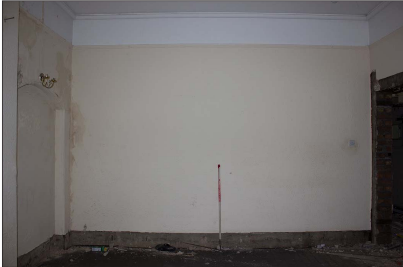
Plate 48: First Floor Room 8, from the south. Scale 1.0m.
