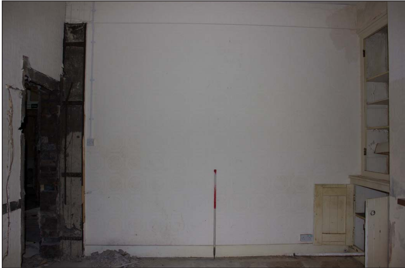
Plate 39: Ground floor Store 2, from the north. Scale 1.0m.
