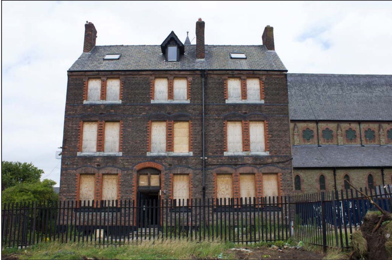
Plate 01: Southern principle external elevation, from the south. Scale 1.0m.
