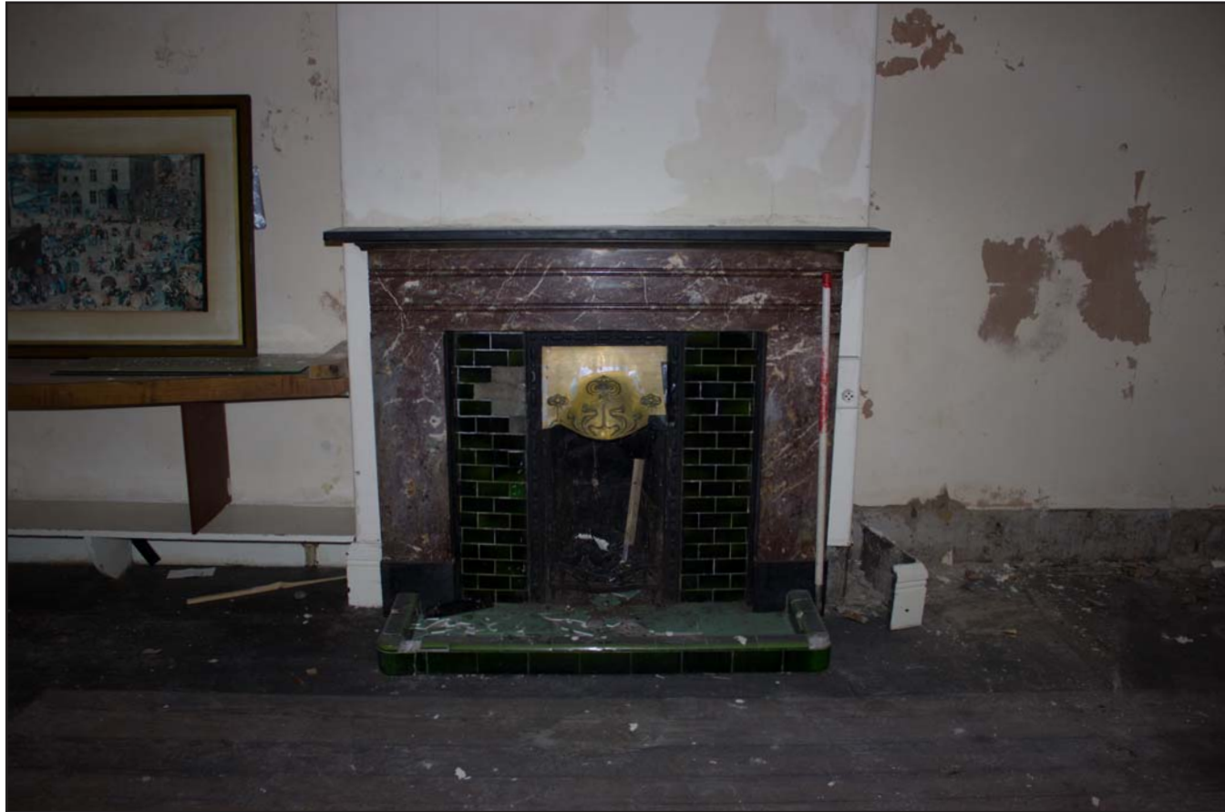
Plate 33: Ground floor Office 1 showing fireplace, from the east. Scale 1.0m.
