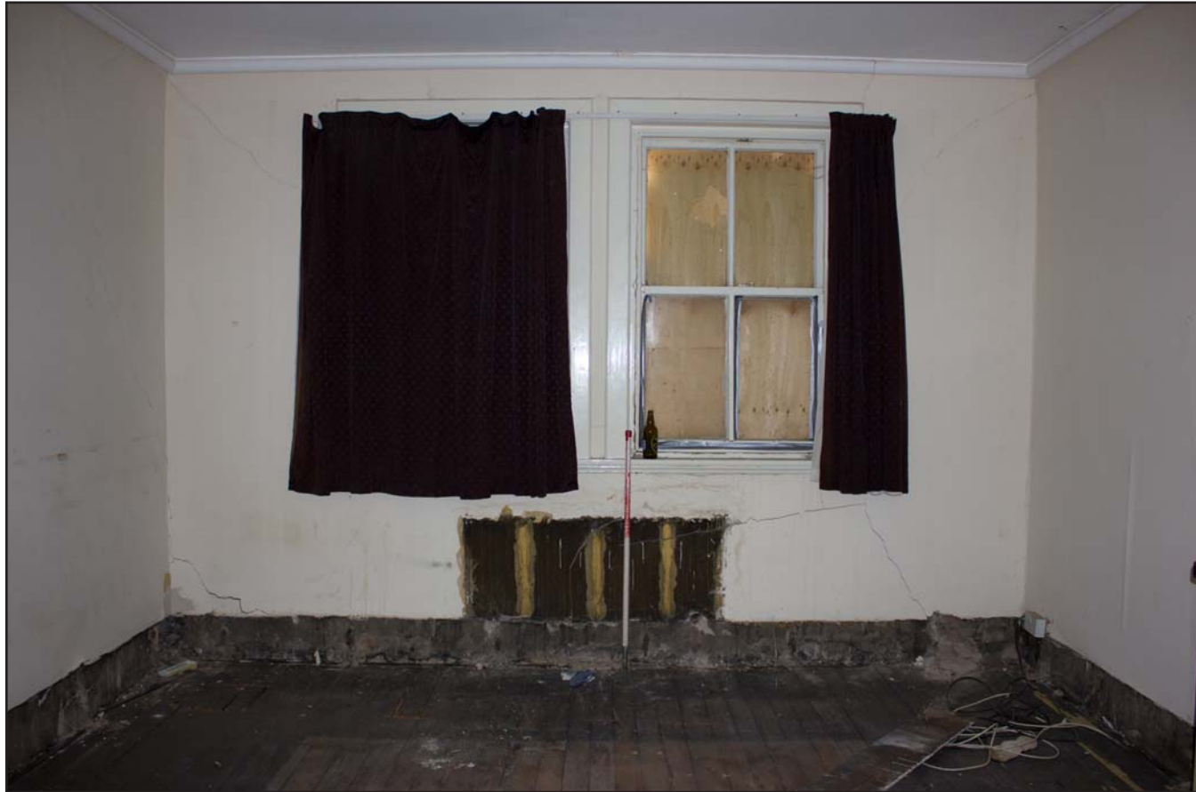
Plate 64: Second Floor Room 1, from the north. Scale 1.0m.
