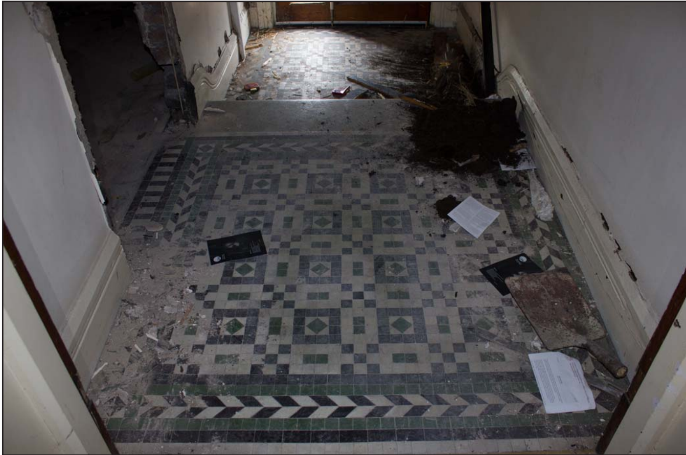
Plate 25: Ground floor Hallway showing tiled floor, from the north.
