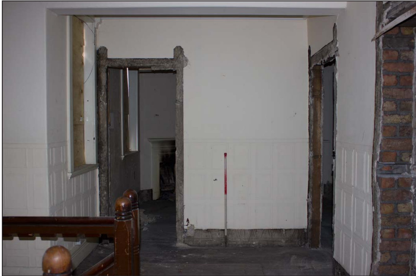
Plate 62: Second Floor Landing, from the west. Scale 1.0m.
