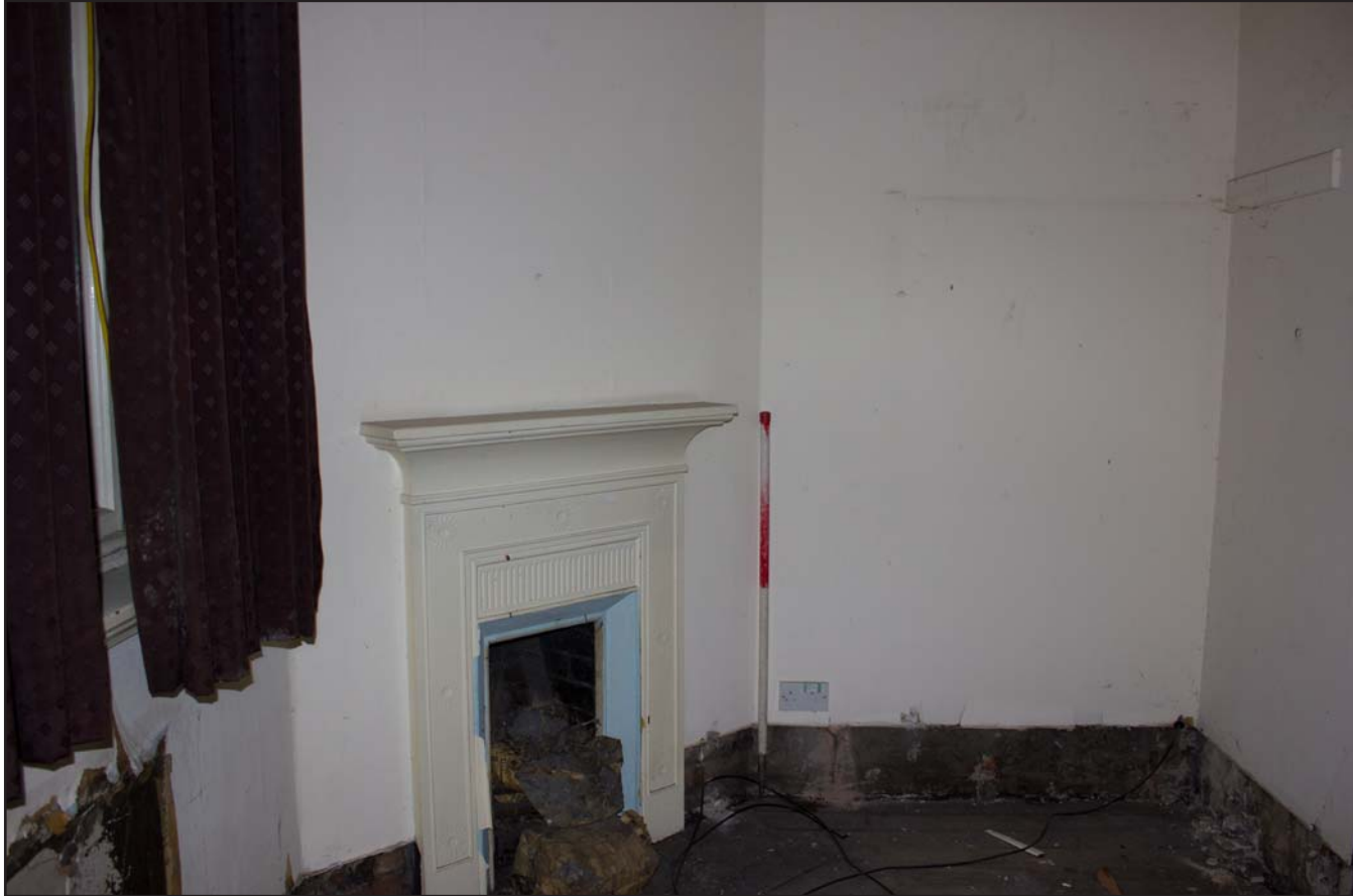
Plate 57: First Floor Store, from the west. Scale 1.0m.
