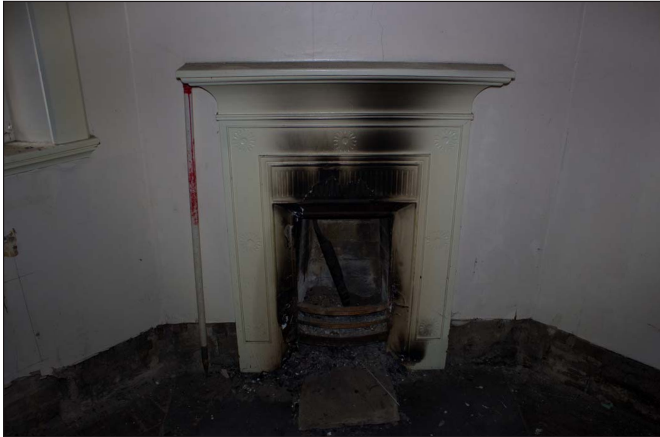
Plate 78: Second Floor Store showing fireplace, from the southwest. Scale 1.0m.
