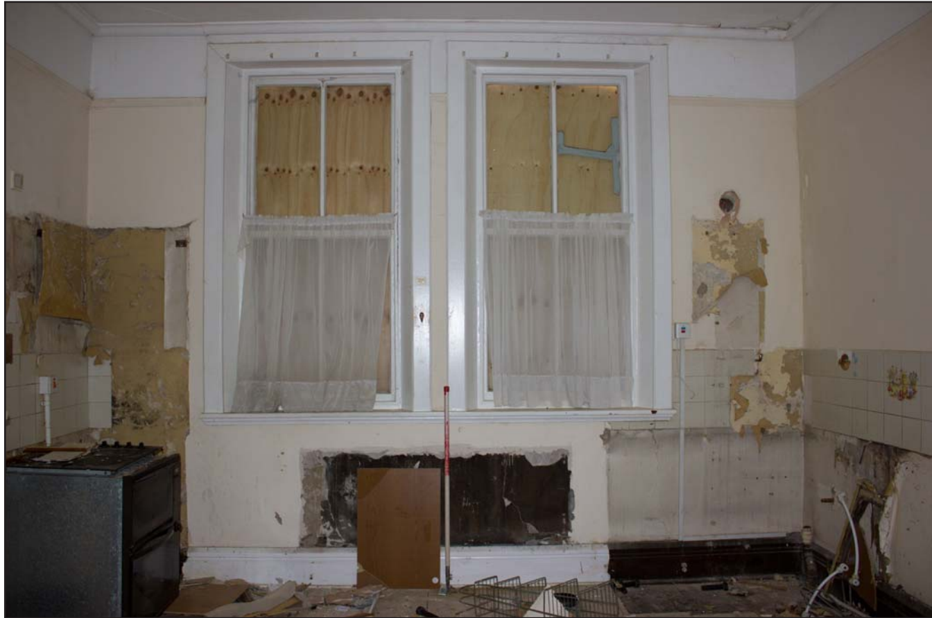
Plate 49: First Floor Room 9, from the south. Scale 1.0m.
