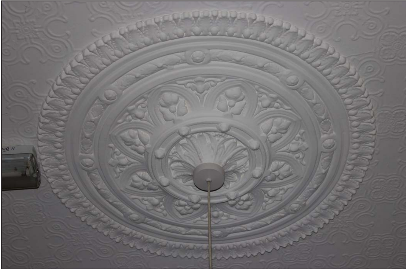
Plate 37: Ground floor Office 2 showing plaster ceiling rose, from the west.
