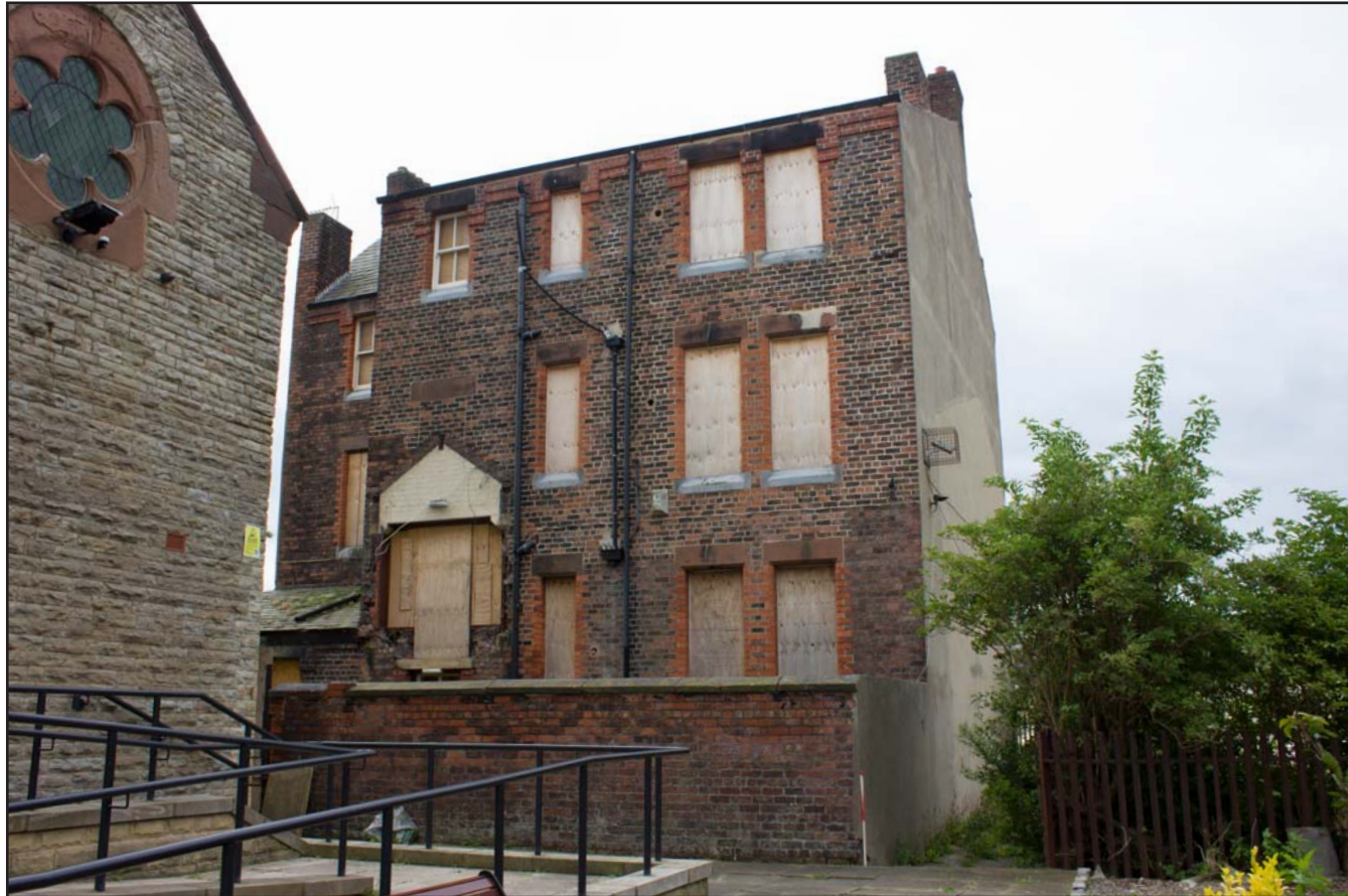
Plate 09: Northern external elevation, from the north-northwest. Scale 1.0m.
