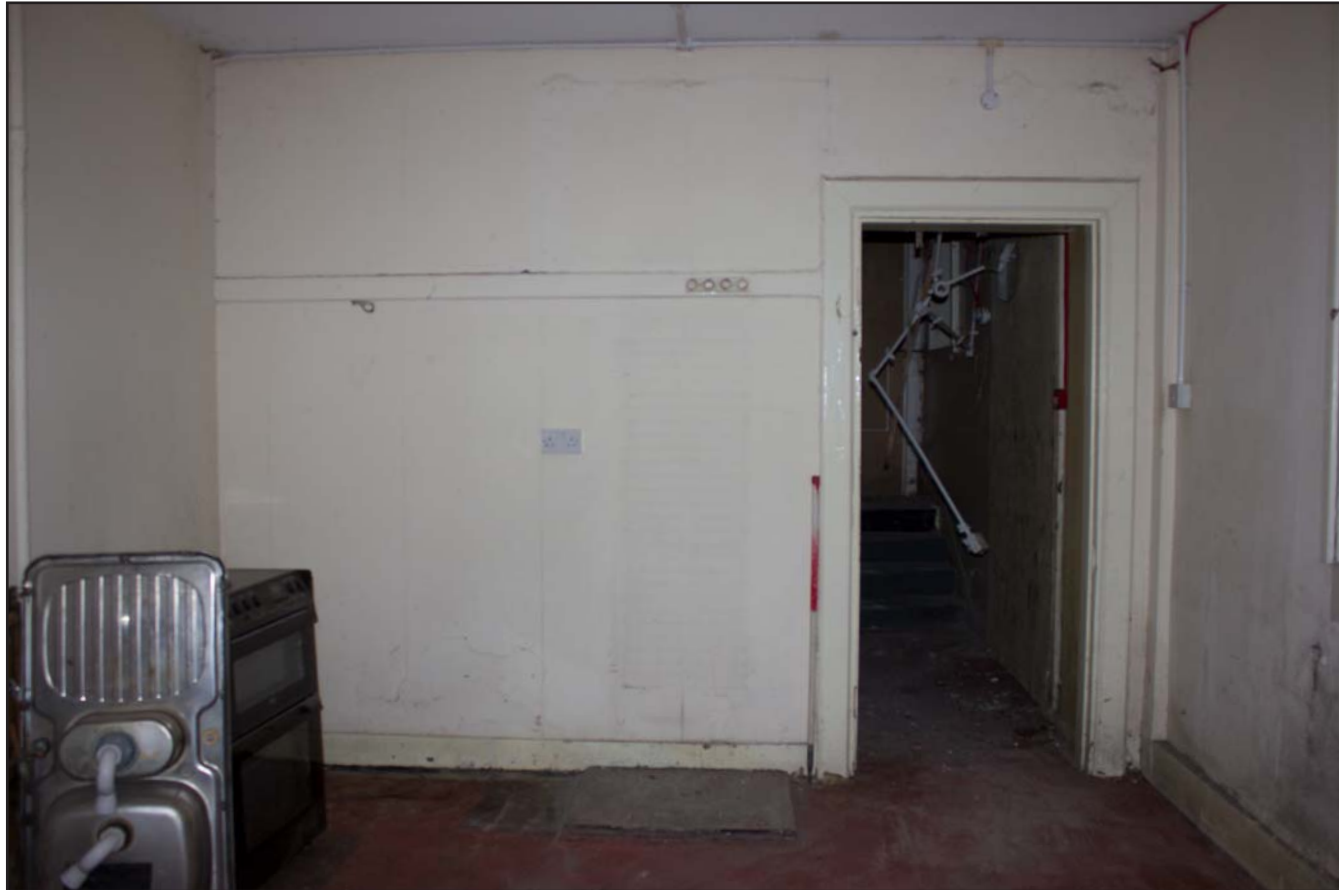
Plate 43: Ground floor Kitchen, from the east. Scale 1.0m.
