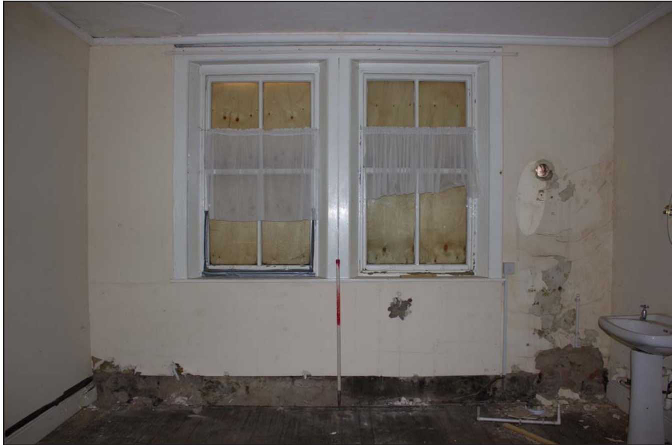
Plate 67: Second Floor Room 2, from the south. Scale 1.0m.
