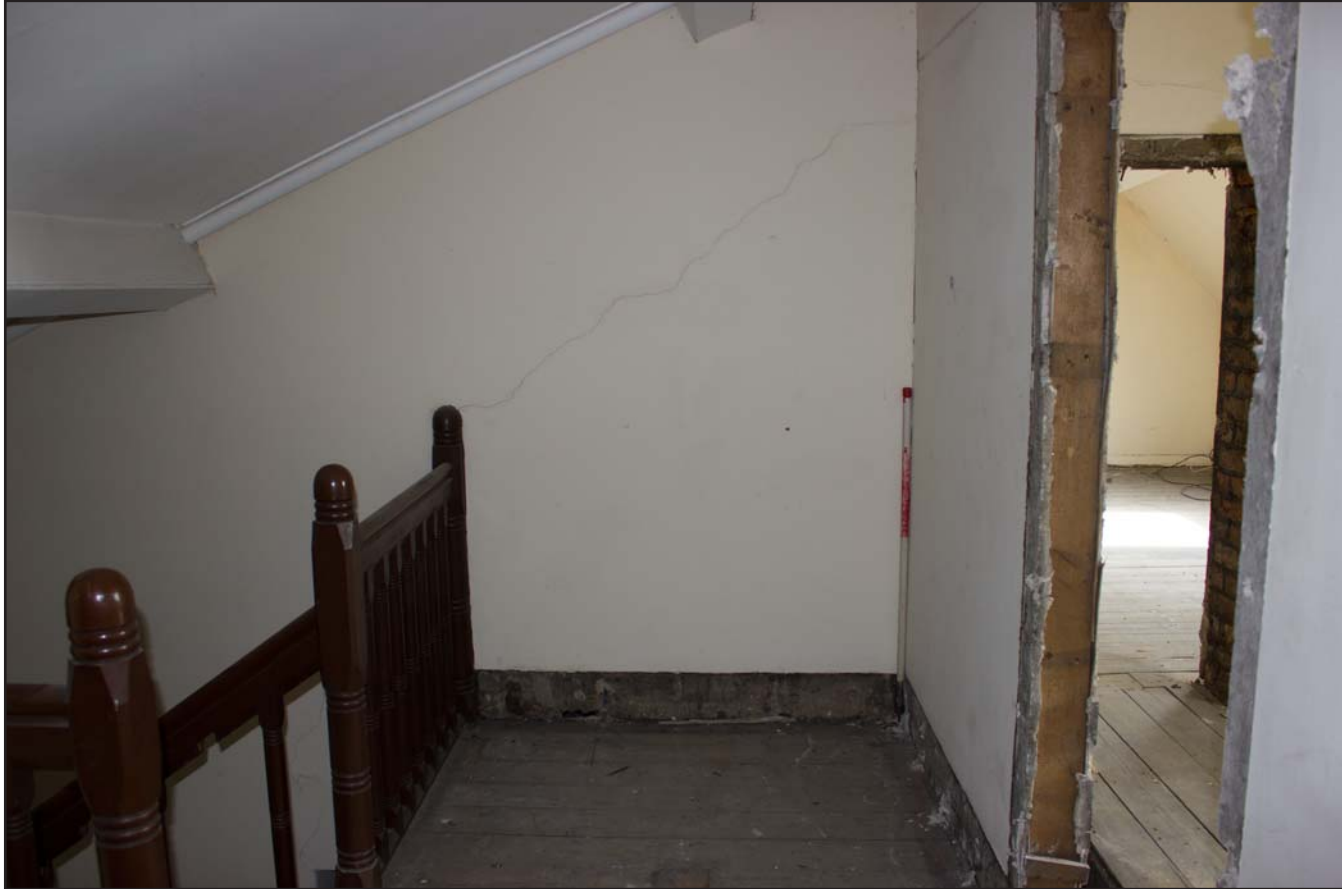
Plate 81: Third Floor Landing, from the west. Scale 1.0m.
