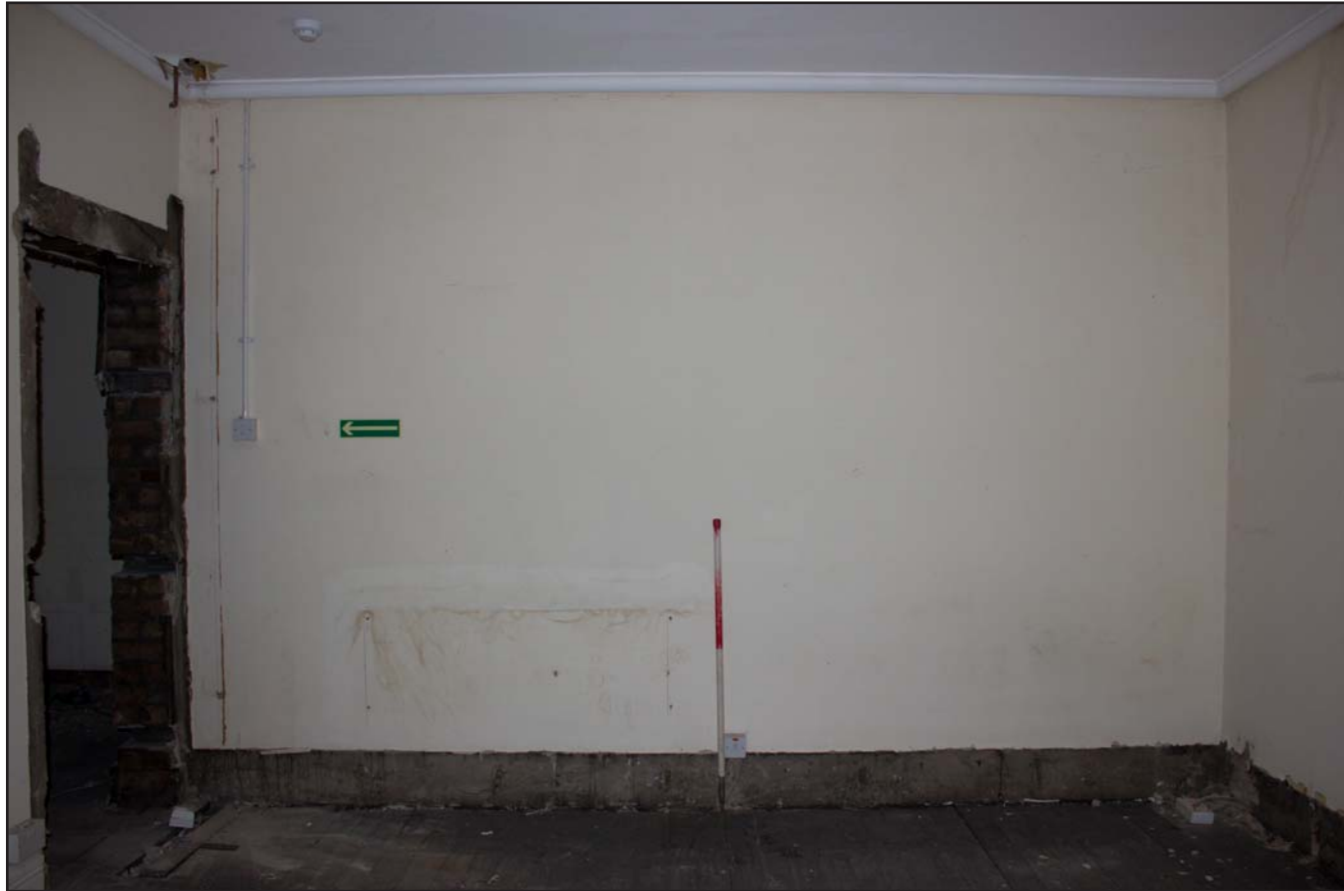
Plate 68: Second Floor Room 2, from the north. Scale 1.0m.
