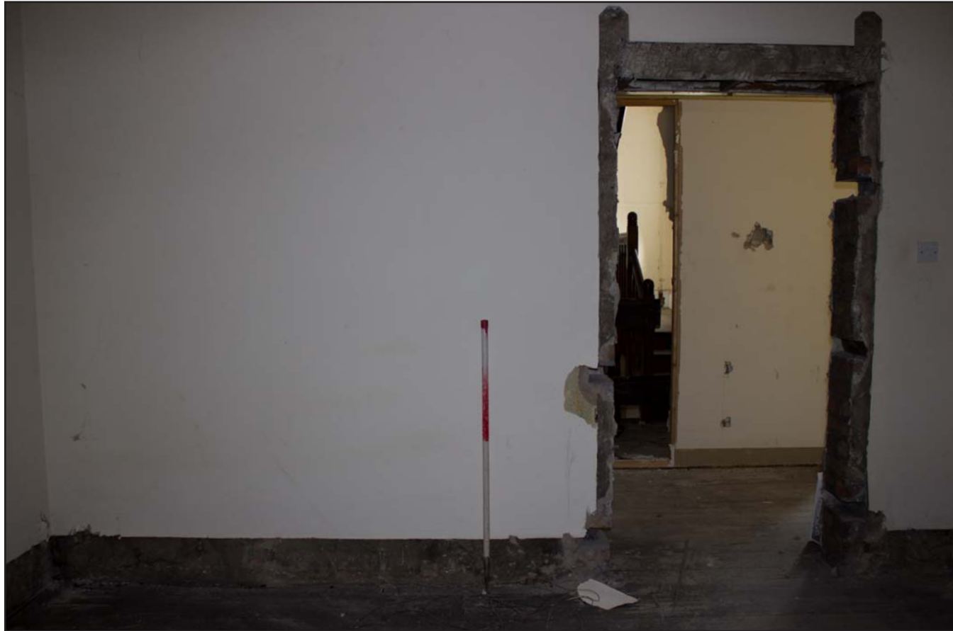
Plate 53: First Floor Room 10, from the south. Scale 1.0m.
