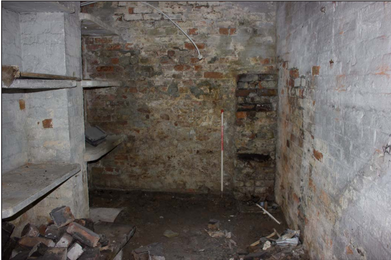
Plate 18: Cellar B3, from the north. Scale 1.0m.
