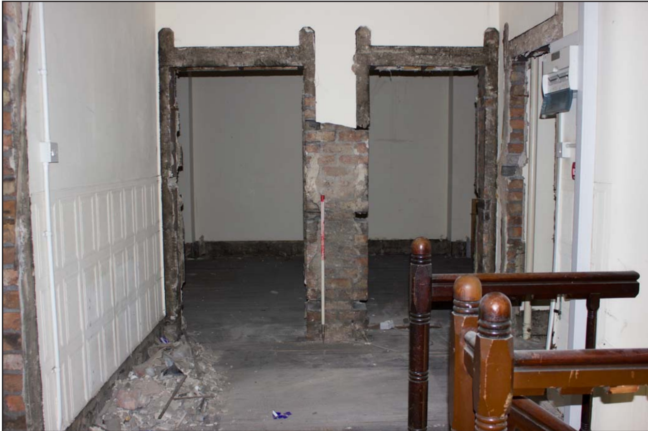
Plate 61: Second Floor Landing, from the east. Scale 1.0m.
