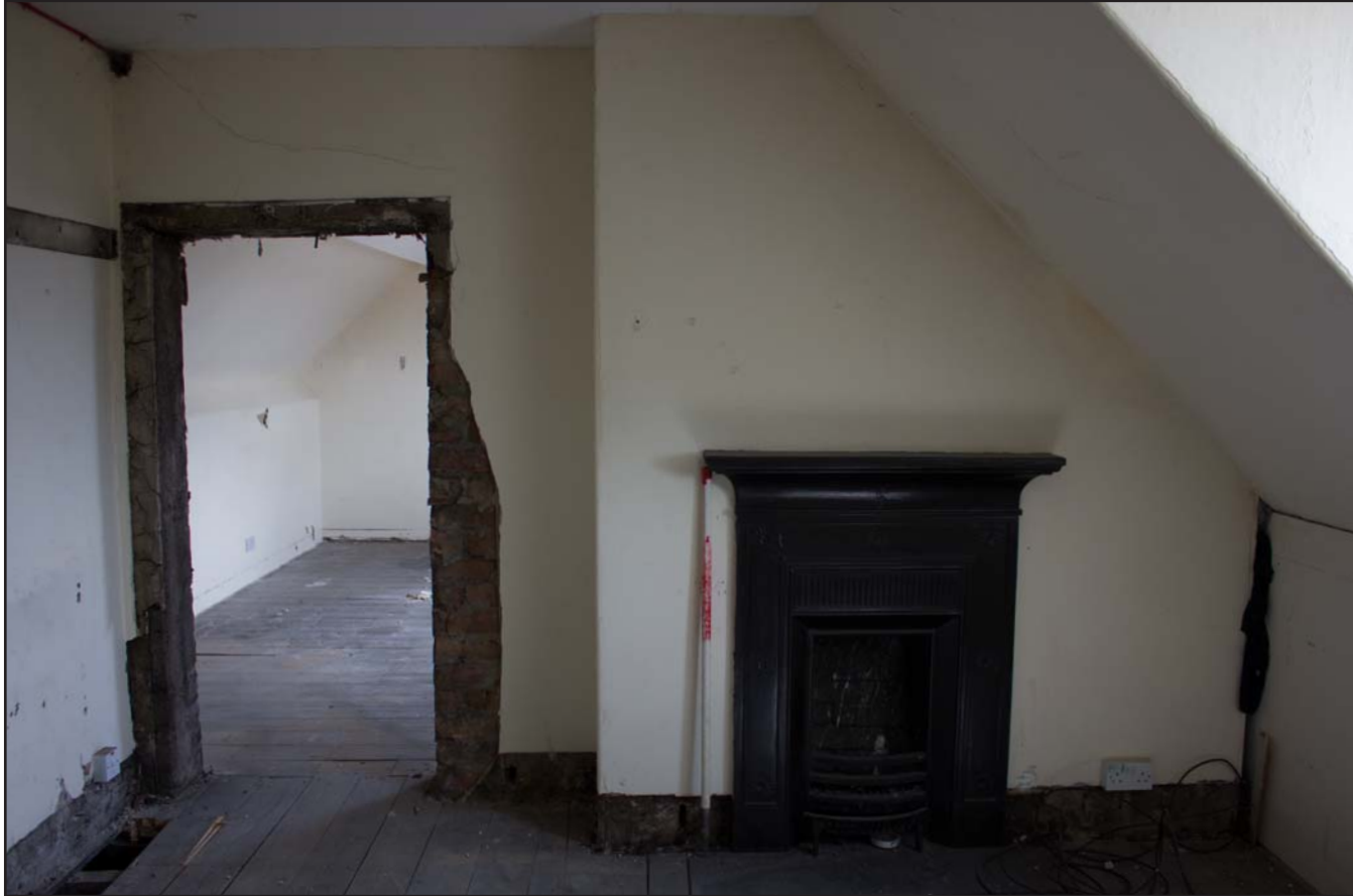
Plate 84: Third Floor Room 6 showing fireplace, from the west. Scale 1.0m.
