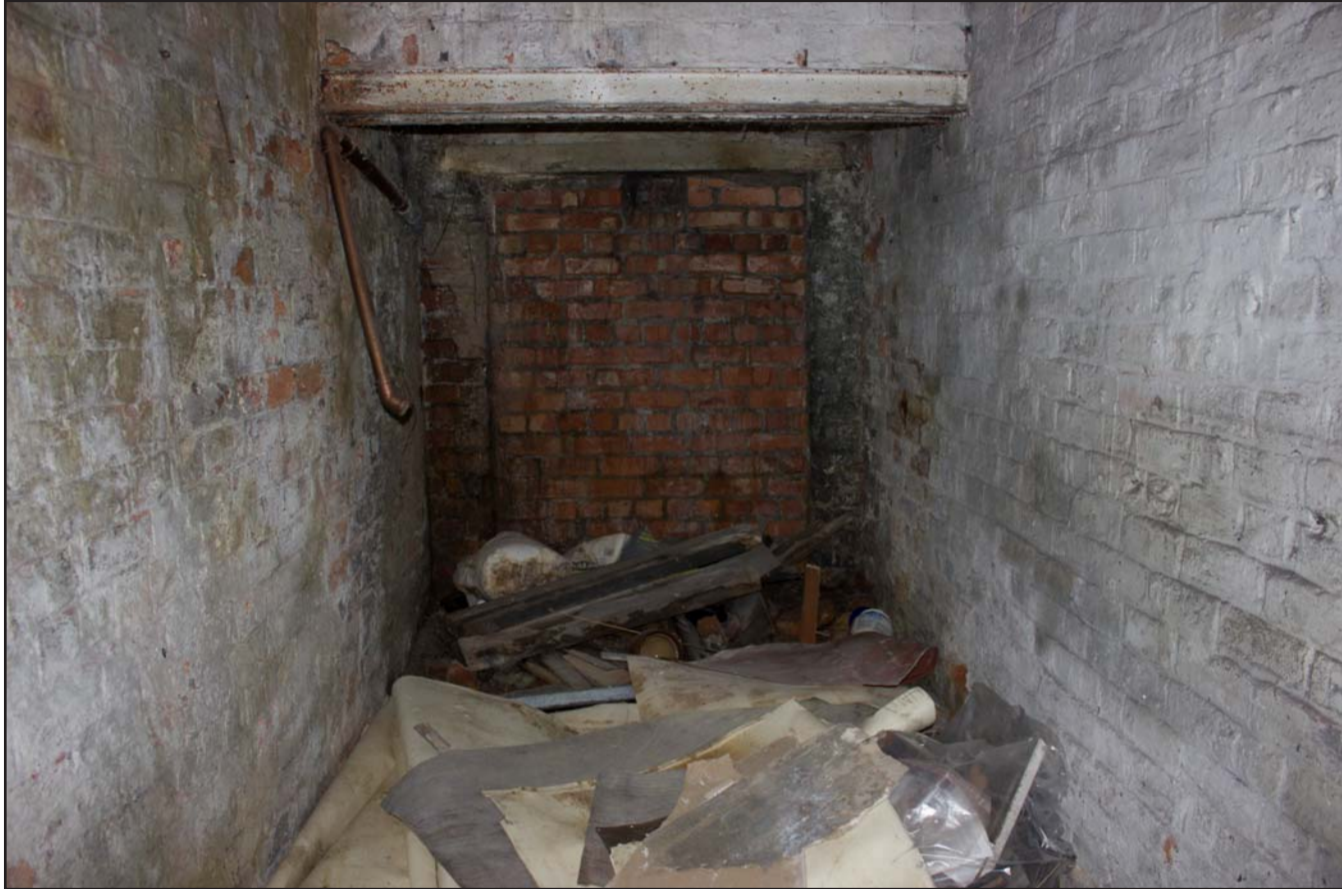
Plate 23: Cellar B6, from the south.
