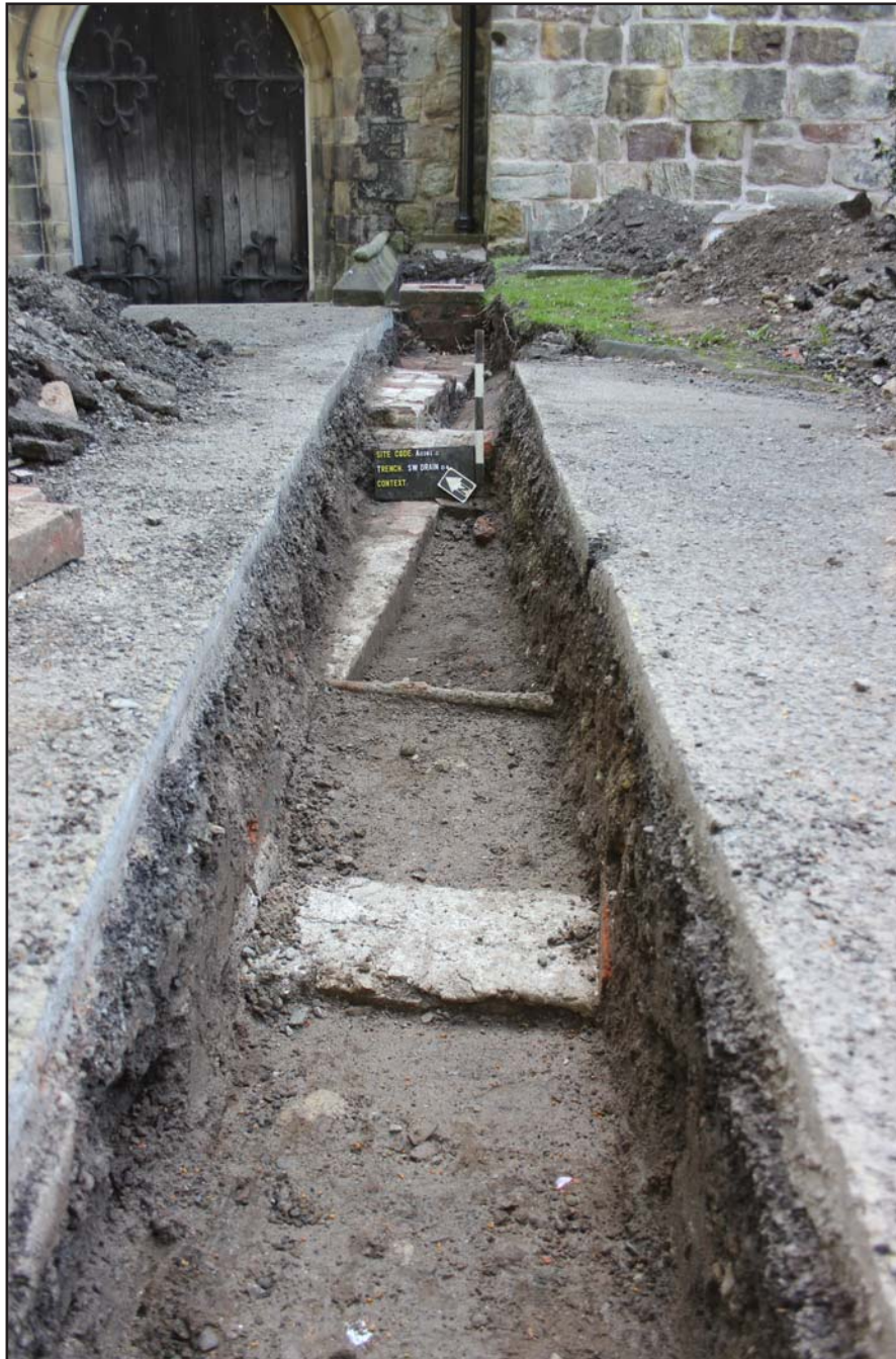
Plate 19: Excavated trench for Drain 4 - from the southwest - scale 2m
