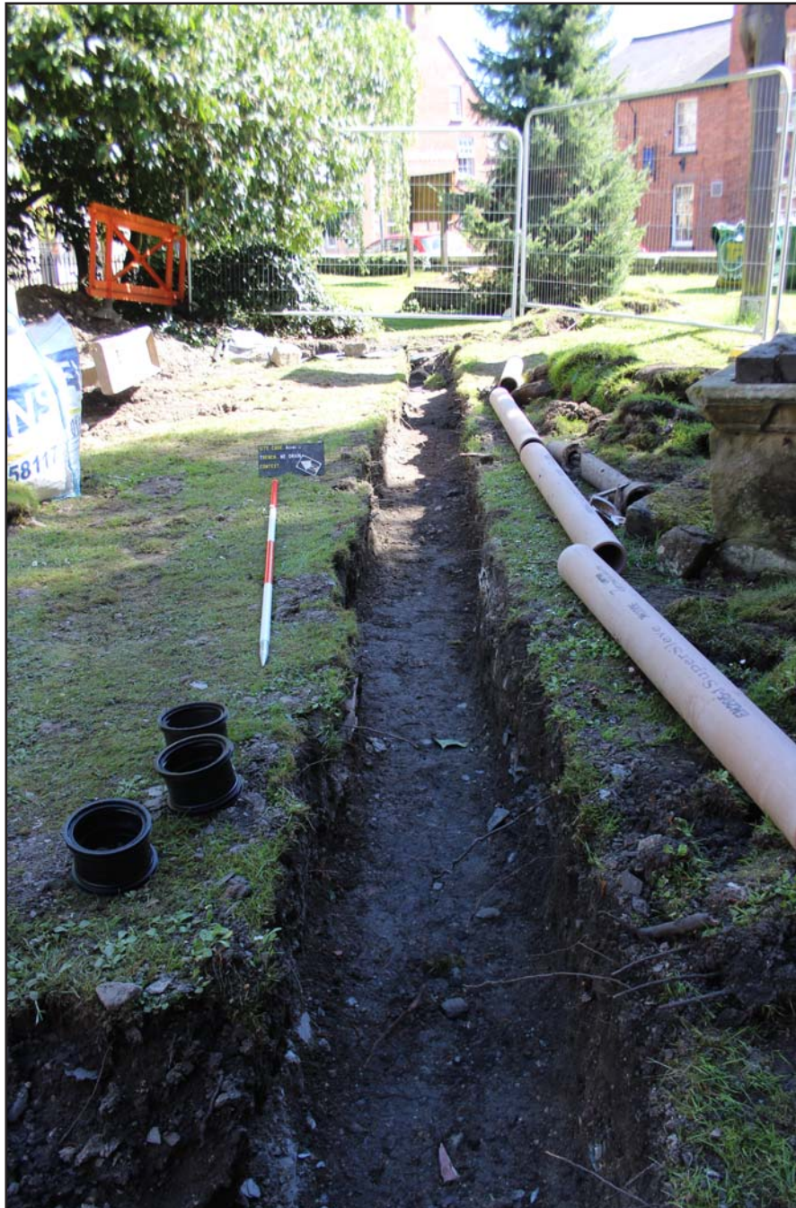
Plate 05: Excavated trench for Drain 2 - from the southwest - scale 2m
