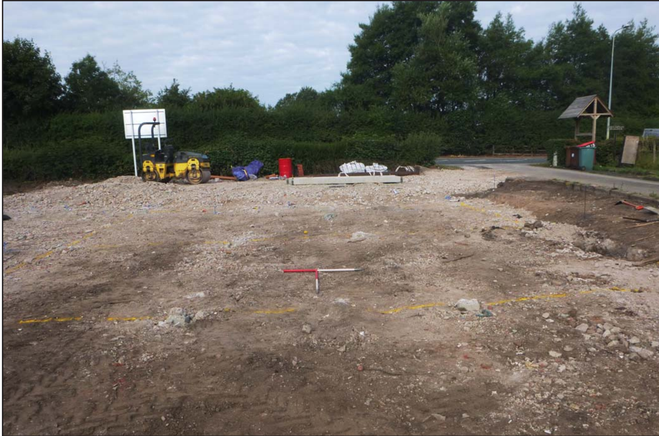
Plate 01: Pre excavation shot - from the east - scale (2x) 1m
