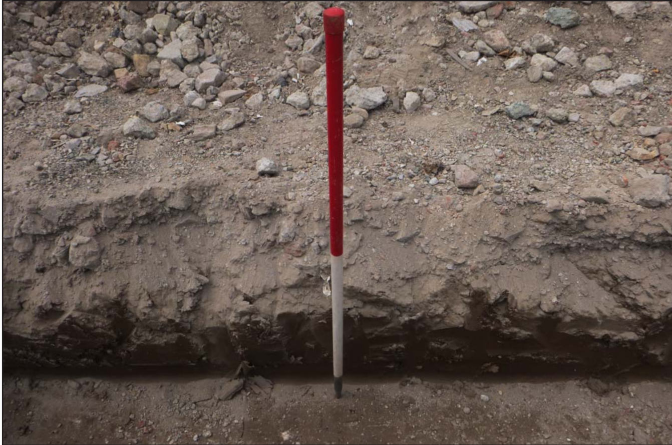
Plate 07: Section of western footing - from the east - scale 1m
