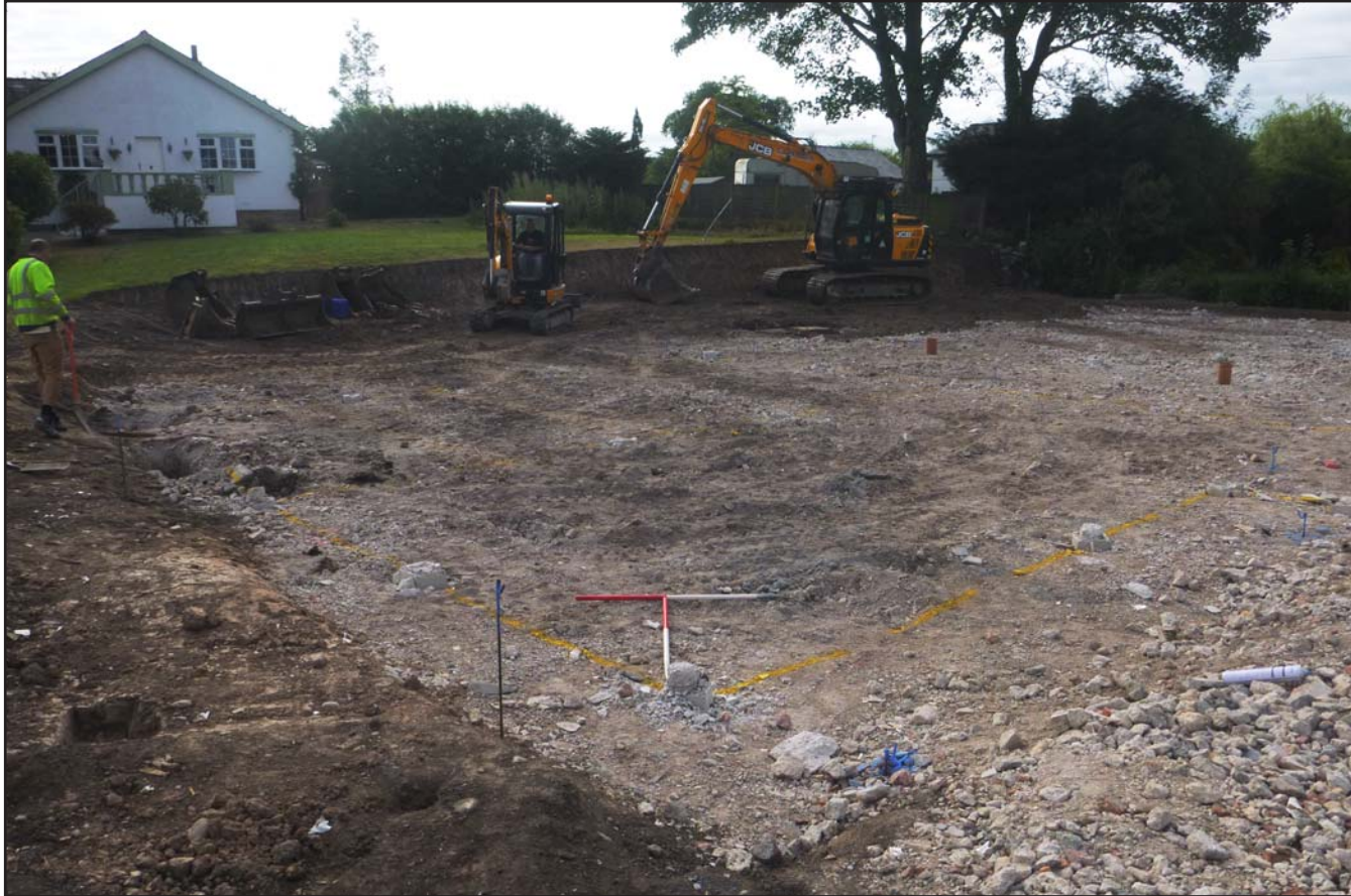
Plate 02: Pre excavation shot - from the northwest - (2x) 1m
