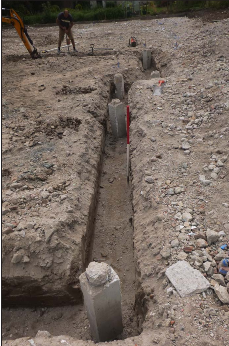
Plate 08: Western footing in context with site - from the north - 1m scale
