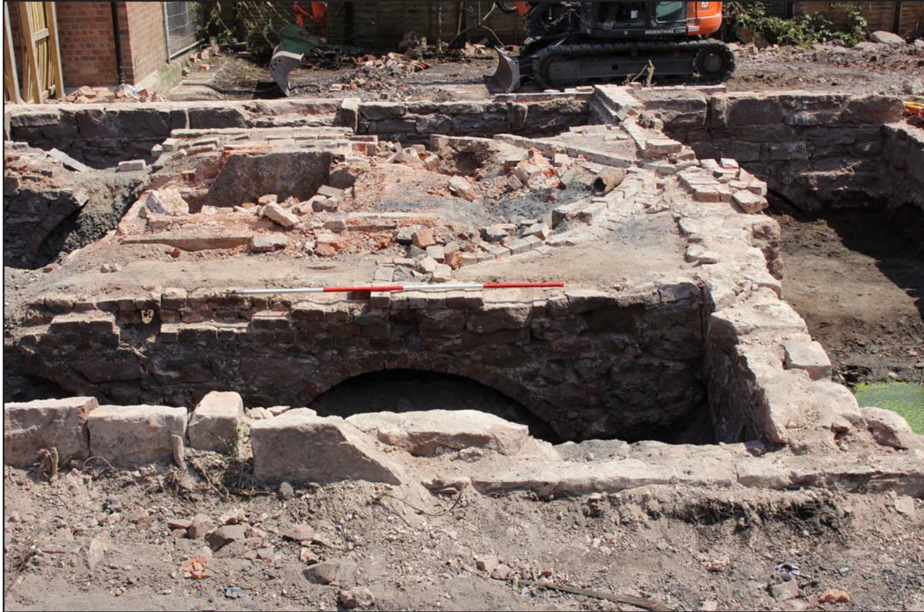
Plate 24: Context shot showing drain area and archway (175) - from the west - scale 2m
