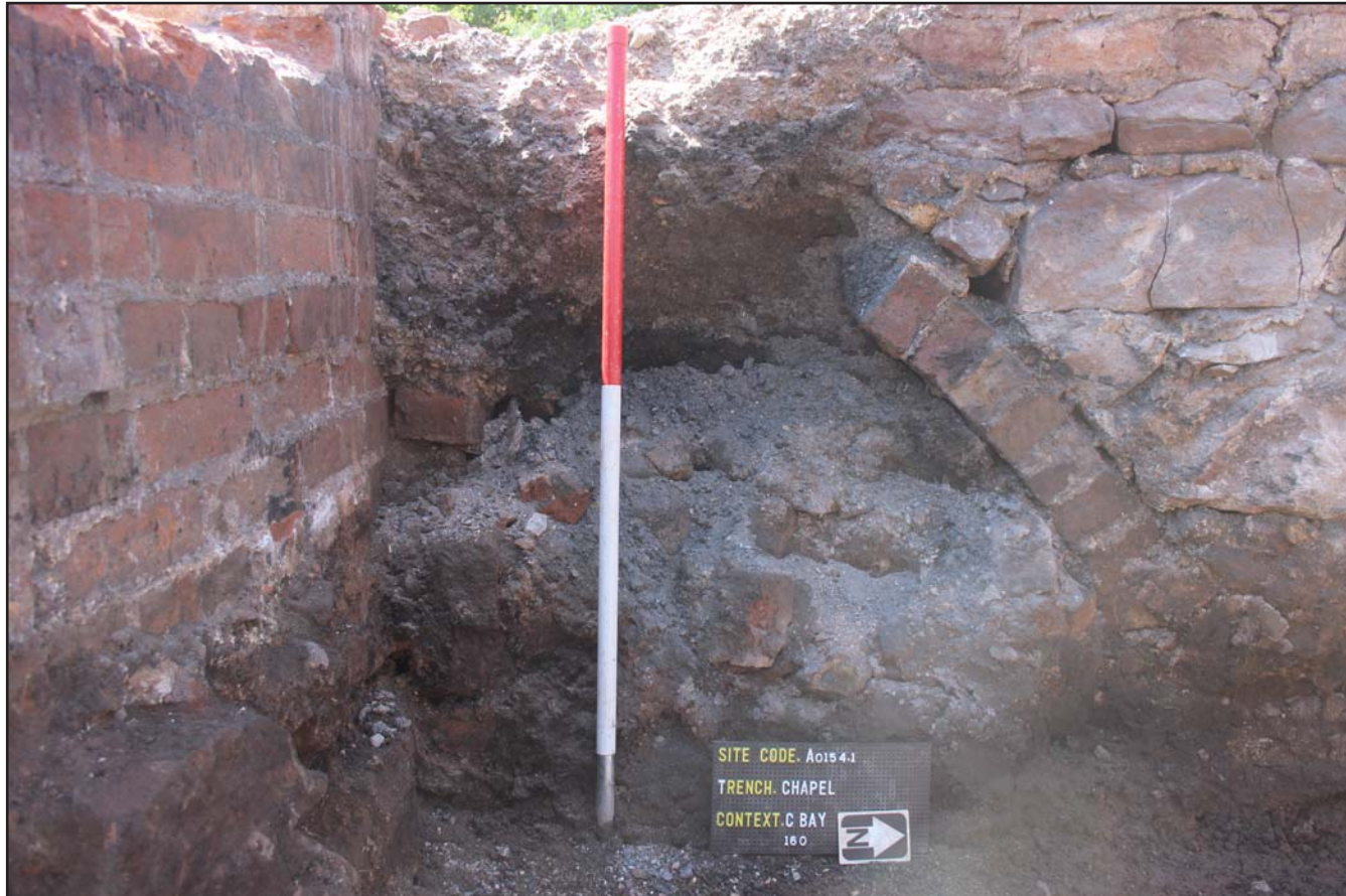
Plate 31: Shot showing physical relationship between interior wall (139), Archway (160) and drain (south eastern corner) - from the east - scale 1m
