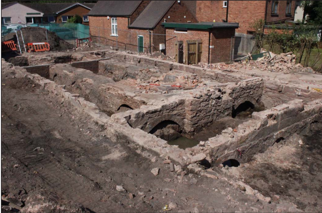
Plate 08: Post-excitation oblique shot of Baptist Pool (128) - from the southwest - 2m
