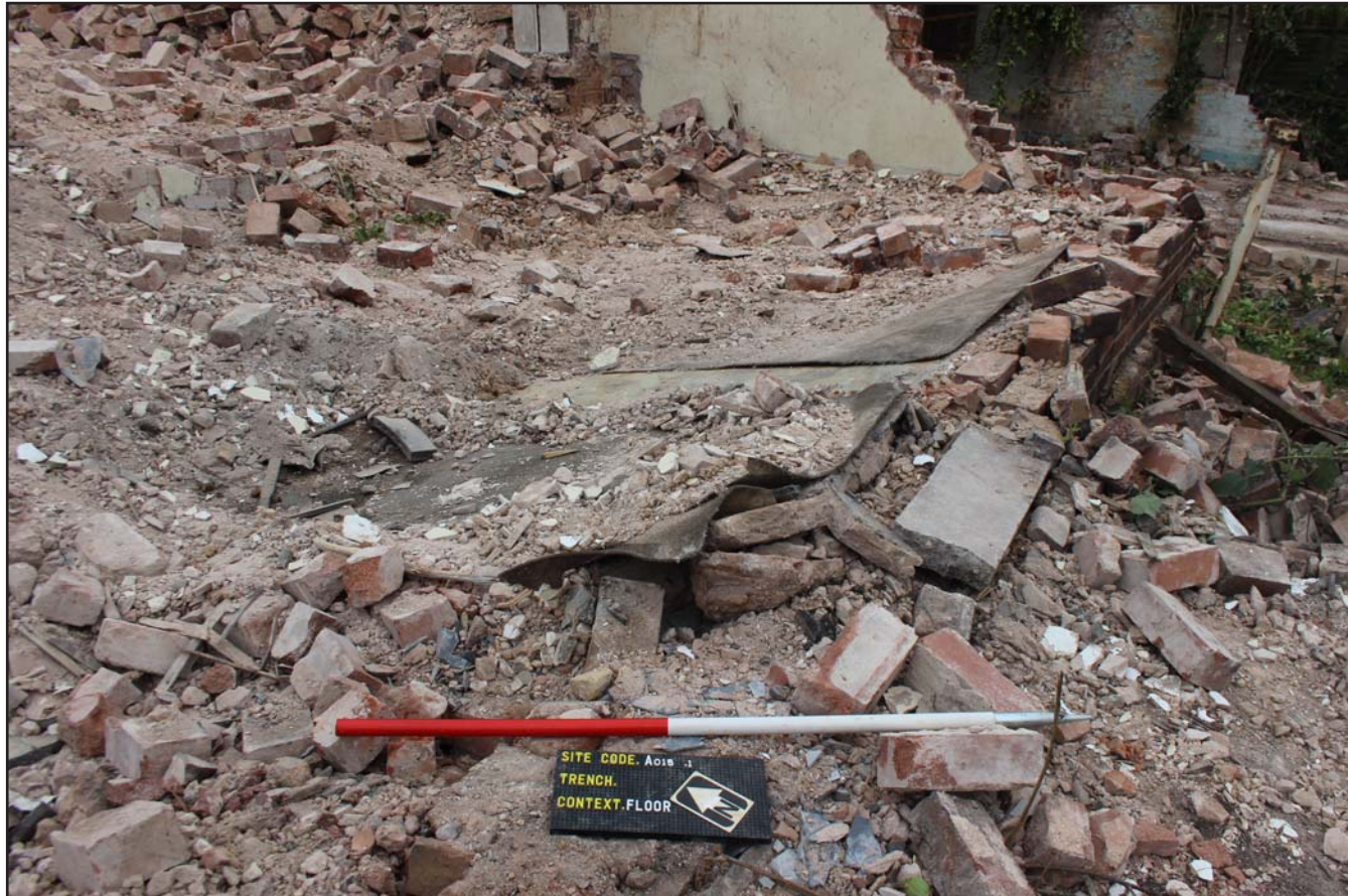
Plate 04: Concrete slab (101) in situ prior to lifting - from the southwest - scale 1m
