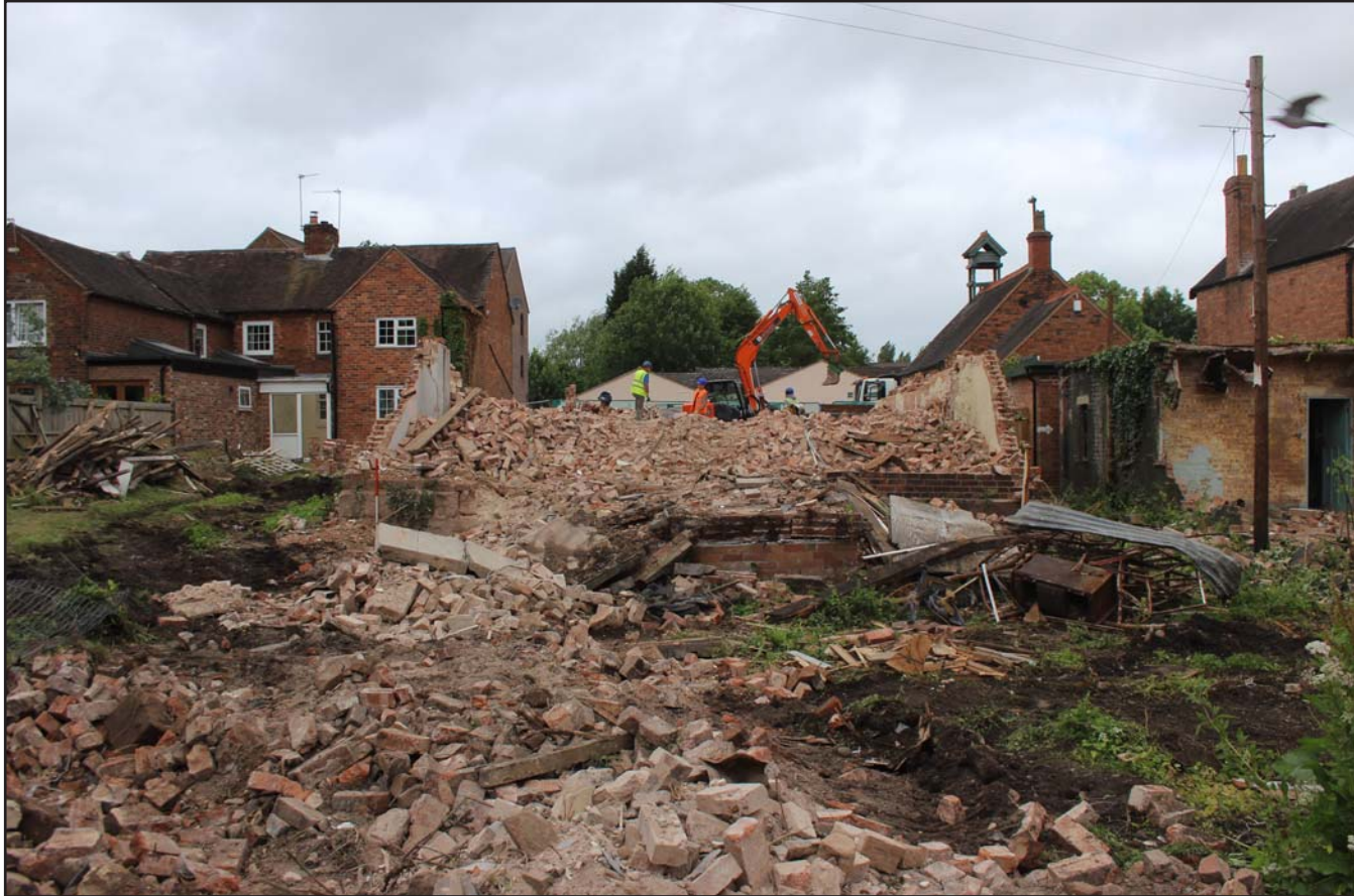
Plate 01: Pre-excavation shot of Zionist Baptist Chapel - from the south - scale 1m
