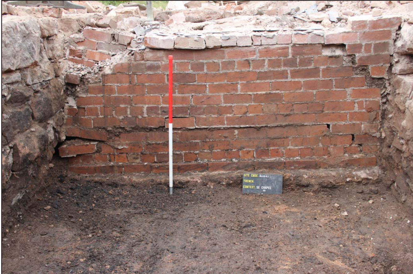
Plate 35: Dividing wall (111) in southern bay - from the east - scale 1m
