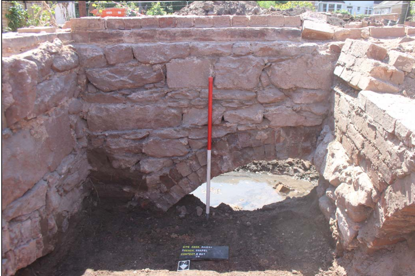
Plate 57: Shot showing relationship between exterior wall (123) and southern interior wall (110) and that wall (122) abuts over archway (113) located within wall (110) - from the north - scale 1m
