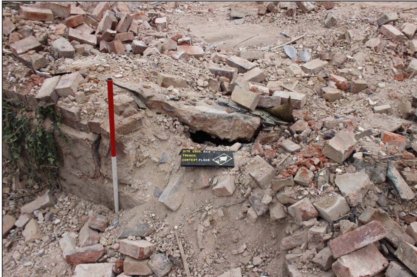
Plate 41: Concrete floor slab (101) collapsed into void - from the southeast - scale 1m
