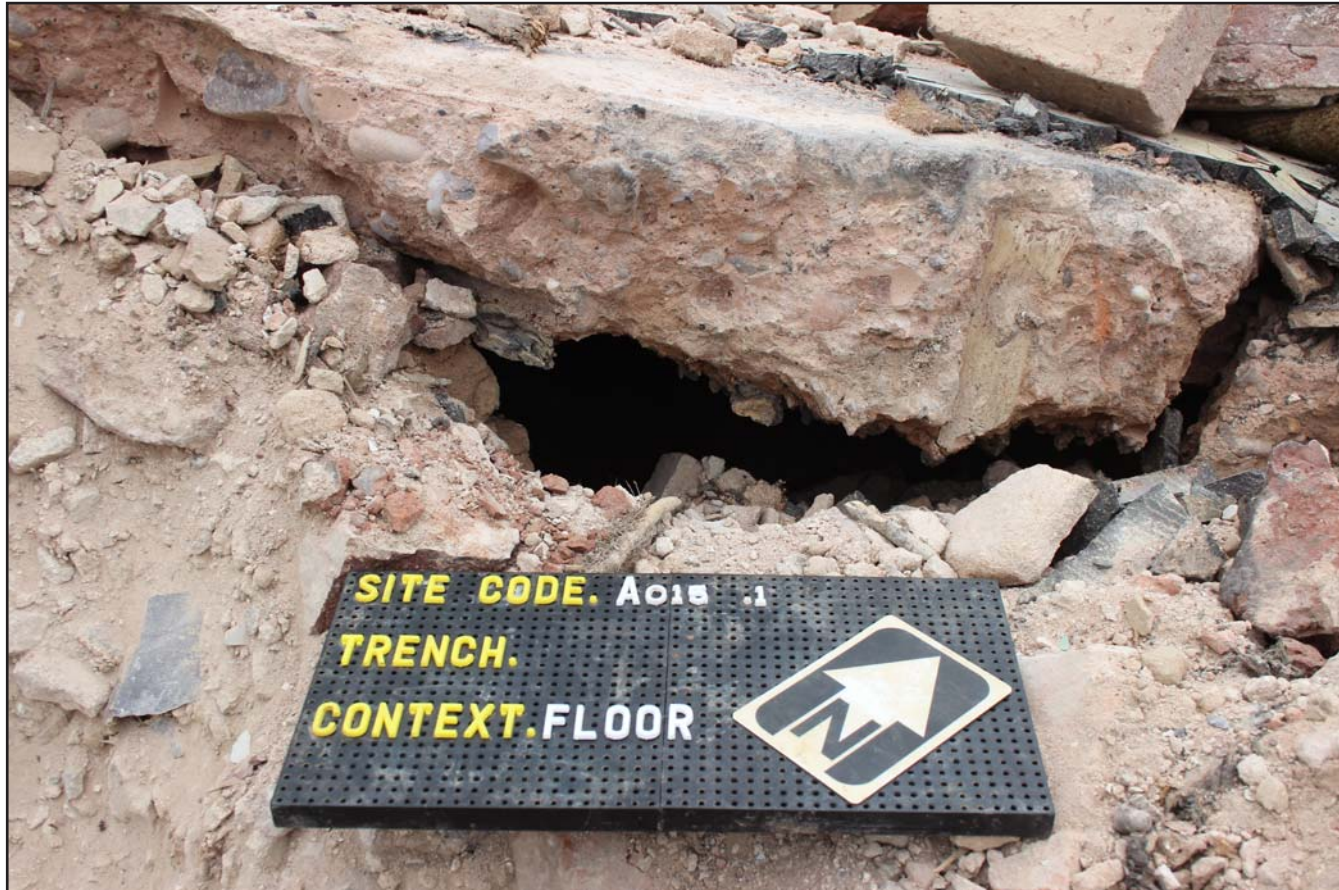
Plate 42: Concrete floor slab (101) collapsed into void (close up) - from the southeast - scale n/a
