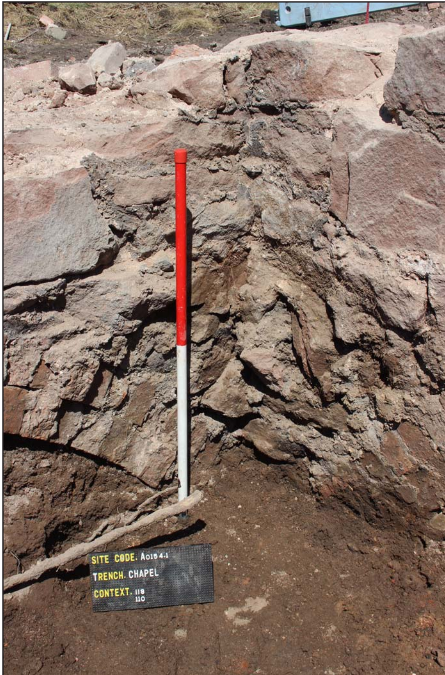
Plate 55: Section showing physical relationship between interior wall (110) and exterior wall (127) - from the southeast - scale 1m
