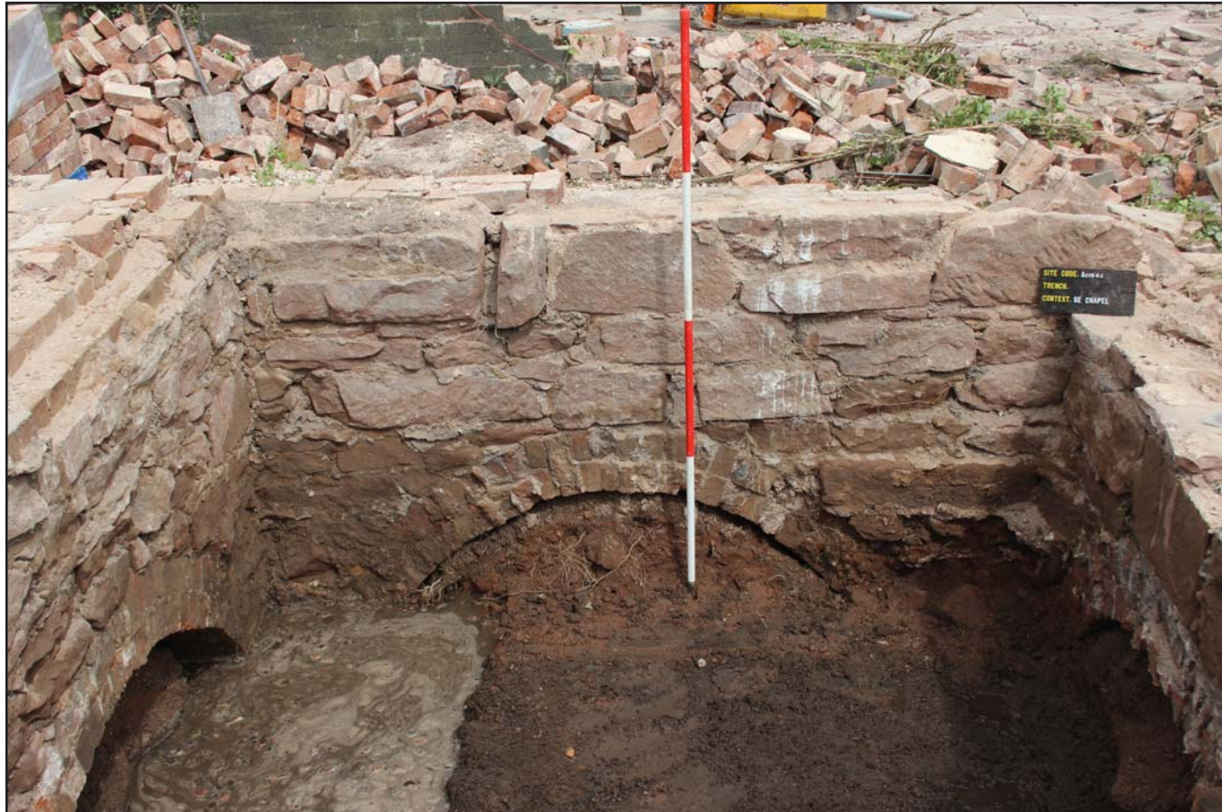
Plate 13: Shot showing example of wall and arch construction (southwestern corner of chapel) - from the west - scale 2m
