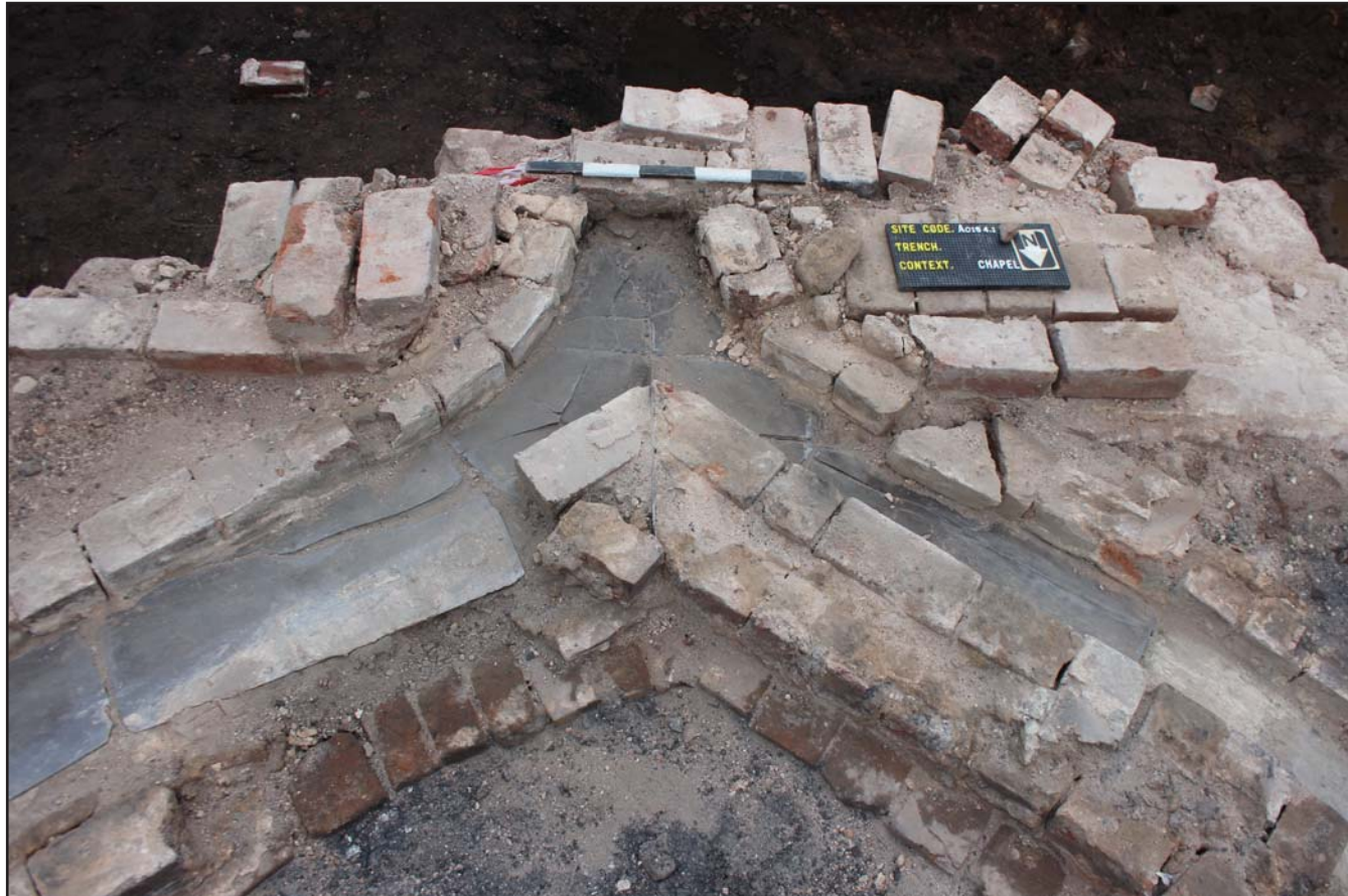
Plate 21: Point at which drains (131) & (132) are connected on top of buttress (112 - from the west - scale 0.5m
