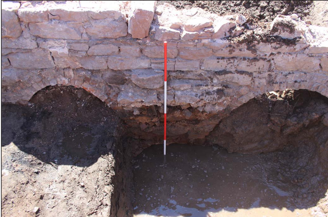
Plate 14: Shot showing visible depth of arches (southern wall of chapel) the sandstone base is obscured by water table - from the north - scale 2m
