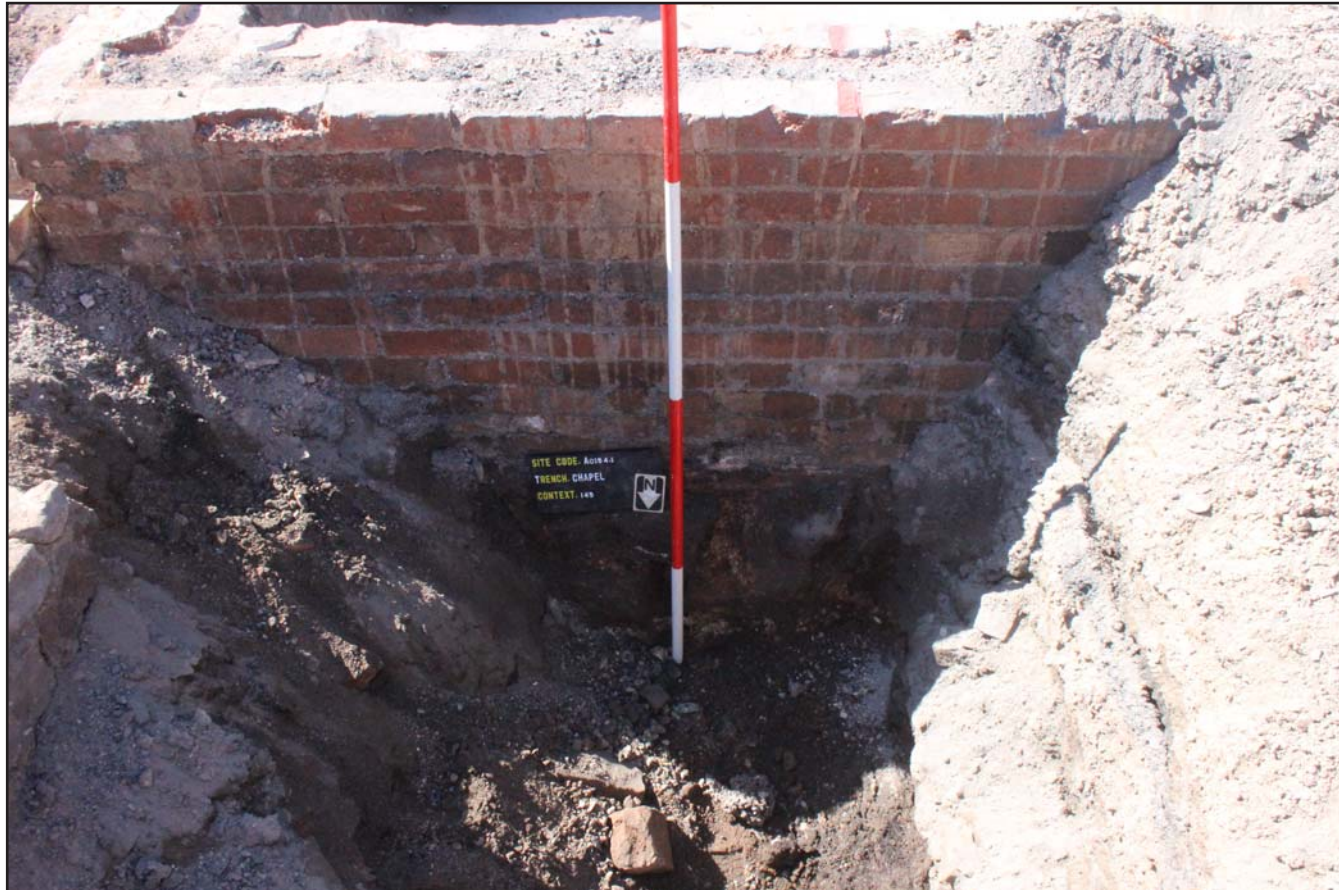
Plate 28: Northern wall of baptismal pool (128) showing sandstone foundation below (145) - from the north - scale 2m
