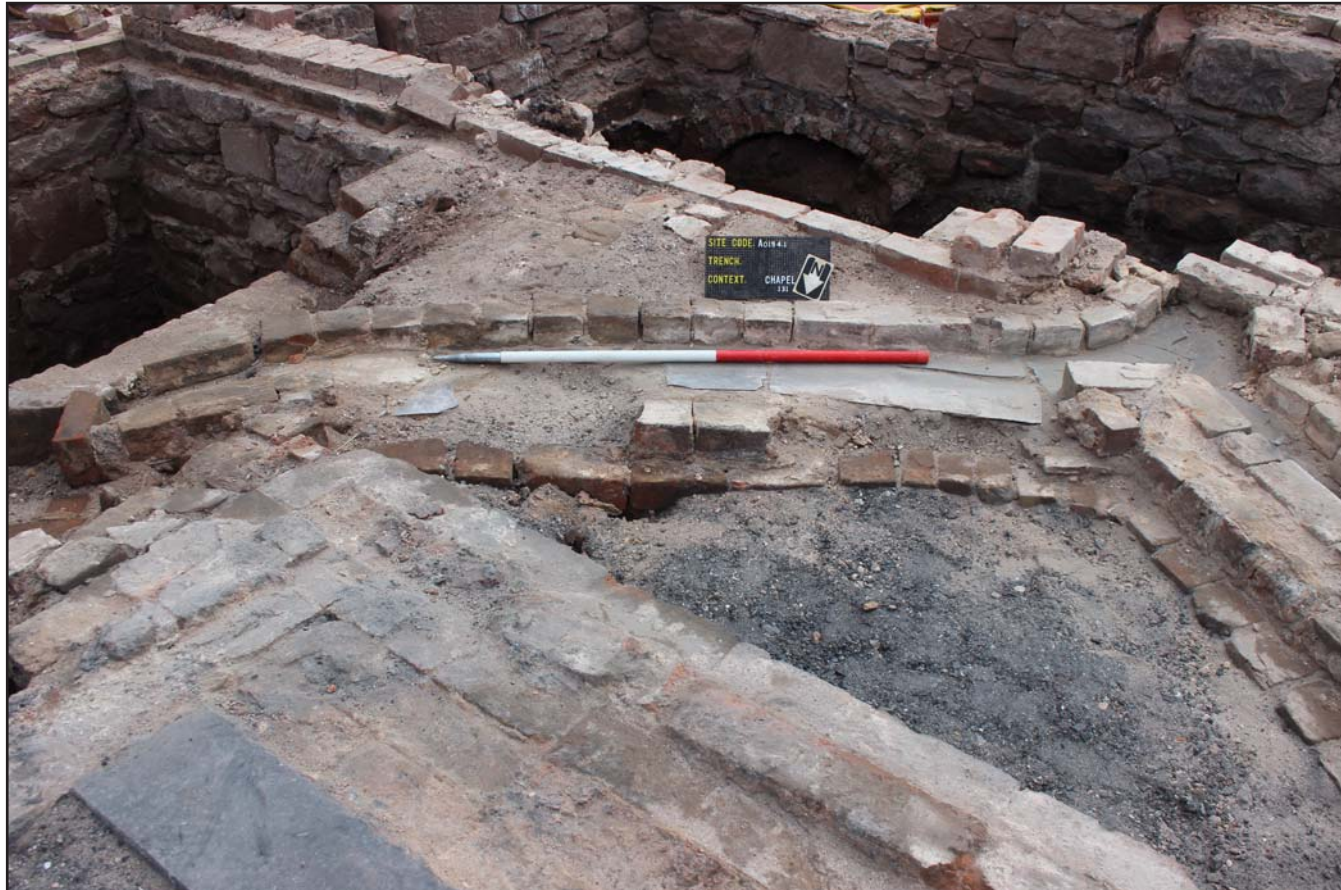
Plate 17: Eastern drain (131) - from the northwest - scale 1m
