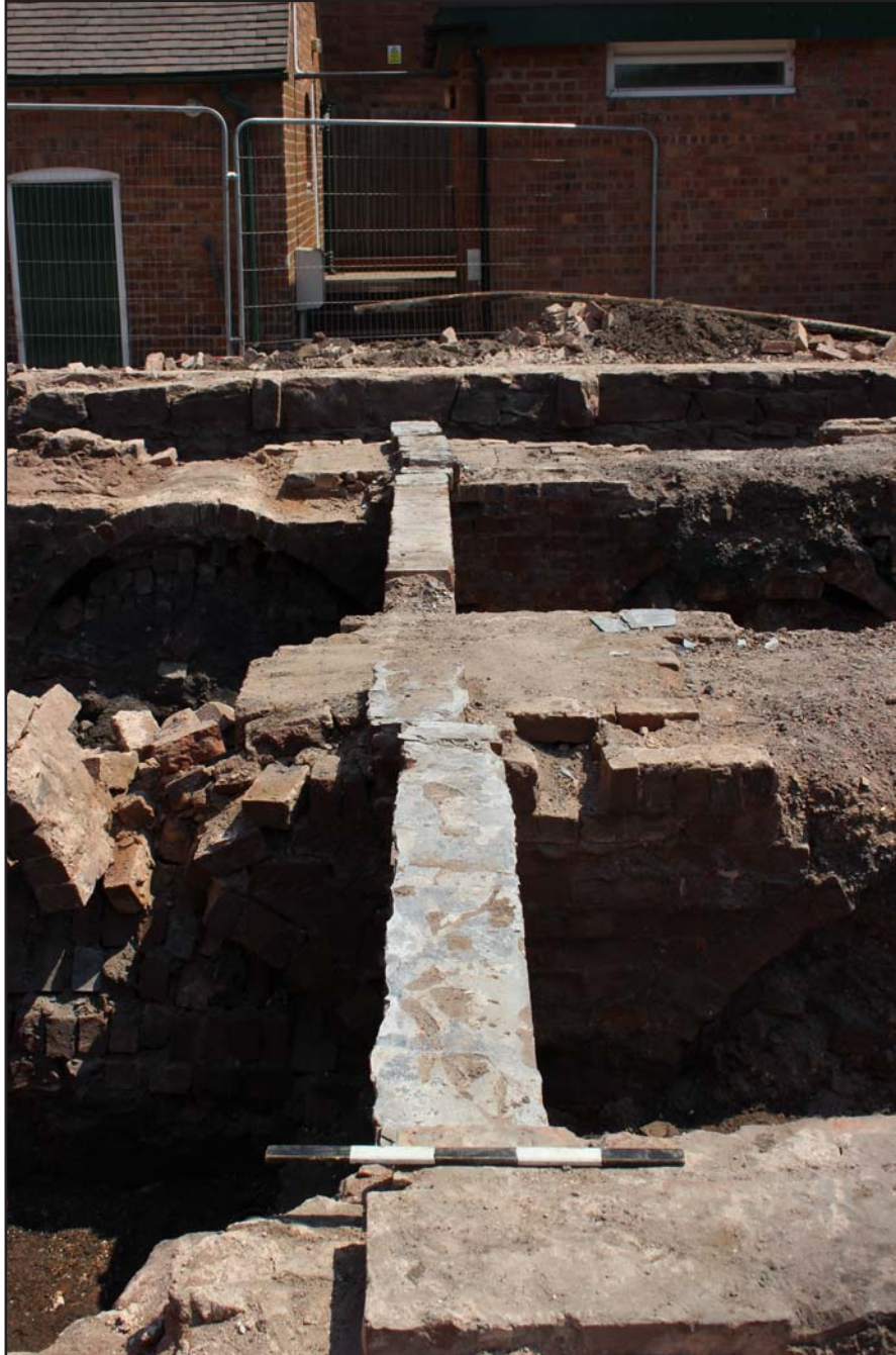
Plate 37: Context shot across dividing walls (168) (foreground) & (159) (background) - from the west - scale 0.5m
