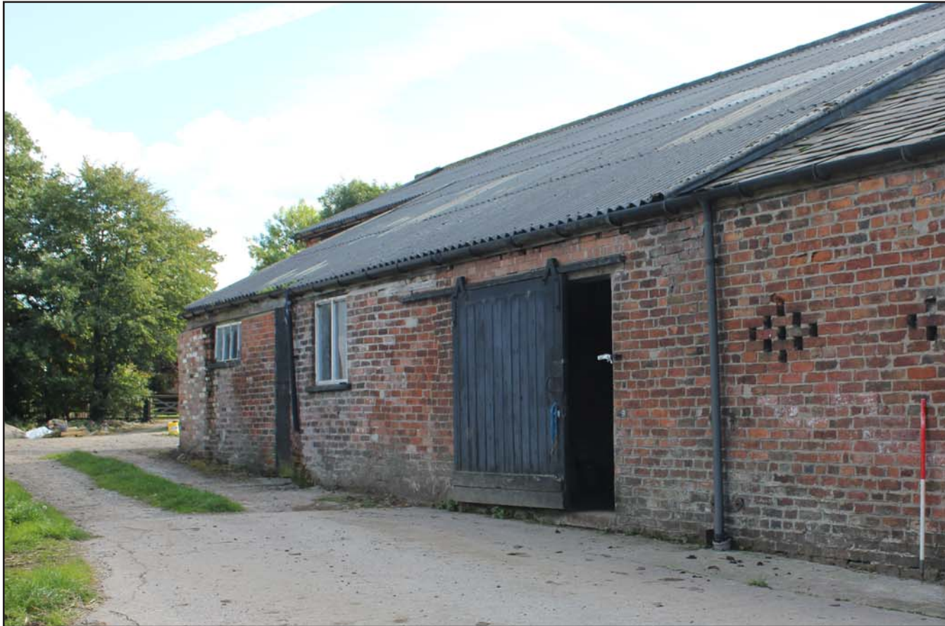
Plate 14: Grimsditch Farm - Northeast Extension northeast external elevation, from the north. Scale 1.0m.
