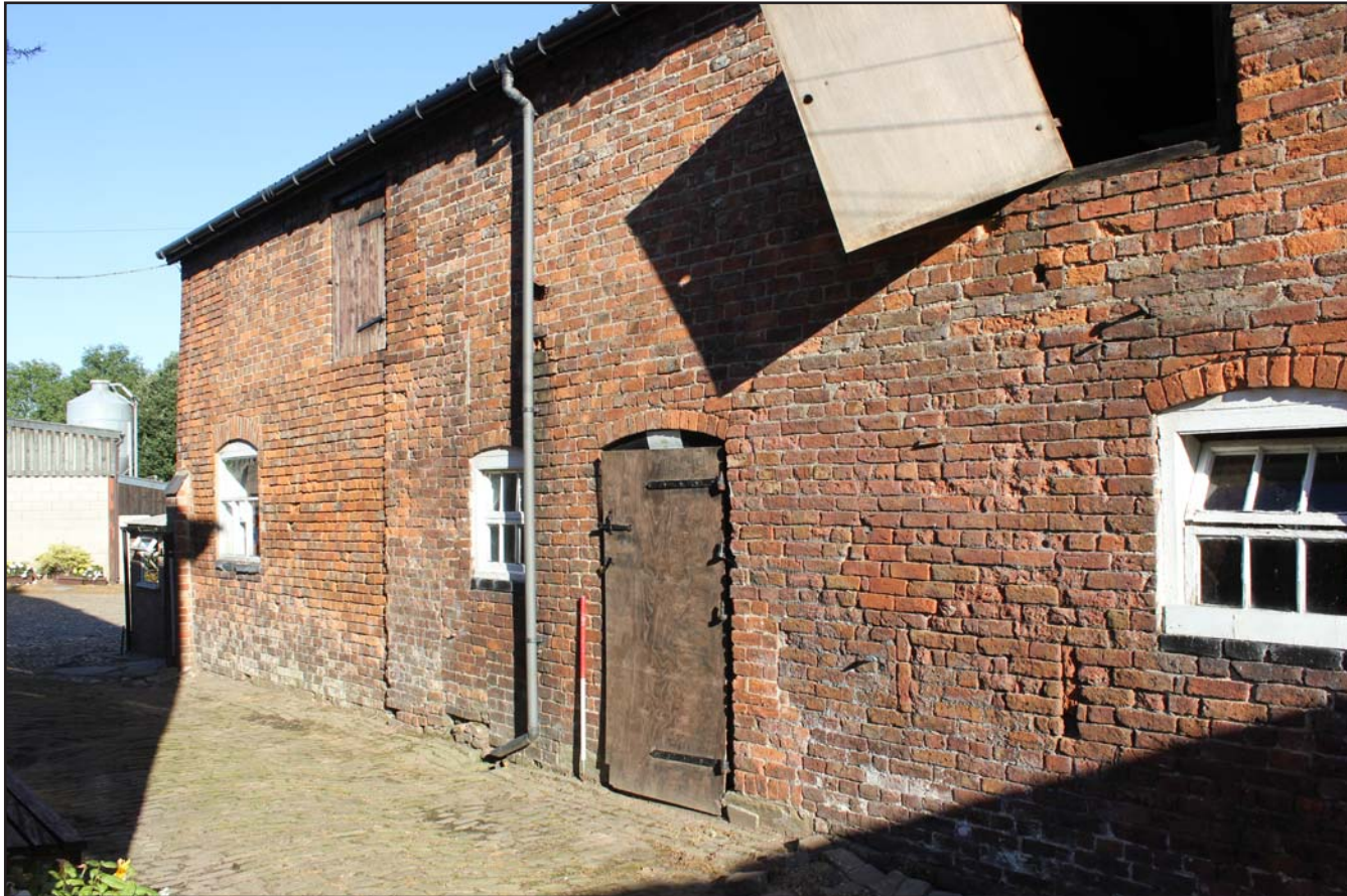
Plate 03: Grimsditch Farm - Barn southwest external elevation, from the south. Scale 1.0m.
