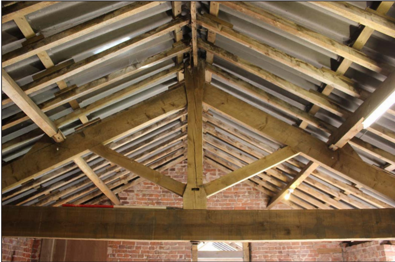
Plate 25: Grimsditch Farm - Barn interior (first floor) showing Queen Post truss, from the northwest. Scale 1.0m.
