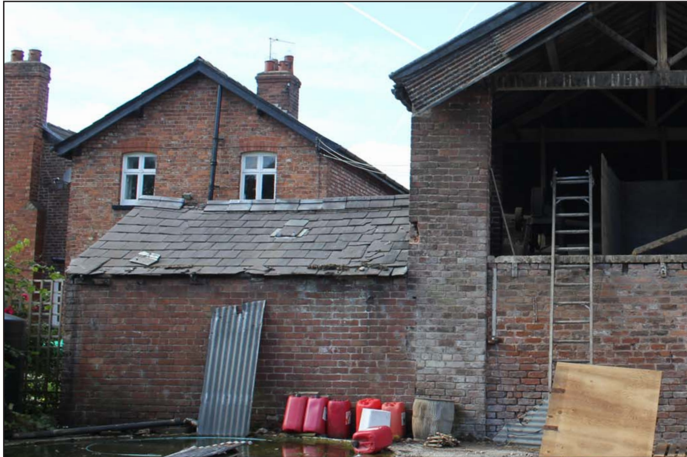
Plate 17: Grimsditch Farm - Southwest Extension southeast external elevation, from the southeast.
