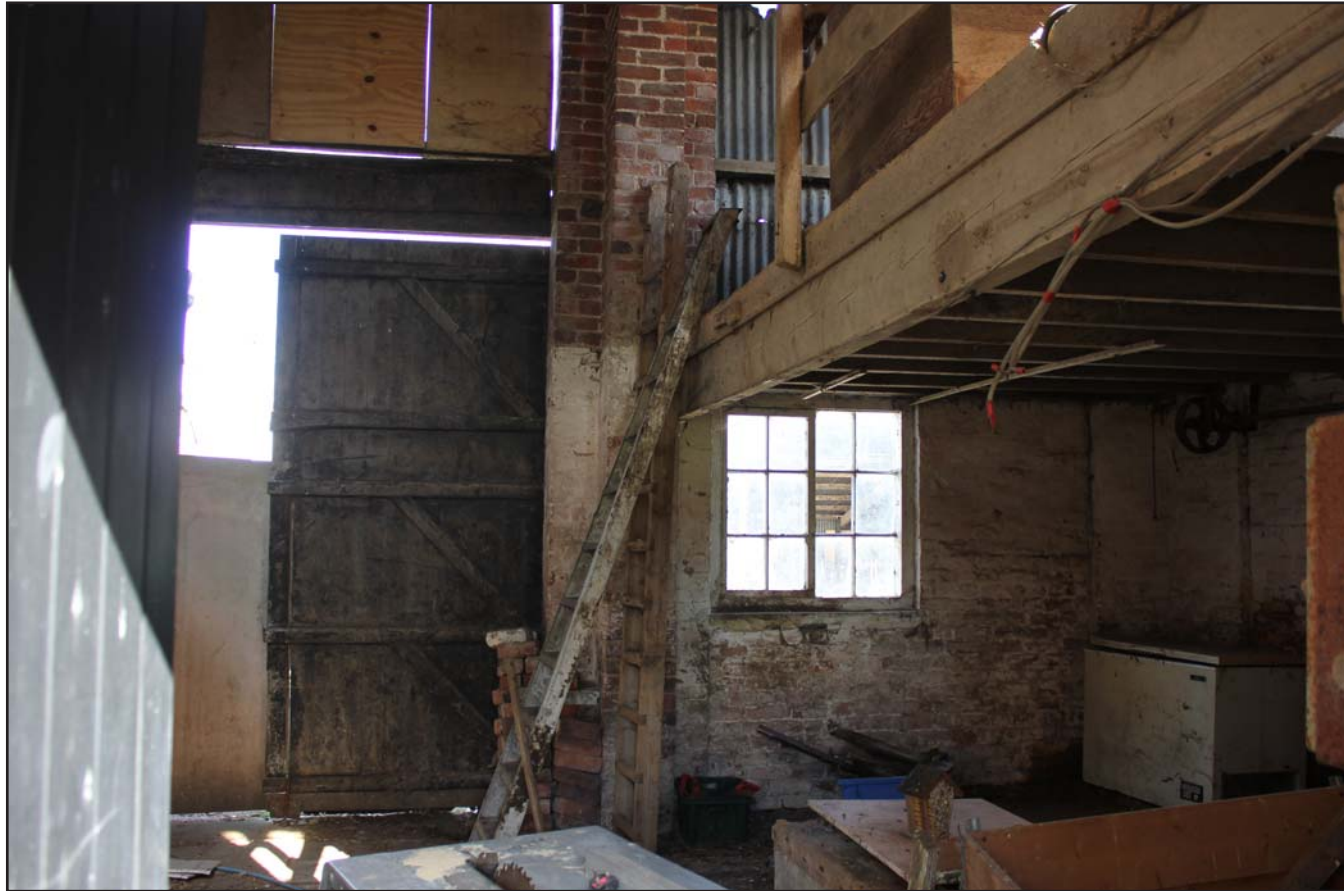
Plate 26: Grimsditch Farm - Hay Barn interior, from the west.
