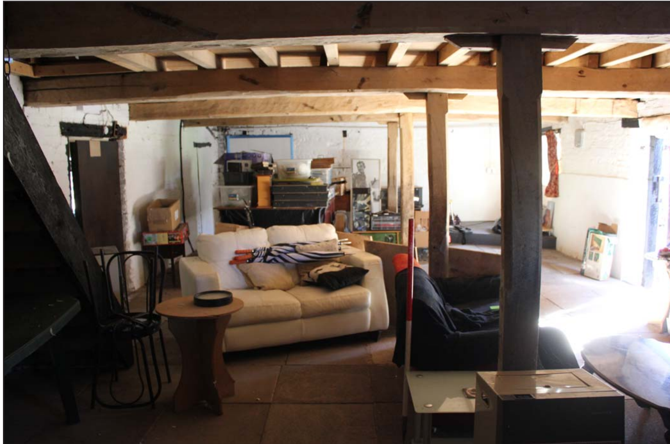
Plate 22: Grimsditch Farm - Barn interior, from the northwest. Scale 1.0m.
