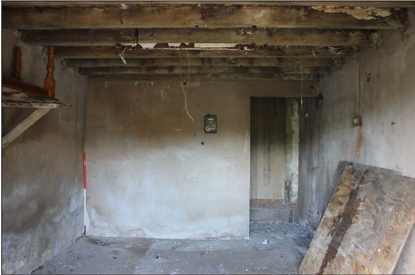
Plate 29: Grimsditch Farm - Northwest Extension Store interior, from the northeast. Scale 1.0m.
