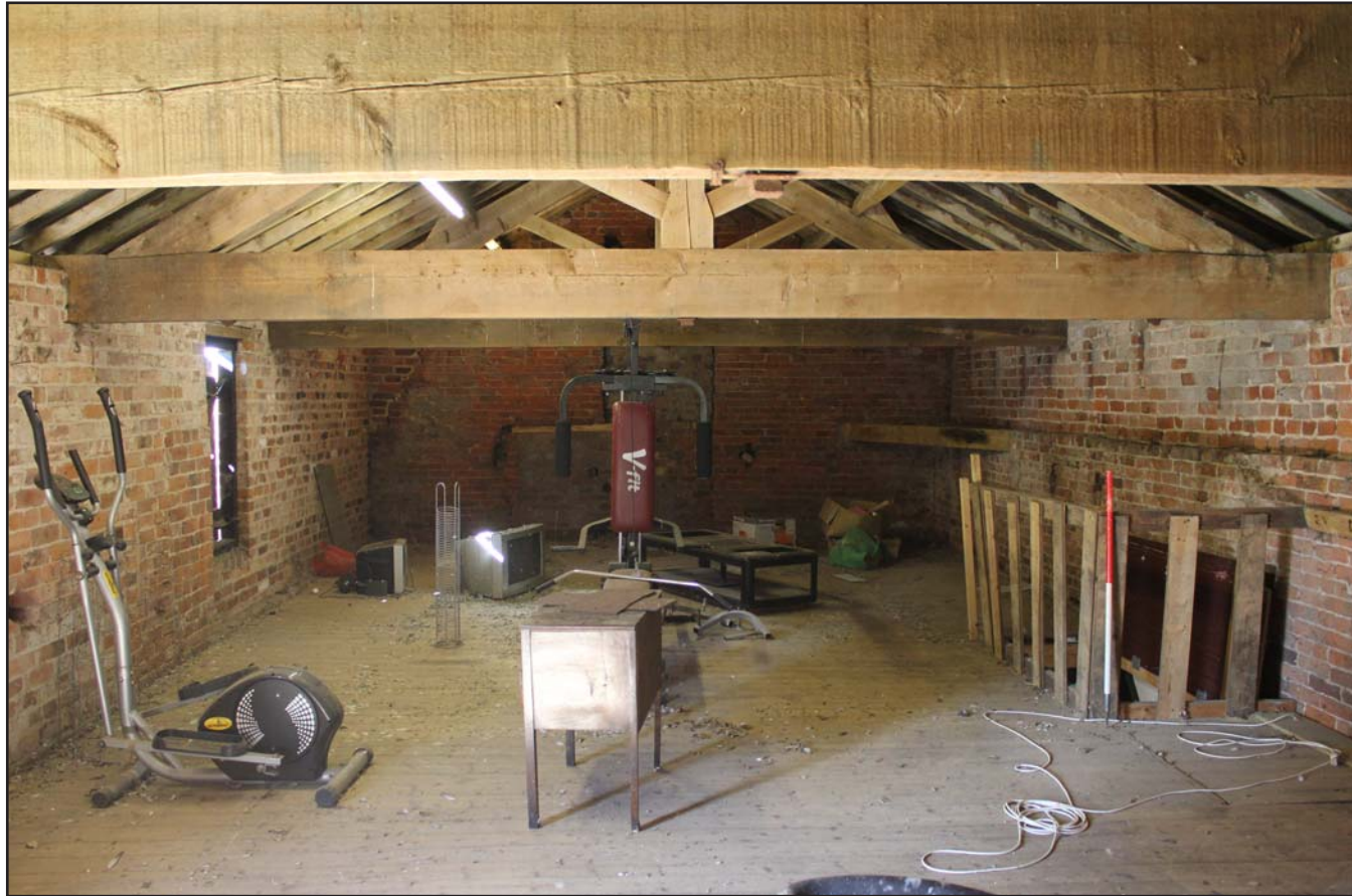
Plate 24: Grimsditch Farm - Barn interior (first floor), from the southeast. Scale 1.0m.
