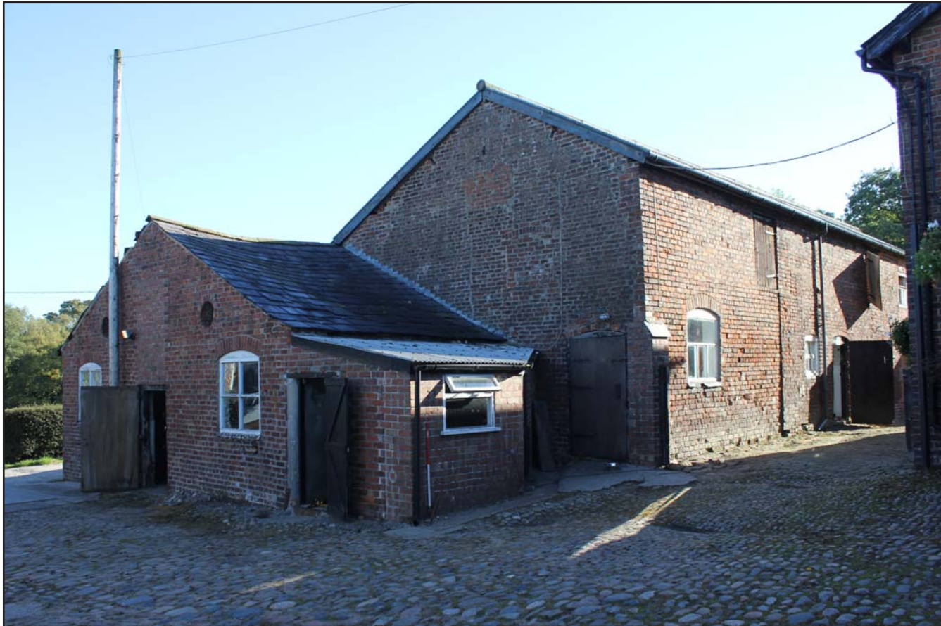
Plate 01: Grimsditch Farm - Barn northwest and southwest external elevations, from the west. Scale 1.0m.
