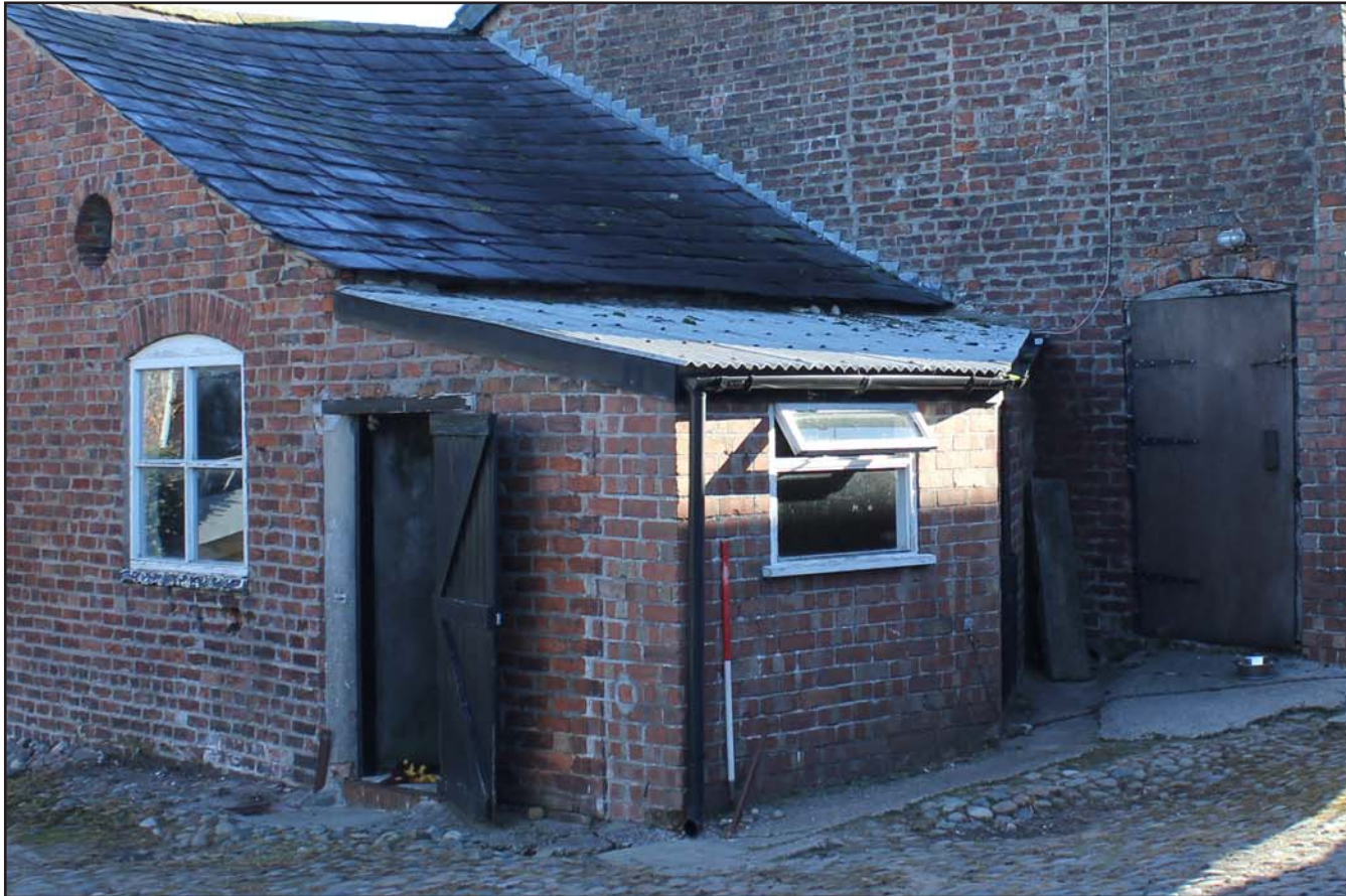
Plate 19: Grimsditch Farm - Kennel Extension northwest and southwest external elevations, from the west. Scale 1.0m.
