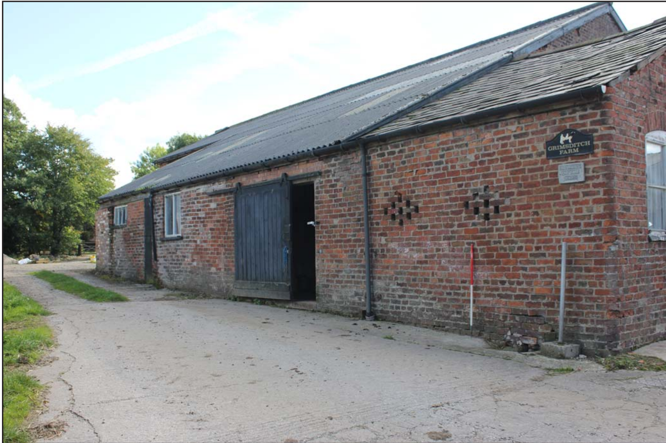
Plate 09: Grimsditch Farm - Northwest Extension northeast external elevation, from the north. Scale 1.0m.
