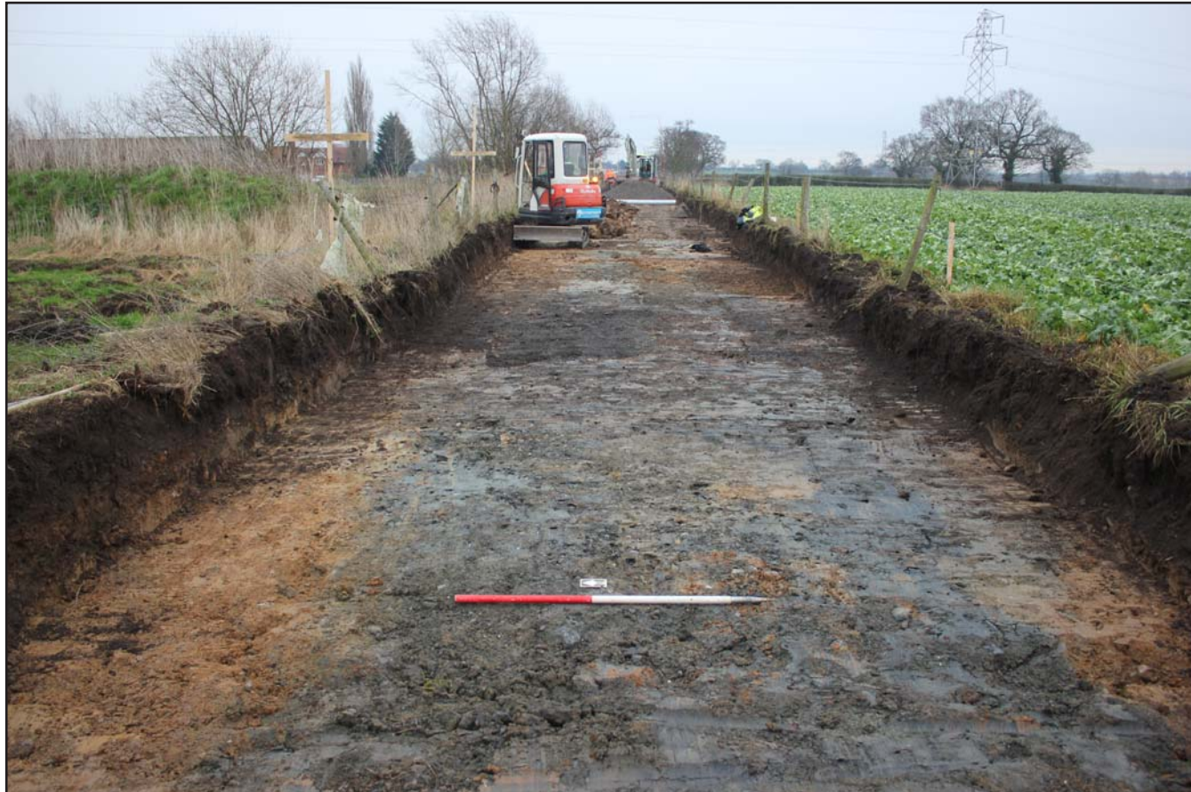
Plate 15: Shot of exposed Roman Road alignment (from lower angle) - from the west - scale 1m
