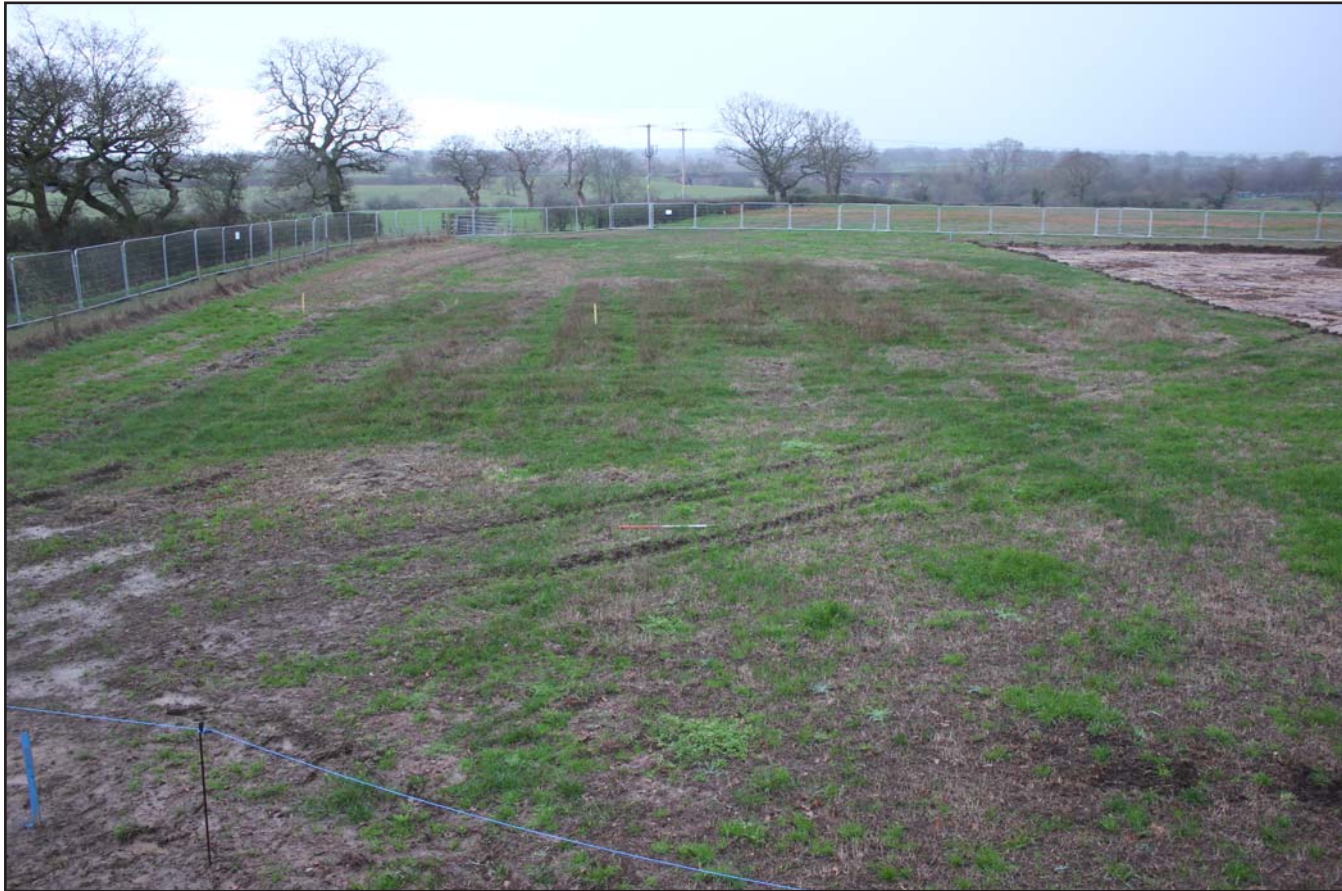
Plate 19: Pre excavation shot of 25m wide development corridor (eastern end of site) - from the northwest - 1m scale
