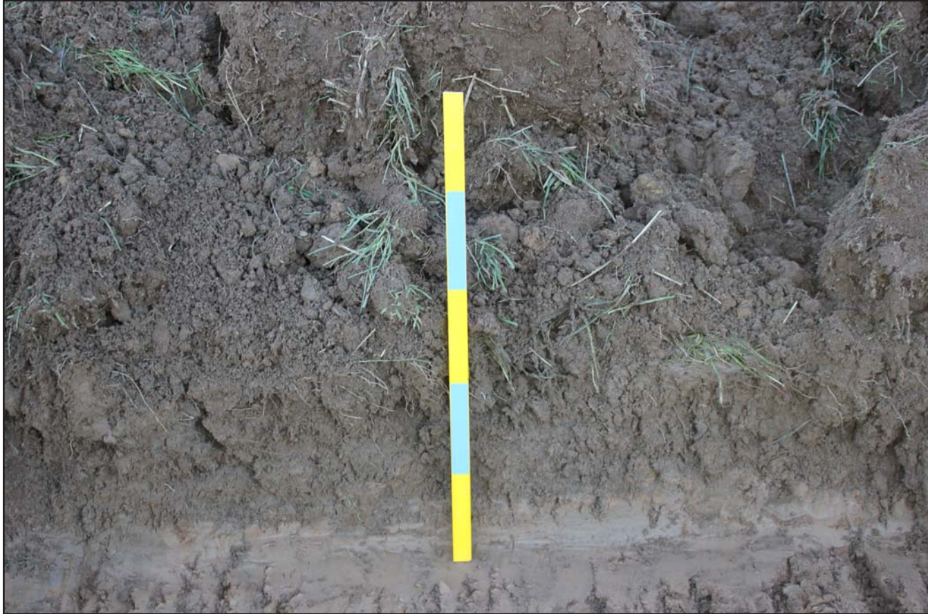
Plate 22: Generic section showing stratigraphy (in 25m development corridor area) - from the southwest - 0.50m scale
