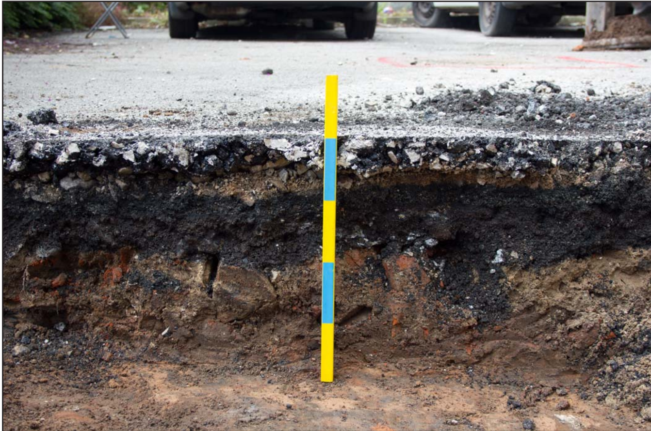
Plate 08: Generic section of trench - from the northwest - scale 0.50m
