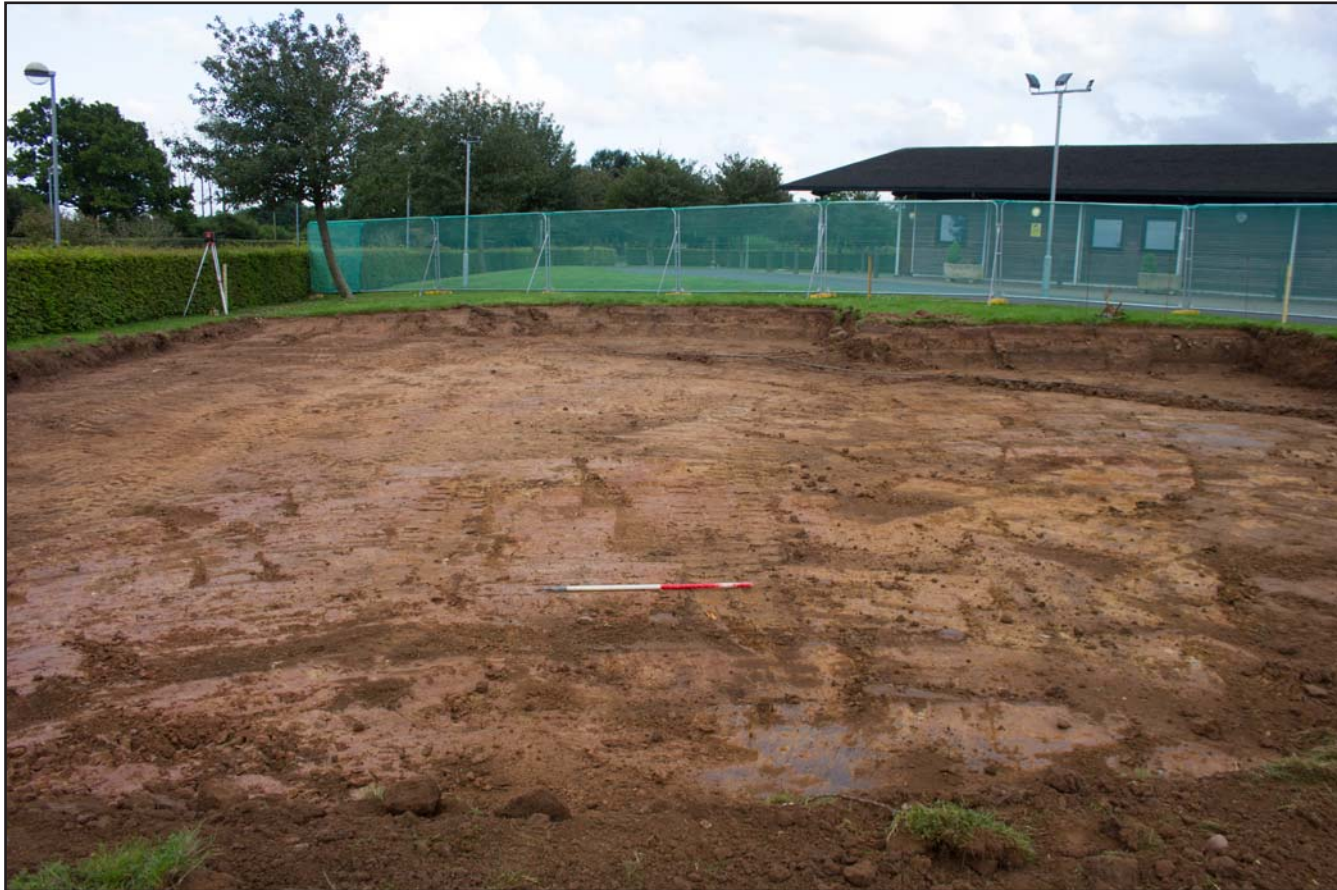
Plate 08: Post excavation shot of area; Car Park B at Telford Crematorium, Woodhouse Lane, Redhill, Shropshire, TF2 9NJ - from the northwest - scale 1m.
