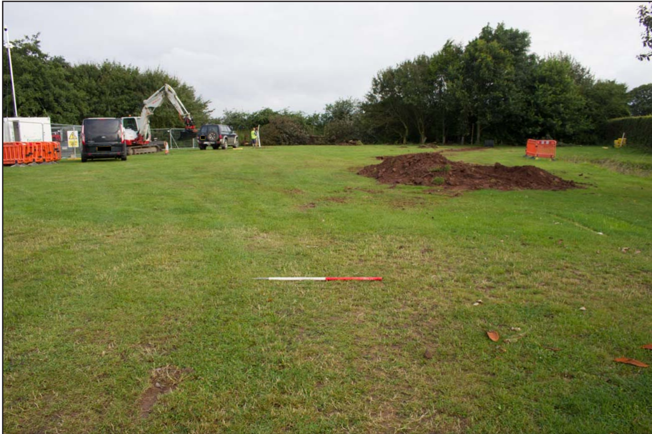
Plate 01: Pre excavation shot of area; Car Park A at Telford Crematorium, Woodhouse Lane, Redhill, Shropshire, TF2 9NJ - from the southeast - scale 1m.
