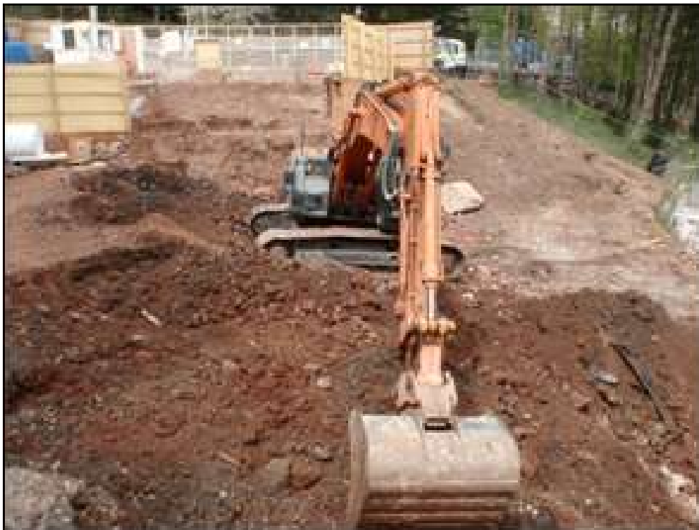
Plate 3 General view of the reduced level excavation for the basement. Looking NW.
