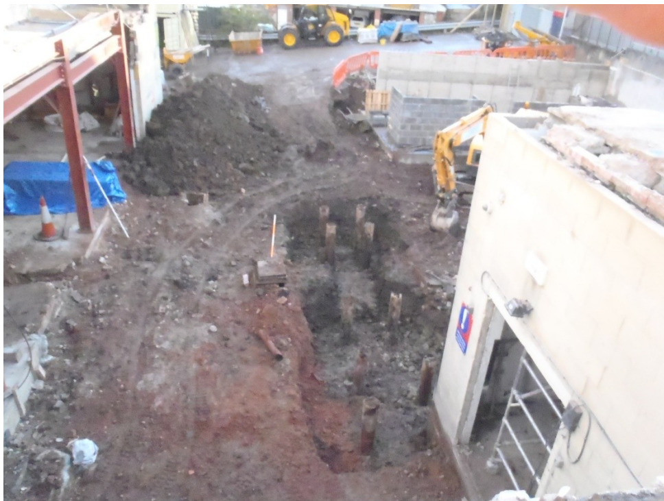
Plate 5. General view across site looking south following bulk excavation, showing completed excavations for pile caps and ground beams. Scale 1x2m.
