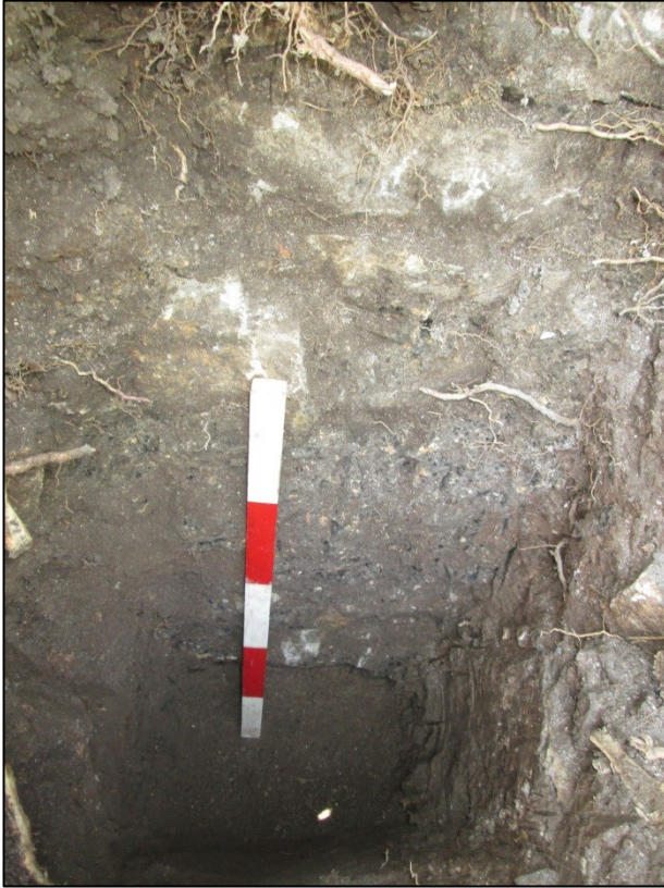
Plate 7. Sondage to test depth of existing building foundations, looking W. Scale 0.5m.
