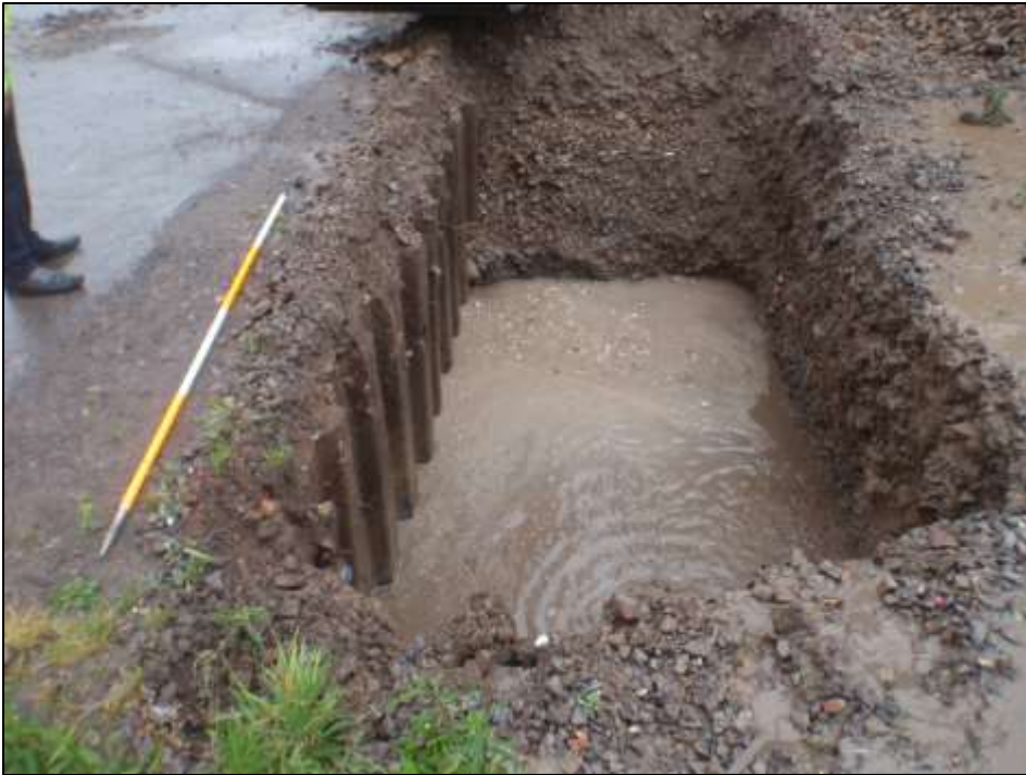
Plate 5. STP 9 as excavated, looking W, scale 2m.
