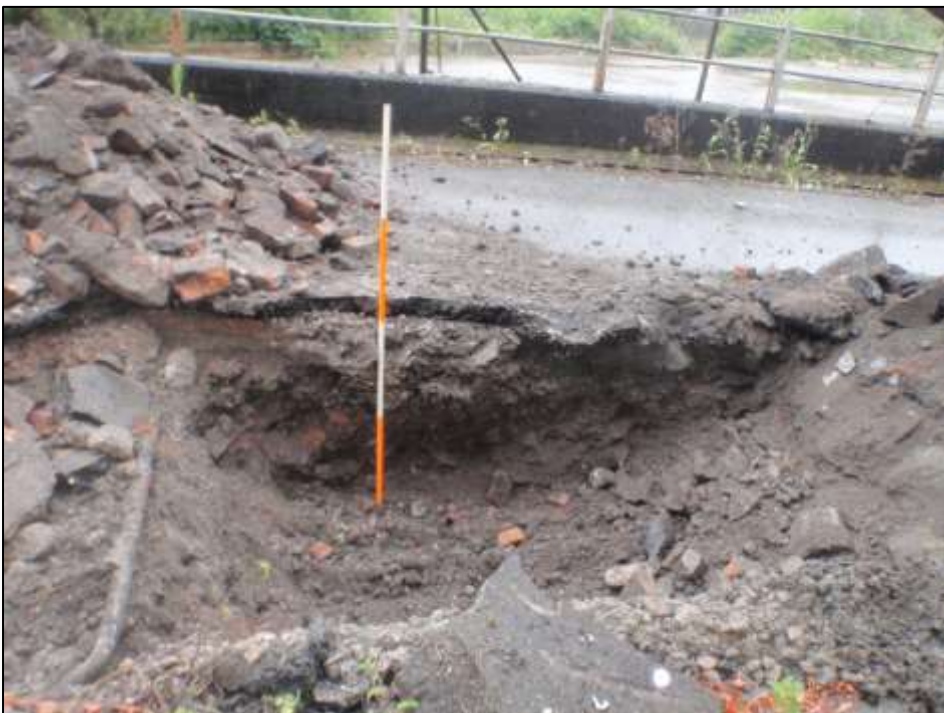
Plate 4. STP 07 as excavated to lower concrete surface, looking E
