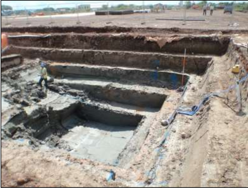
Plate 3. Petrol Interceptor Tank as excavated, looking SW. Scale 2m.
