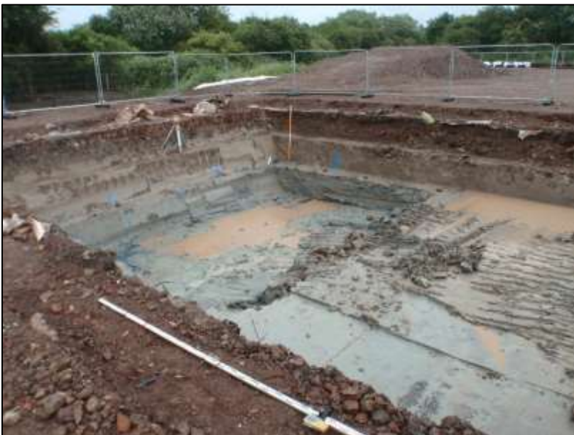
Plate 2. Petrol Interceptor Tank as excavated, looking N, scale 2m.
