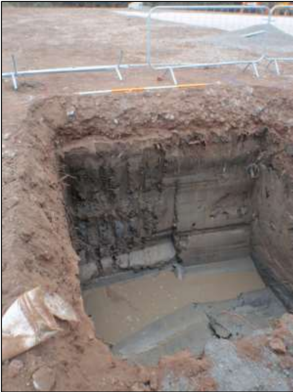
Plate 1. Sewage Treatment Plant Pit as excavated, looking NW, scale 2m.
