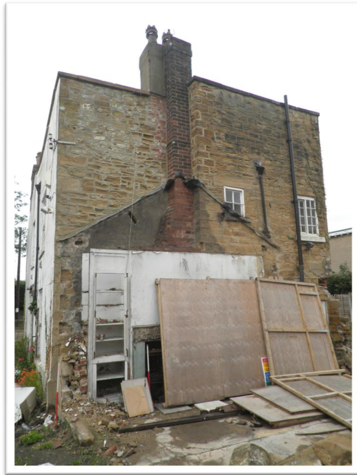
Plate 3: Northern elevation showing demolition of 1870s extension
