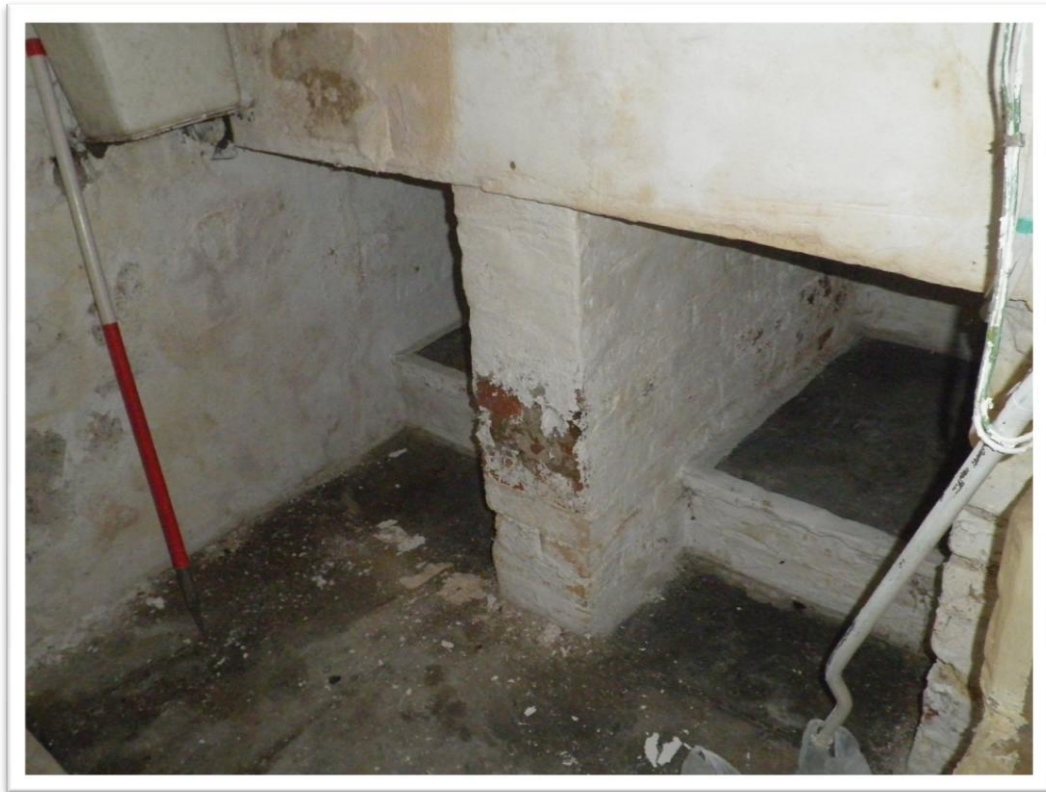
Plate 6: 19 th century brick storage bins (Room 4)
