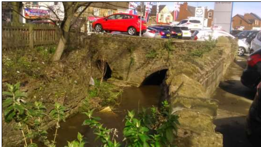
Plate 3: Detail of River Hipper entering culvert under site.
