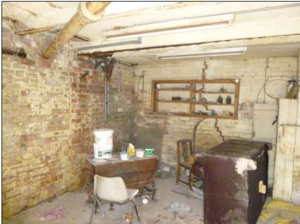
Plate 18: General view of sub-ground level
