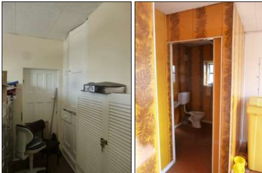
Plates 12 & 13: General view of former kitchen and later extension
