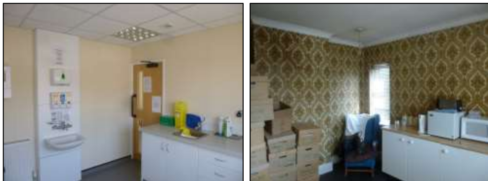
Plate 14 & 15: General view of refurbished and un-refurbished first floor
