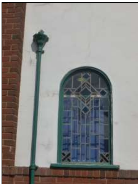
Plates 6 & 7: Examples of surviving stained glass windows and original downpipe
