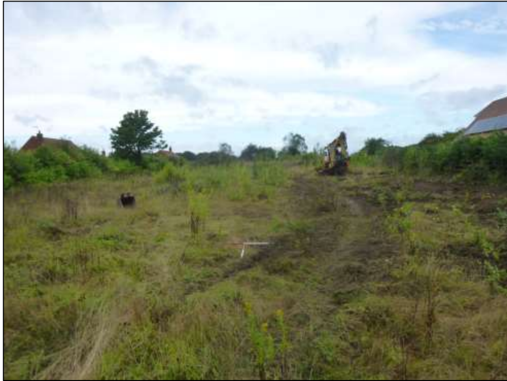
Plate 1: Site prior to excavation, looking west.
