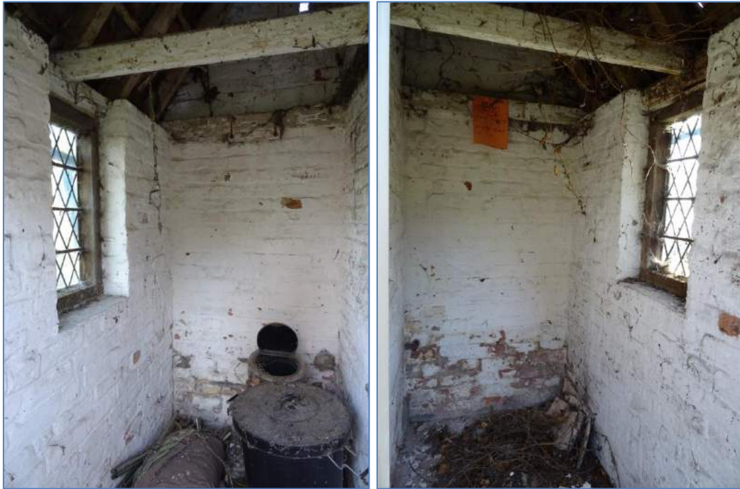
Plate 9 & 10: General views of the interior of the Earth Closets
