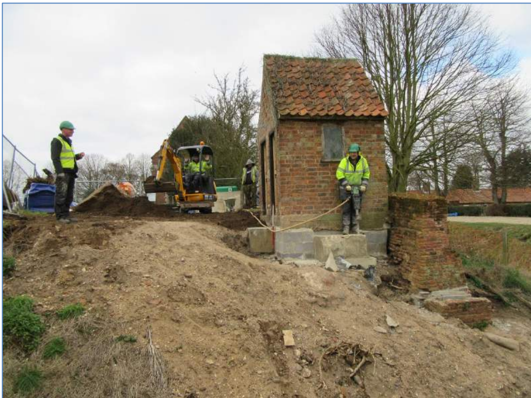
Plate 15: Working shot during final stages of archaeological supervision and recording following righting of the Earth Closet.
