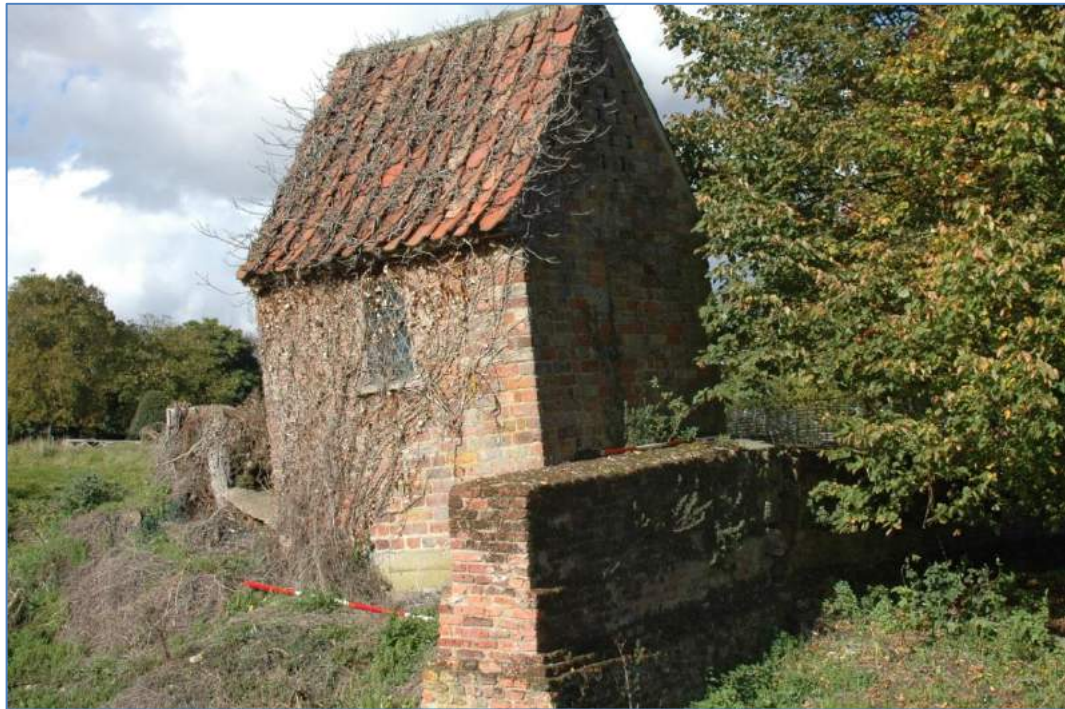
Plate 6: General view of south and east elevations and retaining wall.
