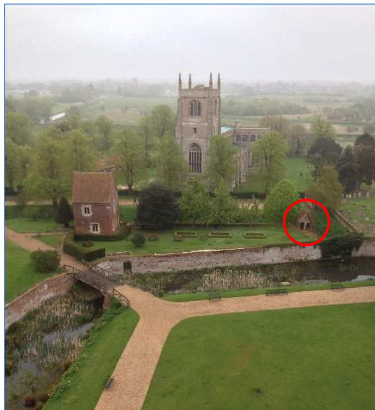
Plate 1: View towards Curzon Earth Closet (circled in red) from Tattershall Castle, positioned between the inner and outer moat.
