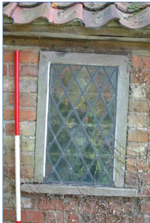
Plate 7 & 8: General view of north elevation and detail of timber framed, leaded window.
