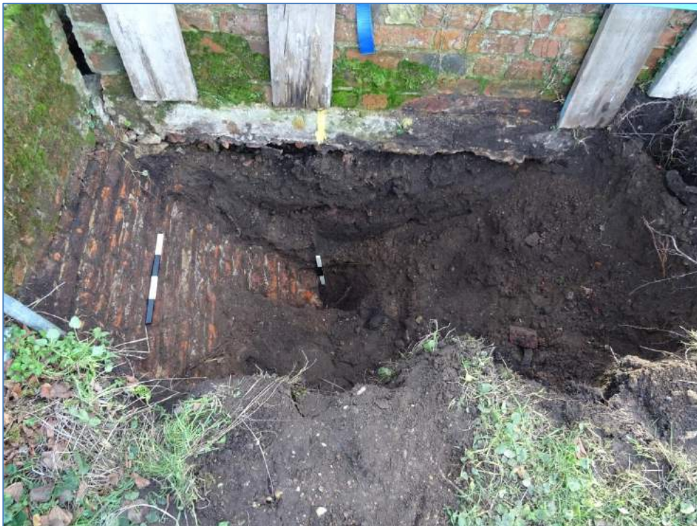
Plate 19: Trench north of Earth Closets, looking south, showing footings of retaining wall (Structure 1011 )
