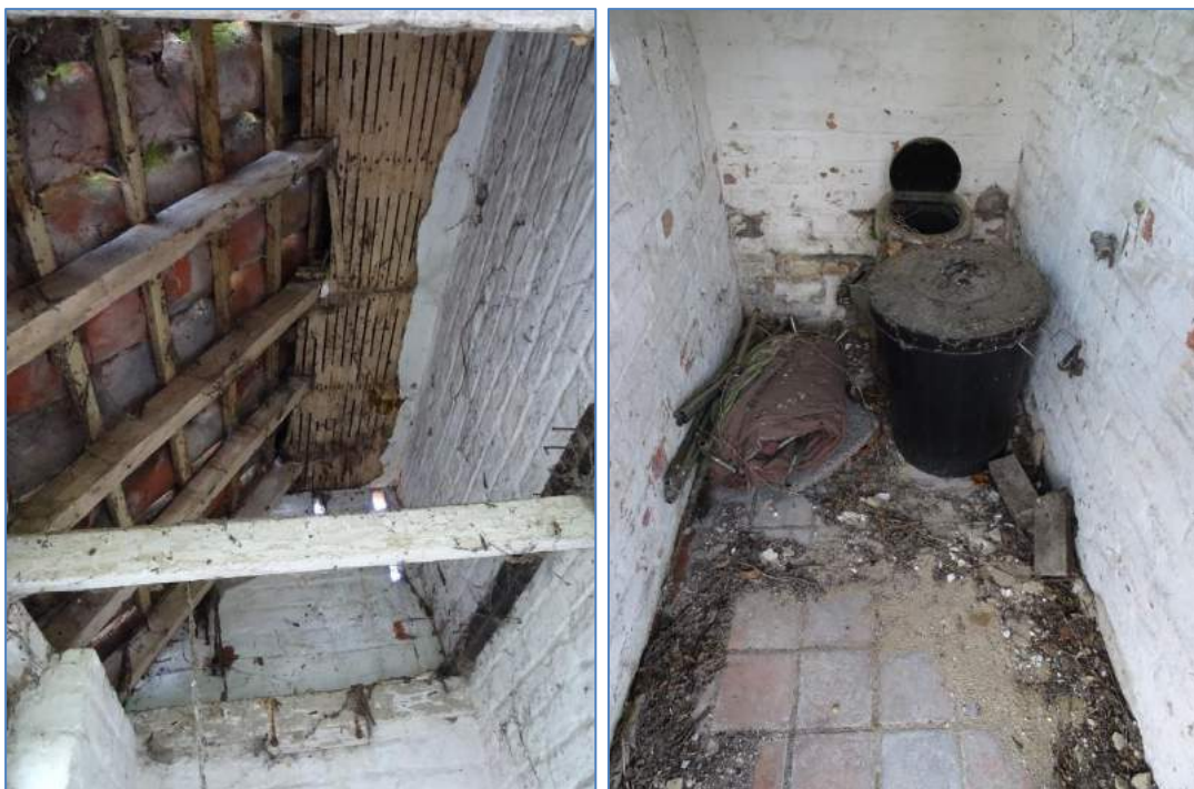
Plate 11 & 12: Detail of the ceiling and floor of the northern room of the Earth Closets.
