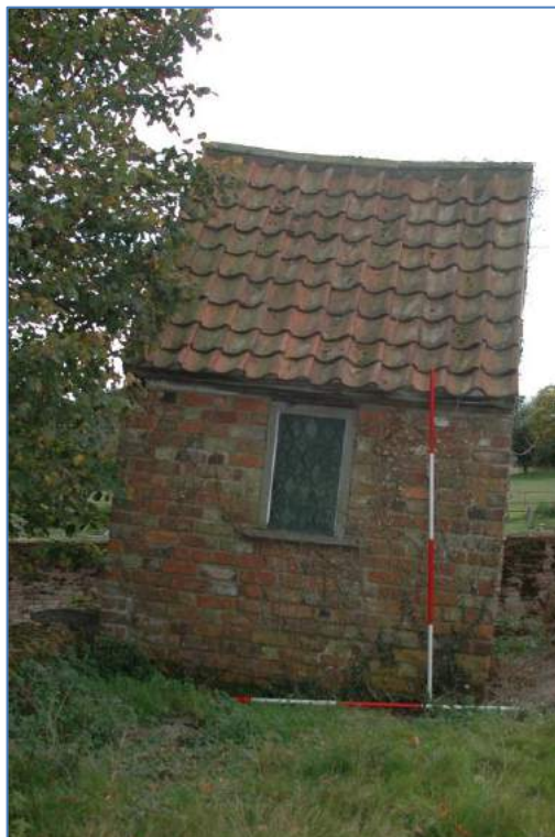
Plate 7 & 8: General view of north elevation and detail of timber framed, leaded window.
