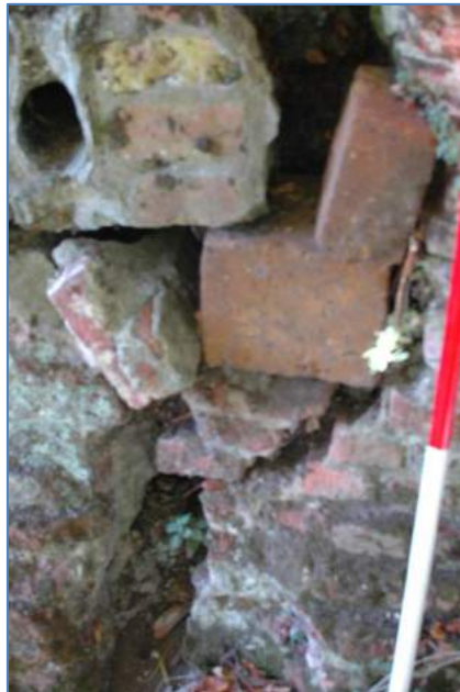
Plate 13 & 14: Detail of inserted plumbing, damage and later repairs to the retaining wall
