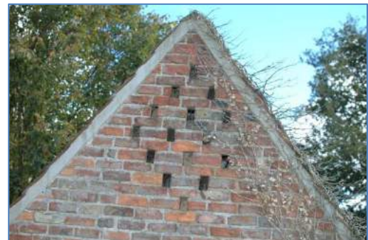
Plates 3 & 4: Detail of timber batten door and detail of ventilation in gable of west elevation
