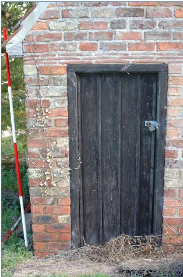
Plates 3 & 4: Detail of timber batten door and detail of ventilation in gable of west elevation
