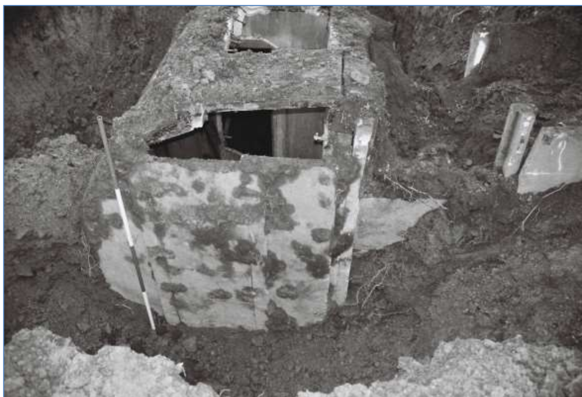
Plate 3: Detail of south-eastern end of the air raid shelter, including blocked entrance leading from access point (1.33)
