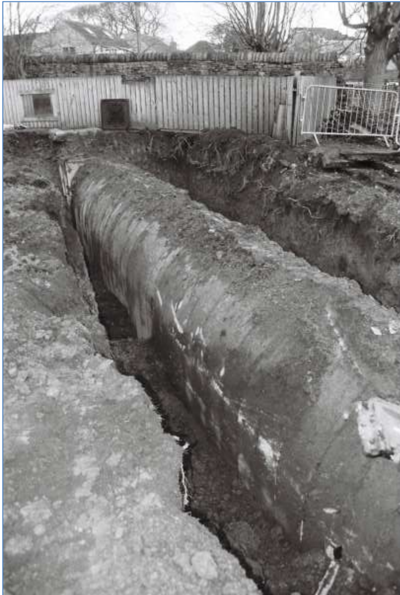
Plate 1: View facing northwest along south side of Tunnel B (1.28)
