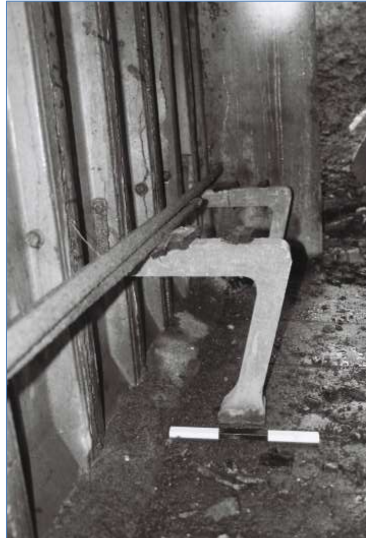
Plate 8: Detail of steel bench bracket (1.14)
