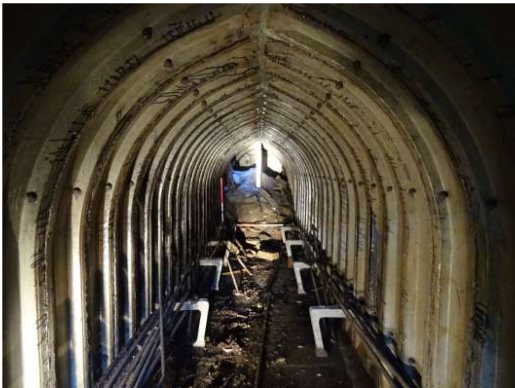
Plate 5: View facing northwest, along Tunnel B (Digital 1:19)
