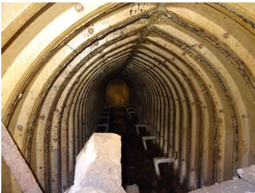
Plate 10: View along Tunnel A (Digital)
