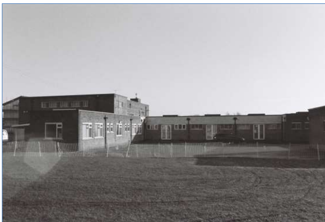
Plate 2: General view of west elevation, including view of the Children's entrance to the former cloakrooms (Film 1.6)
