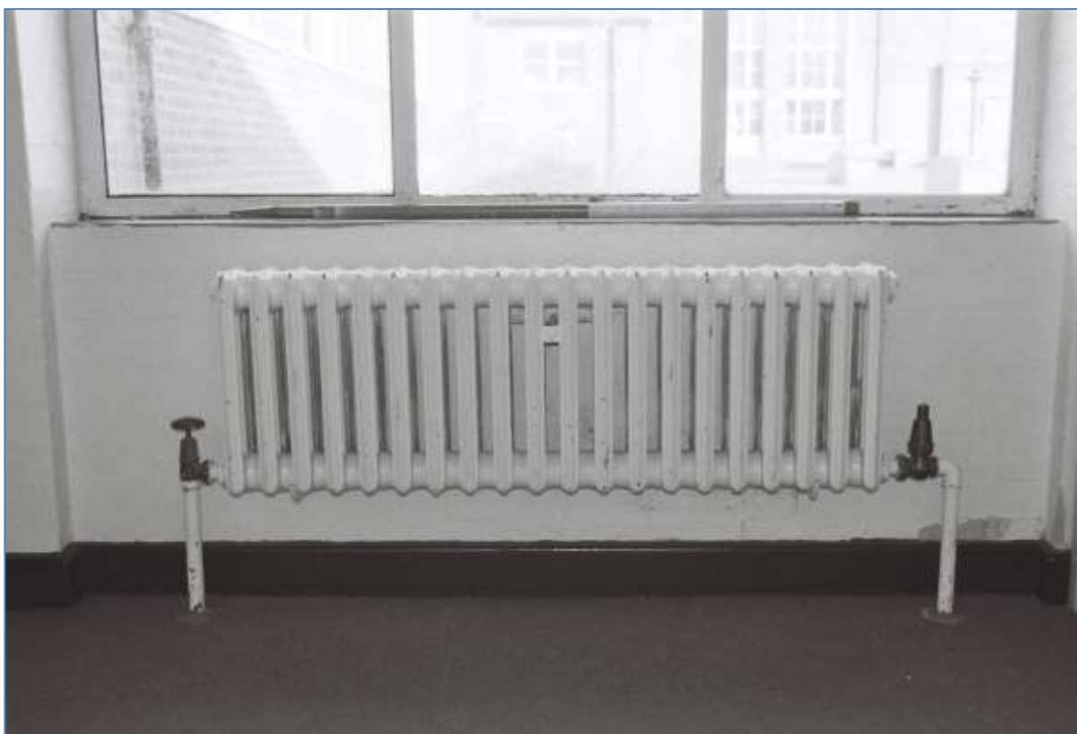
Plate 23: Detail of original radiator (Film 1.19)
