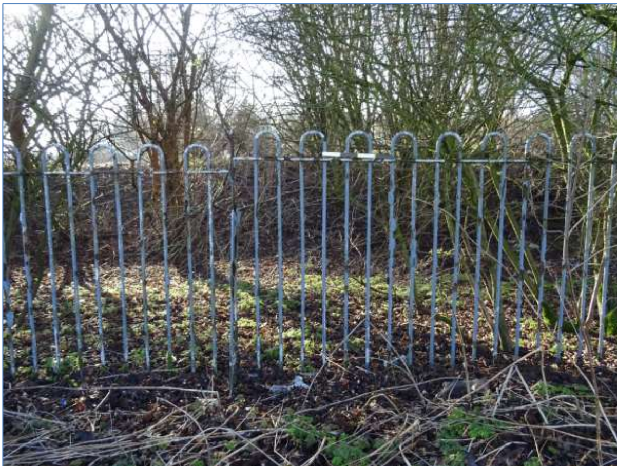
Plate 5: Detail of original school boundary fence (Digital)
