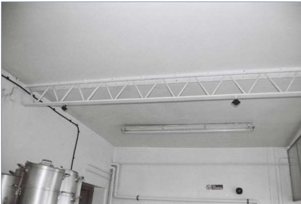
Plate 12: General view of the welded lateral truss in room G7 (Film 1.28)
