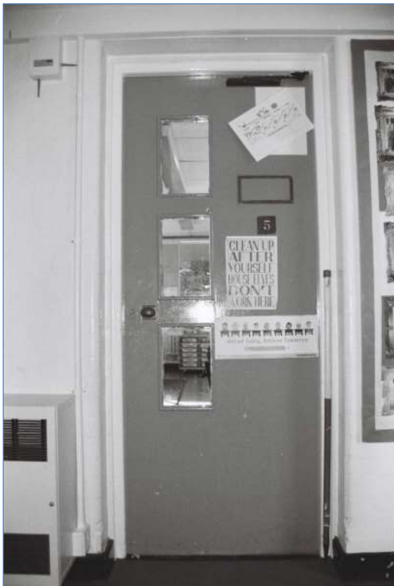
Plate 20: Detail of original classroom door, note handle, classroom number and name card slot (Film 1.21)
