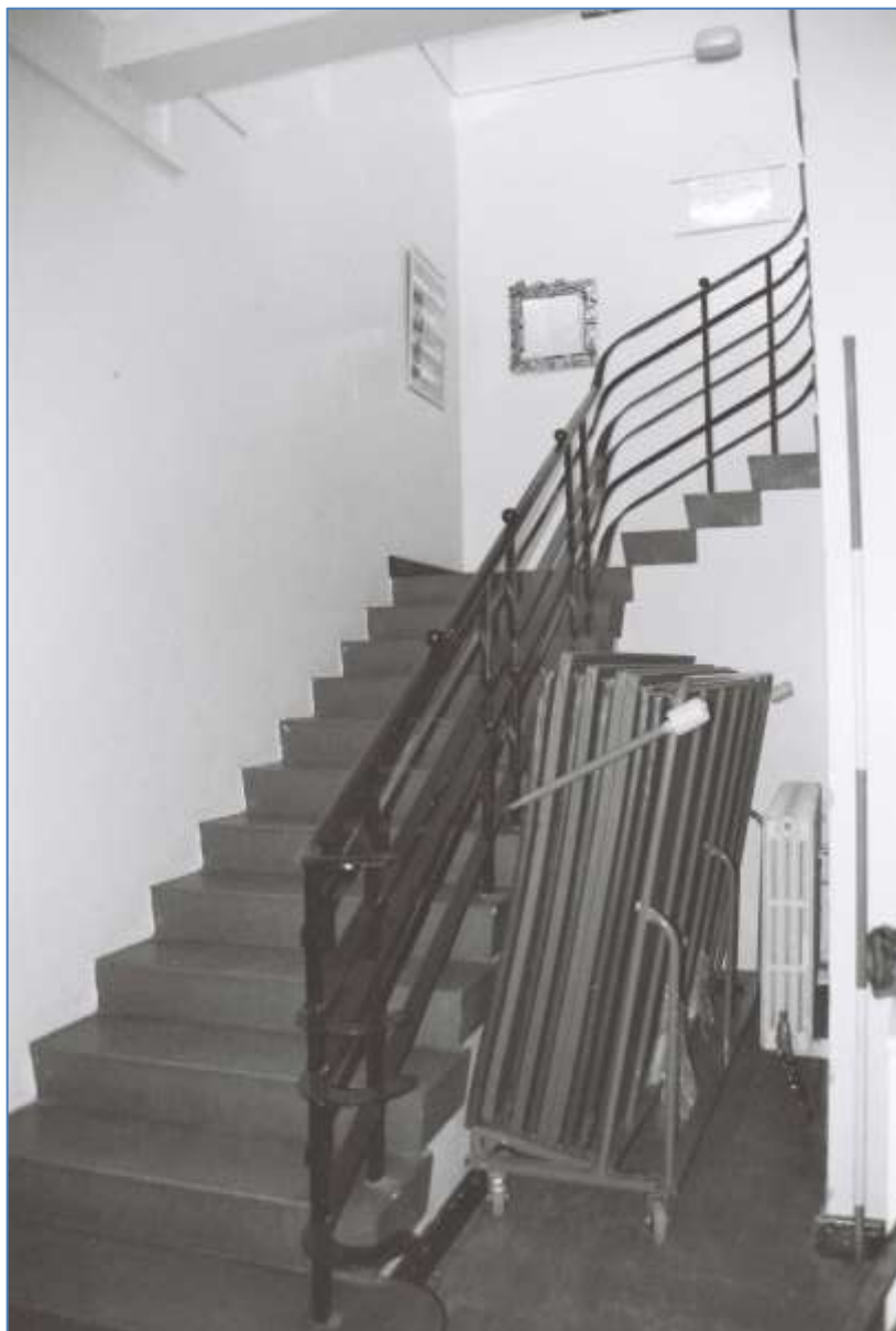
Plate 27: Detail of original staircase and hand rail (Film 1. 32)
