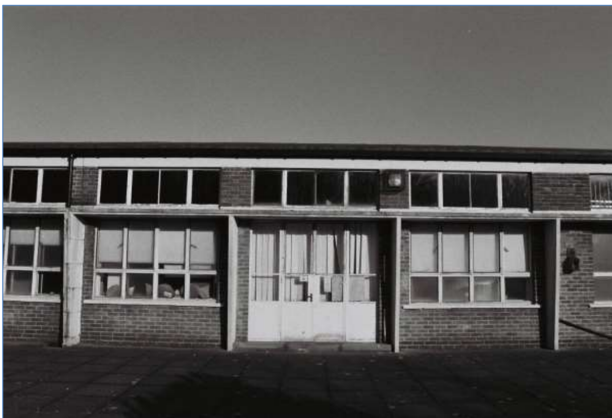
Plate 4: General view of south facing elevation and concrete flagged terrace (Film 1.5)
