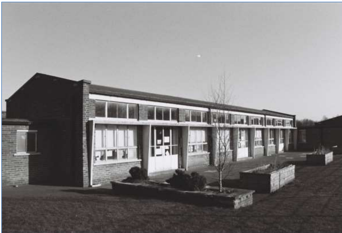
Plate 3: General view of south facing elevation and concrete flagged terrace (Film 1.5)
