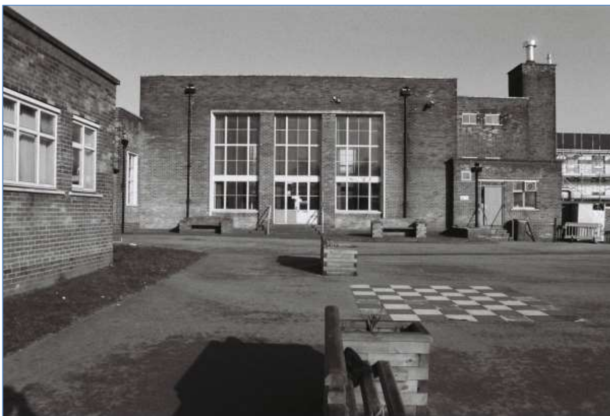
Plate 7: Detail of assembly hall windows, chimney and kitchen block (Film 1.3)
