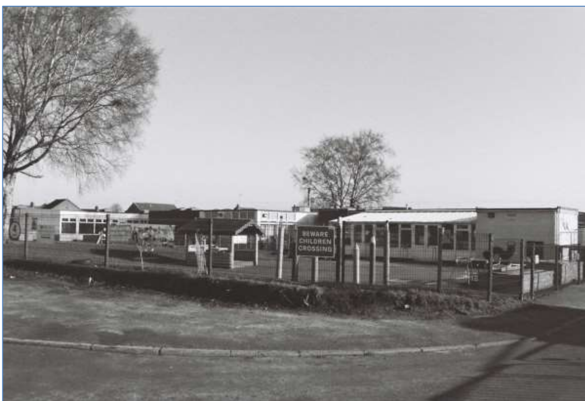
Plate 29: General view of Building 2, including the later 1980s and 1990s extension (Film 1.8)
