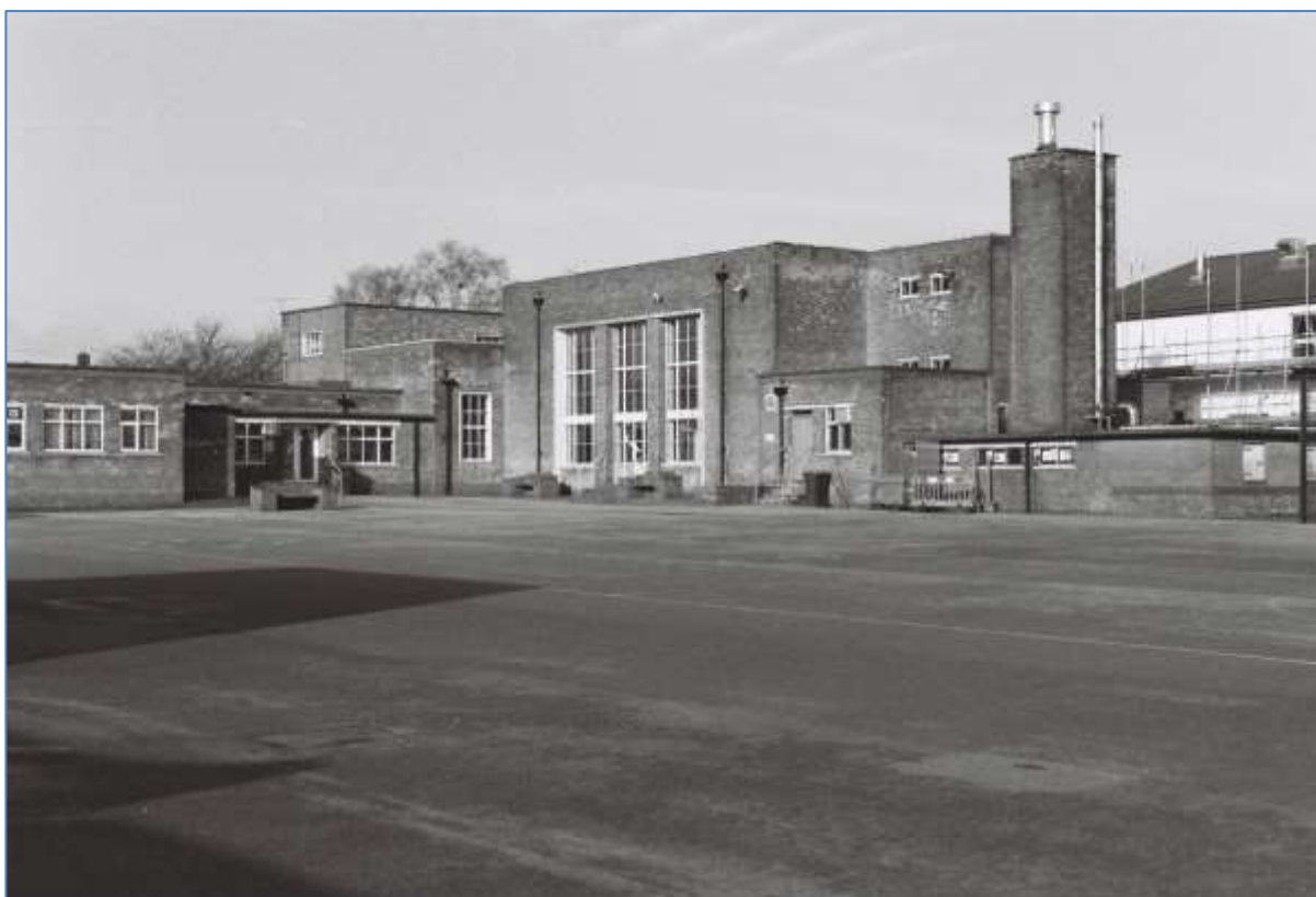
Plate 8: General view of assembly hall, kitchen block, chimney, boiler room and coal store (Film 1.1)
