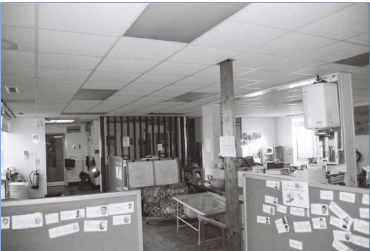
Plate 31: General view of open plan classroom in the 1980s extension of Building 2, note use of screens (Film 1.14)
