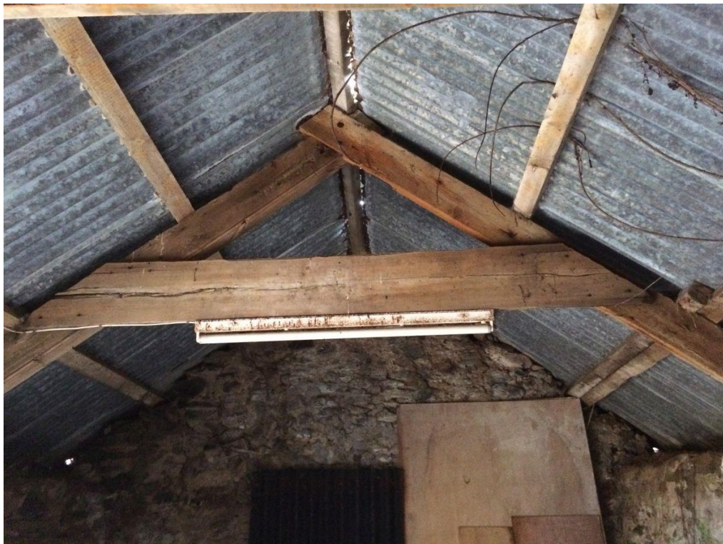
Plate 2: Detail of internal roof structure
