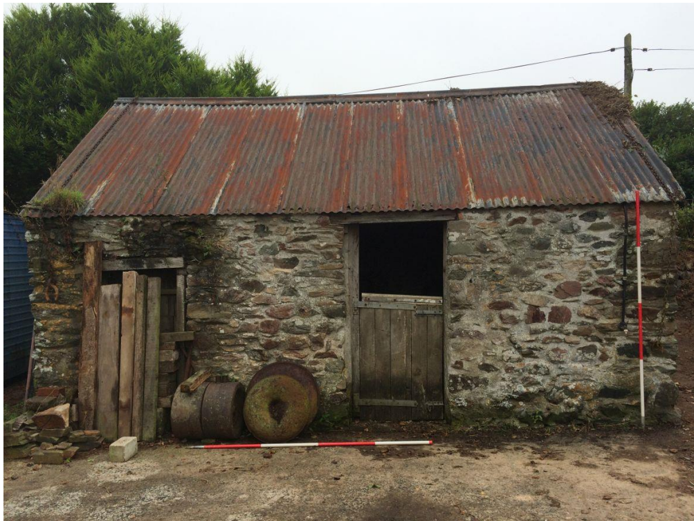
Plate 1: Eastern façade of stone barn. Scales 2 m
