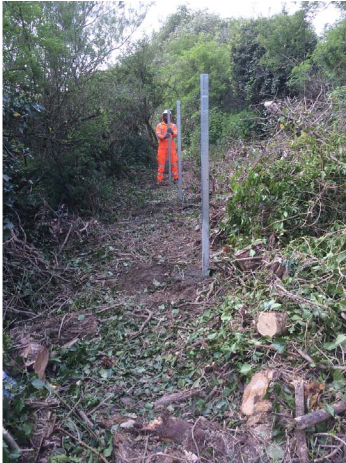
Plate 1: General shot looking southwest along the line of new fence
