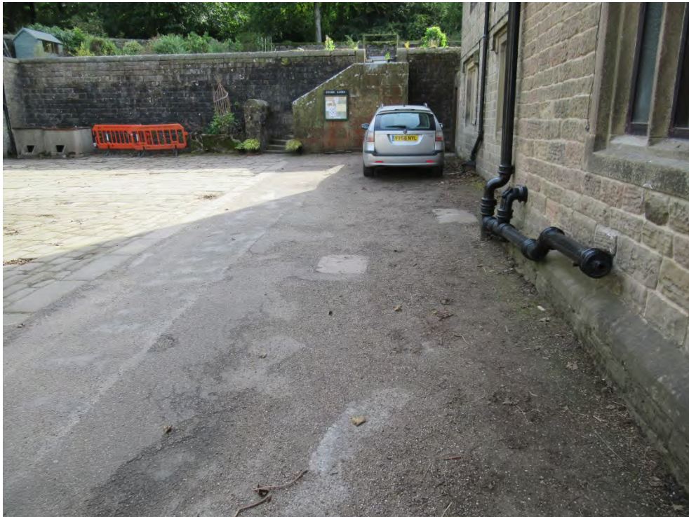
Plate 2: View across south of courtyard with Longshaw Lodge and retaining wall for kitchen garden beyond
