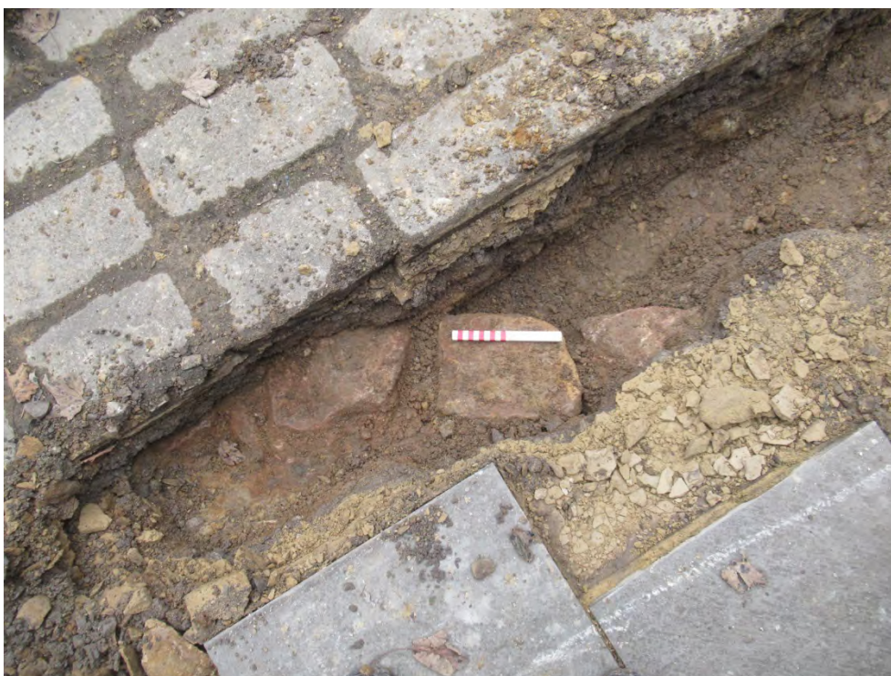
Plate 6: Probable drainage structure (106) from the west
