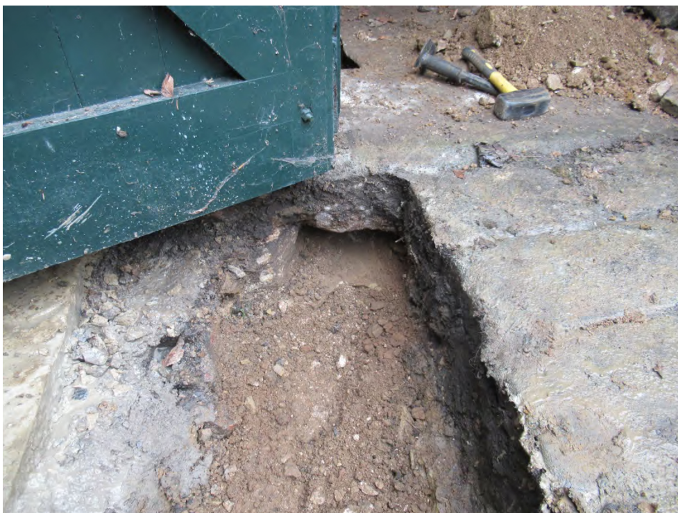
Plate 5: Detail of foundations (109) for carriage house from the southwest
