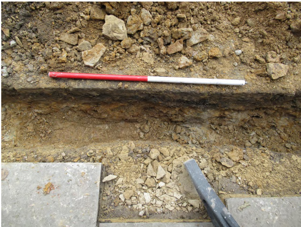
Plate 4: Representative section of the northern section of the groundworks
