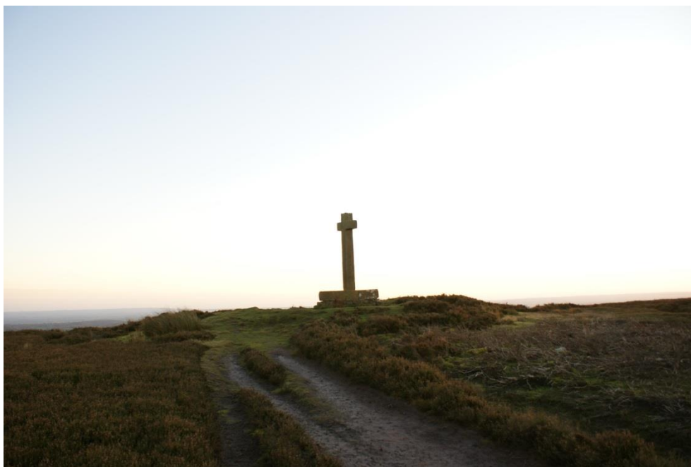
Plate 5: The northern side of the mound before remedial works (November 2017)
