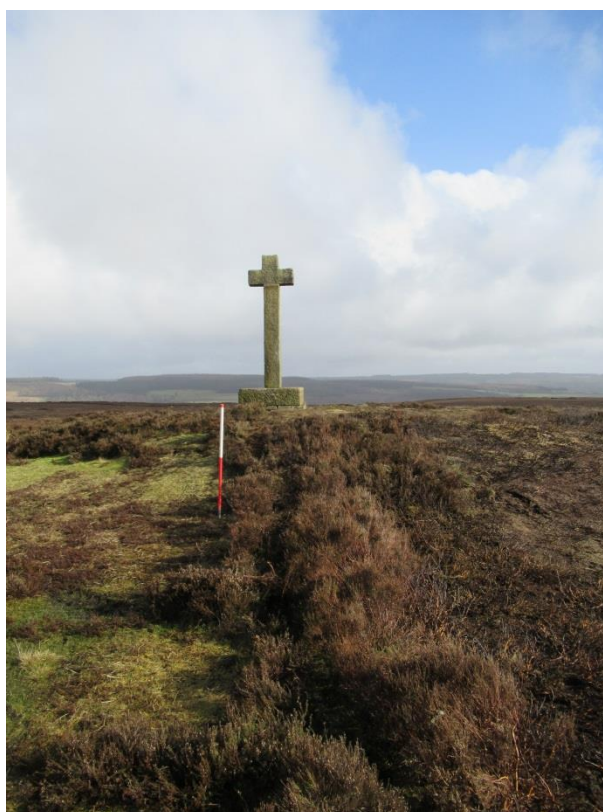
Plate 12: A view of the western track after remedial work (February 2018)
