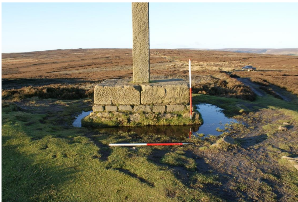
Plate 13: A view of the waterlogged hollow surrounding the monument before remedial work (November 2017)
