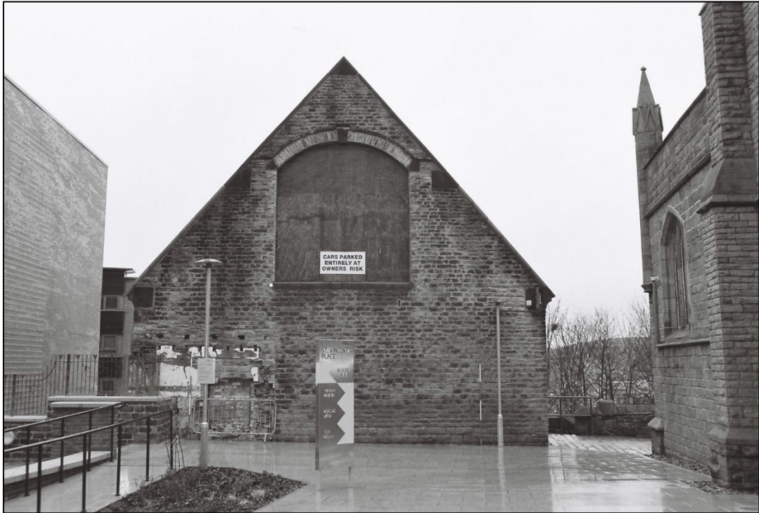
Plate 9: General view of the southern elevation (Film/Frame 3.4)
