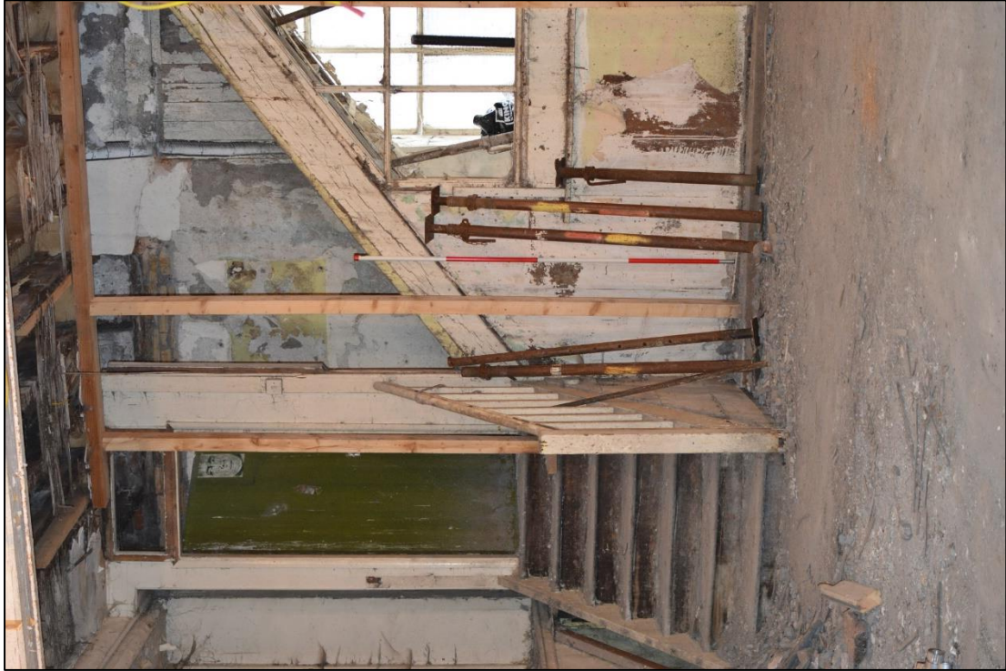
Plate 19: Detail of inserted timber staircase in Room G2 (Digital Shot 019)
