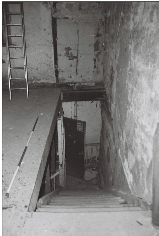
Plate 36: Detail of inserted staircase up to Room F1 (Film/Frame 2.19)
