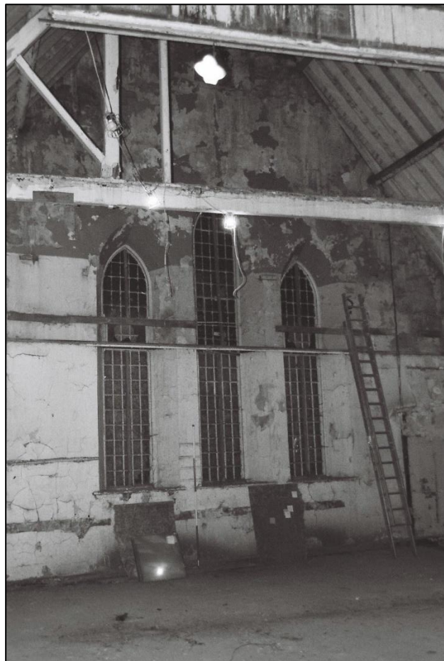
Plate 42: Detail of north facing windows in Room F1 (Film/Frame 2.8)
