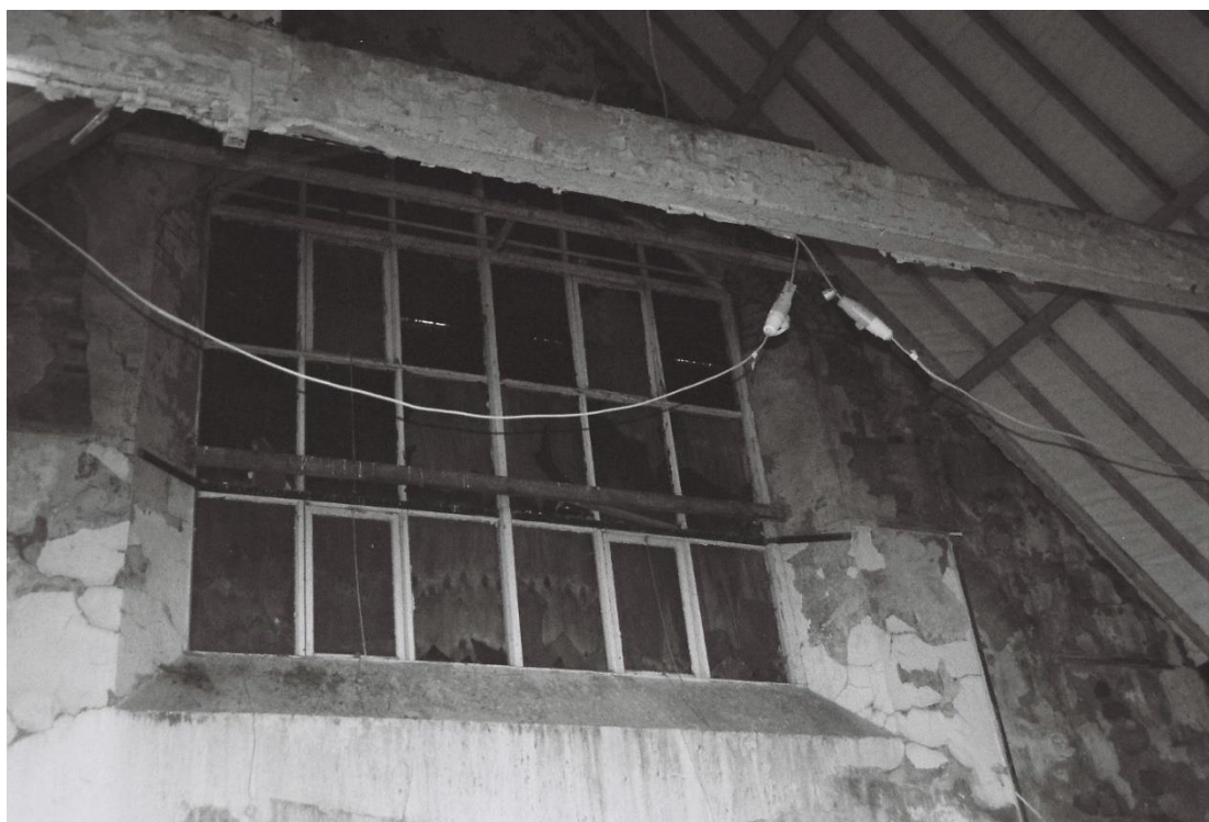
Plate 40: Detail of south facing window in Room F1 (Film/Frame 2.4).
