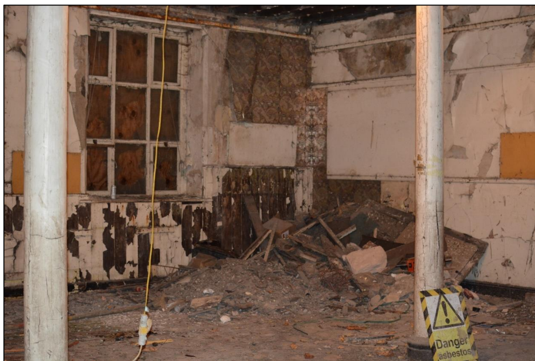
Plate 26: General view of Room G3 (Digital 034)
