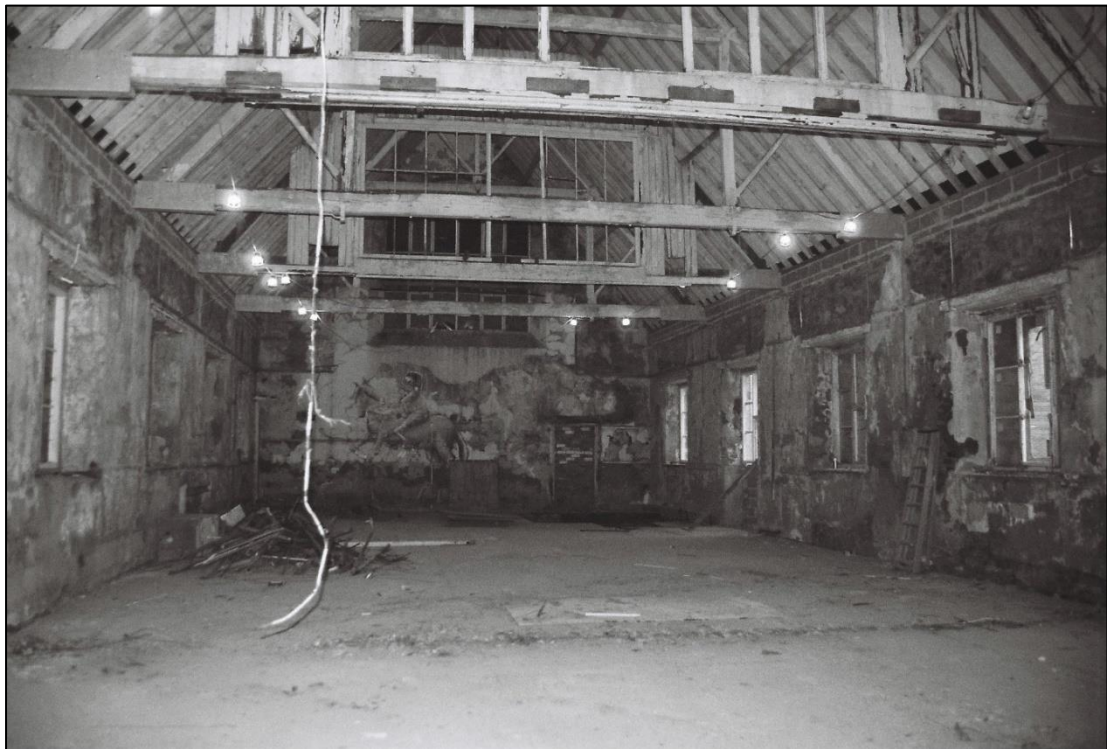
Plate 32: General view of Room F1 (Frame/Film 2.23)
