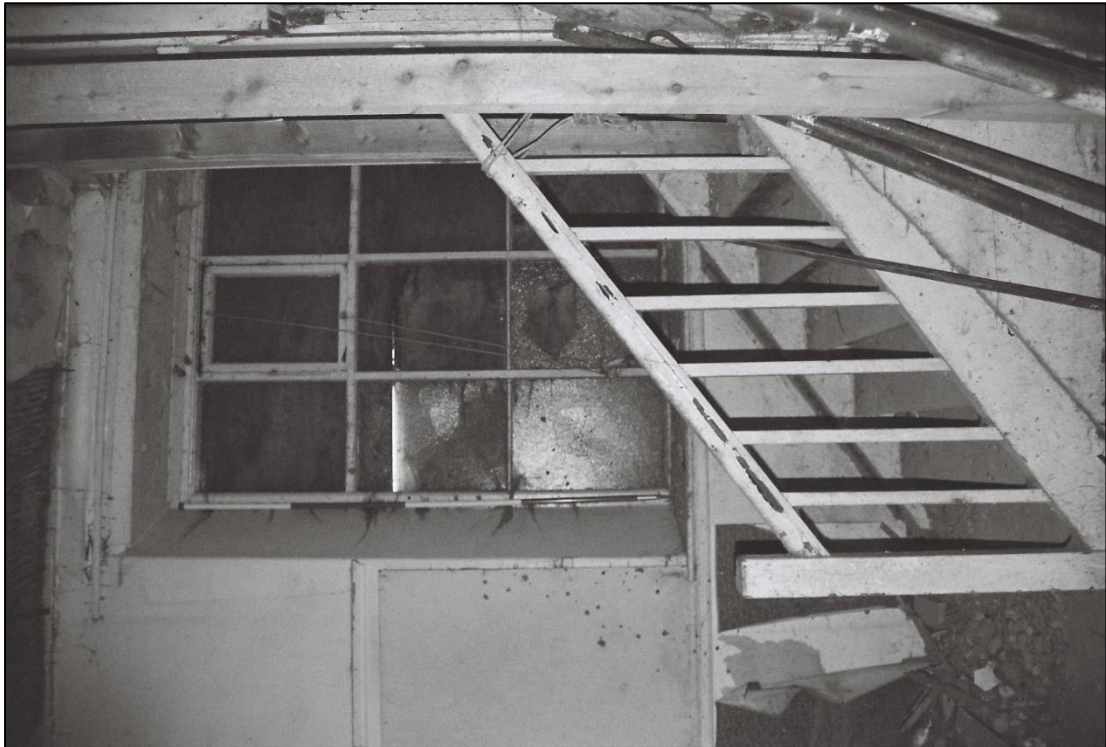
Plate 21: Detail of window in northern wall of Room G2 (Film/Frame 1.10)
