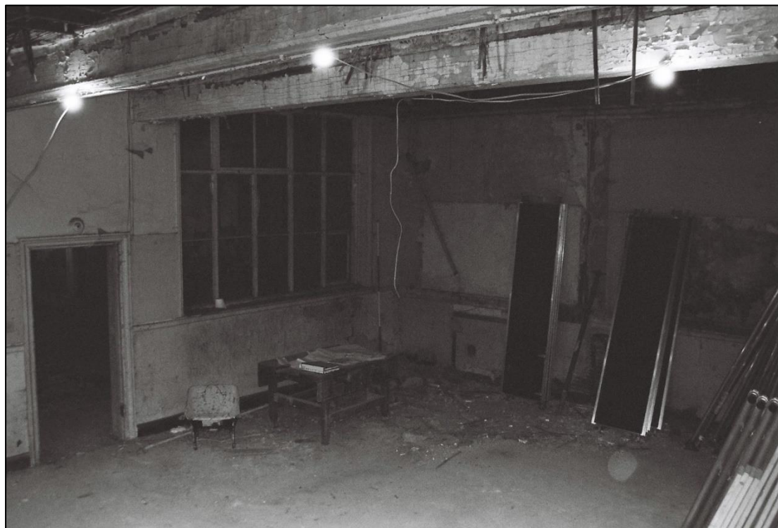
Plate 16: General view of Room G2 from inserted staircase (Film/Frame 1.27)
