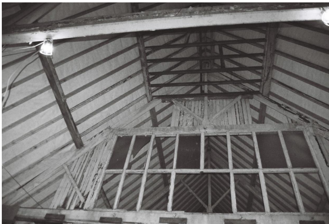
Plate 37: Detail of portioned roof truss (Film/Frame 2.10)
