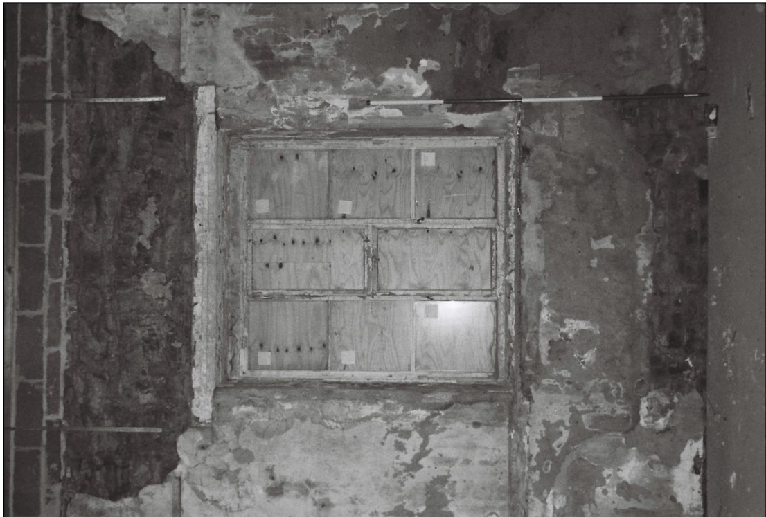
Plate 12: Detail of timber window frame (Film/Frame 2.15)
