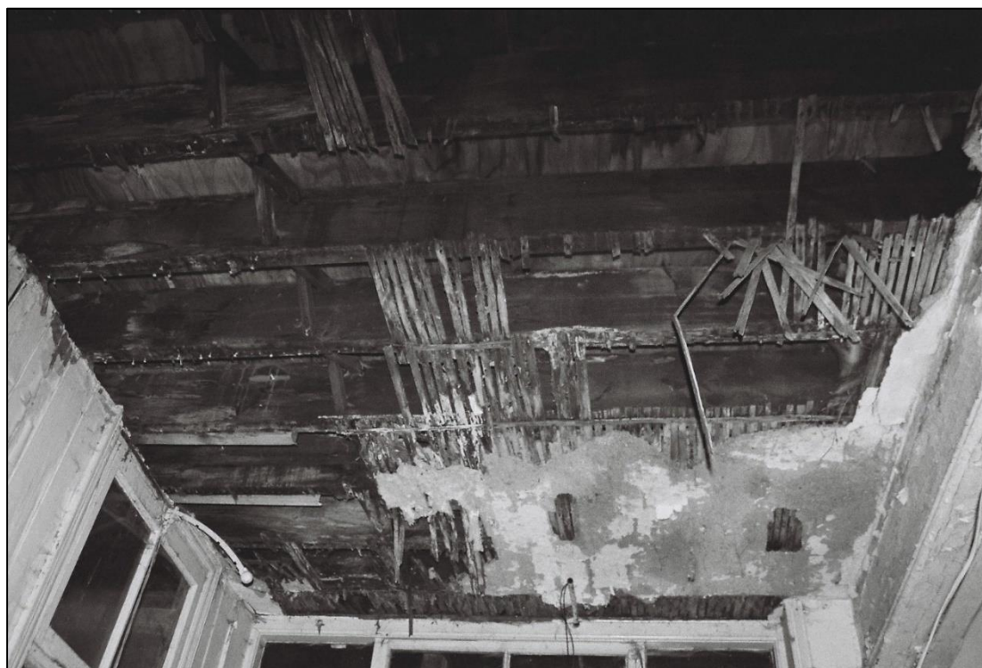
Plate 24: Detail of lath and plaster ceiling in Room G2 (Film/Frame 1.20)
