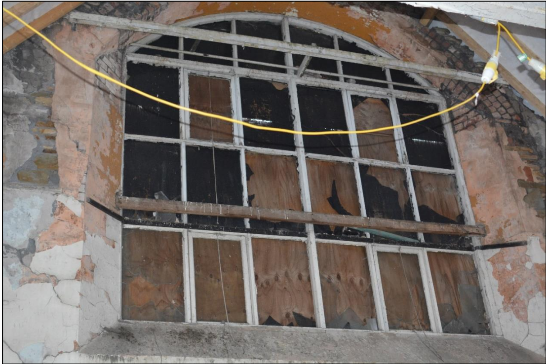
Plate 41: Detail of south facing window in Room F1 (Digital Shot 079)
