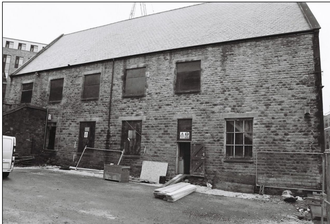
Plate 7: General View of the eastern elevation of the building (Film 3/10)
