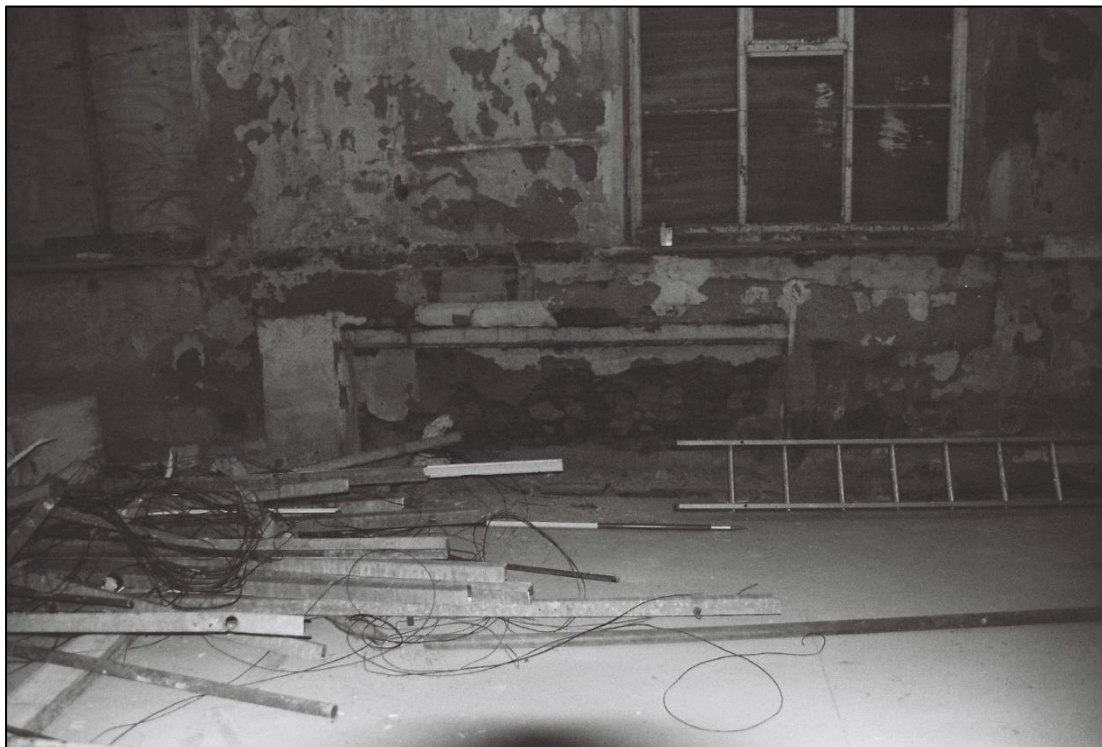
Plate 39: Detail of recess and RSJ, Room F1 (Film/Frame 2.1)
