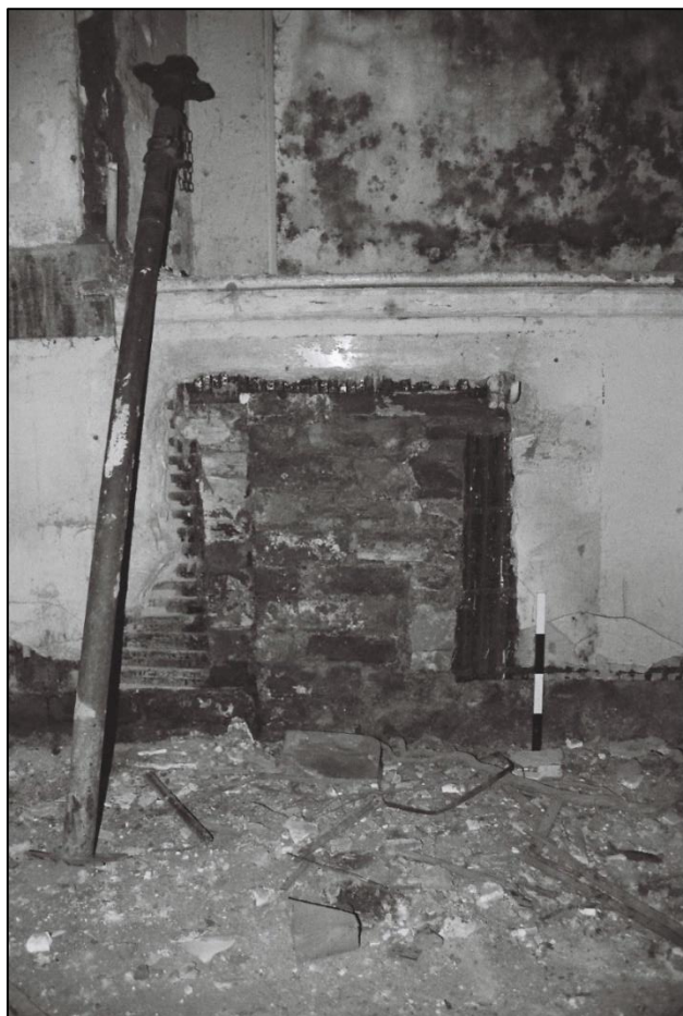
Plate 23: Detail of straight joint in Room G2 (Film/Frame 3.14)
