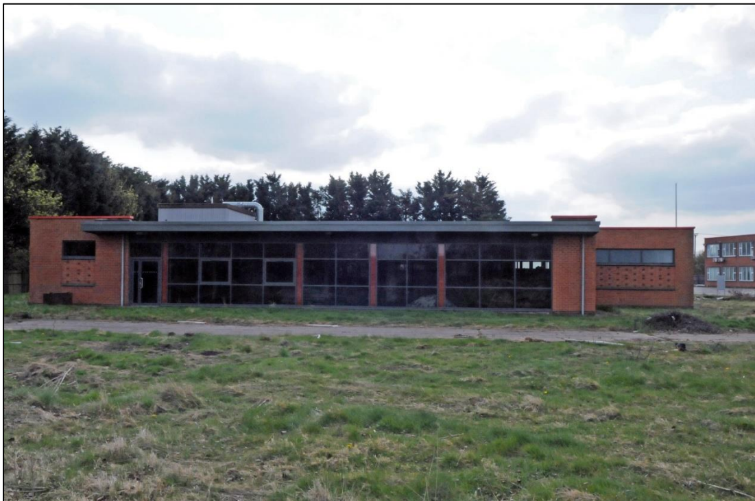
Plate 2: General view of north facing elevation of Building 1 (image0060).
