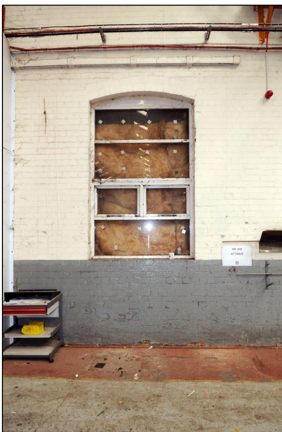
Plate 26: Detail of modern UPVC window (image 0005).
