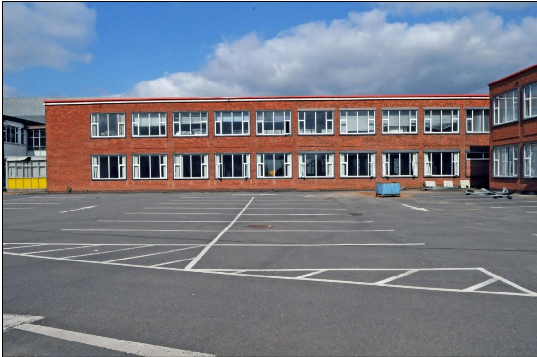
Plate 11: General view of the south facing elevation of Building 2 (image 0094).
