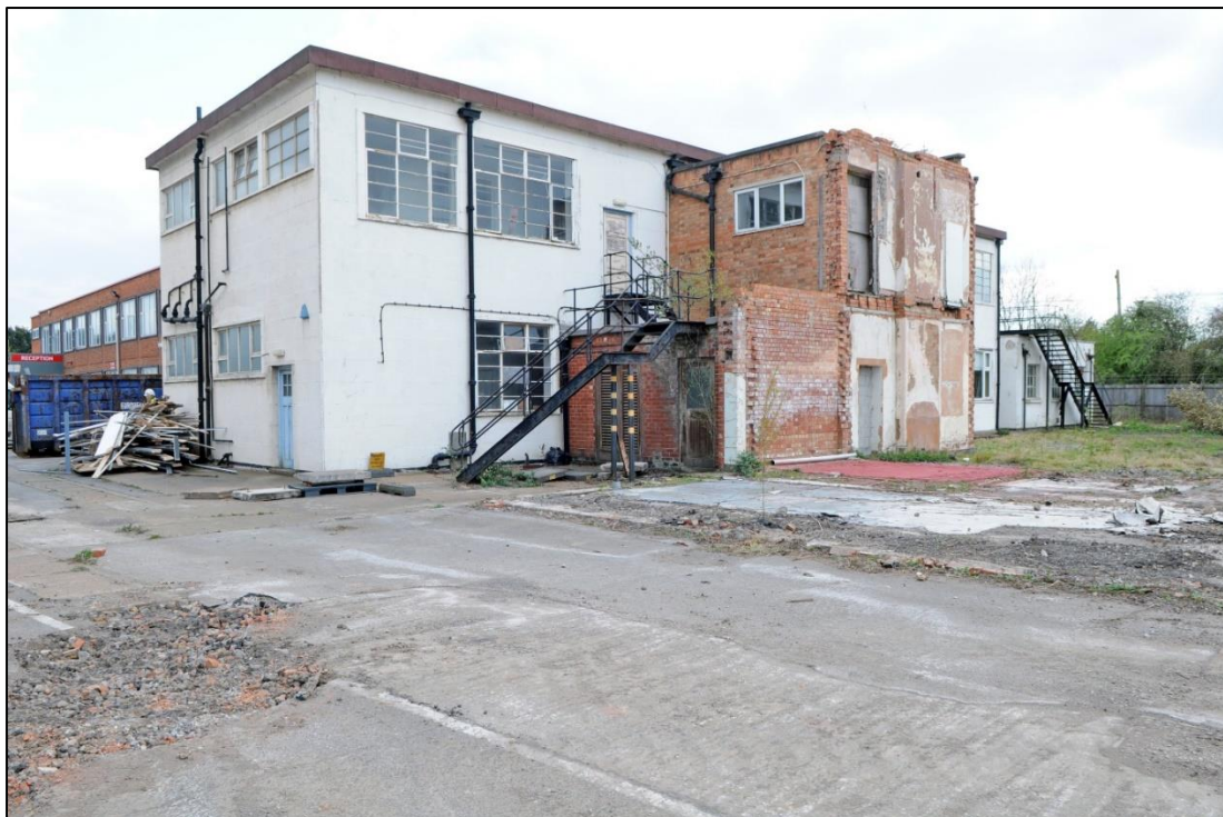
Plate 9: General view of the west facing elevation of Building 2 (image 0078).
