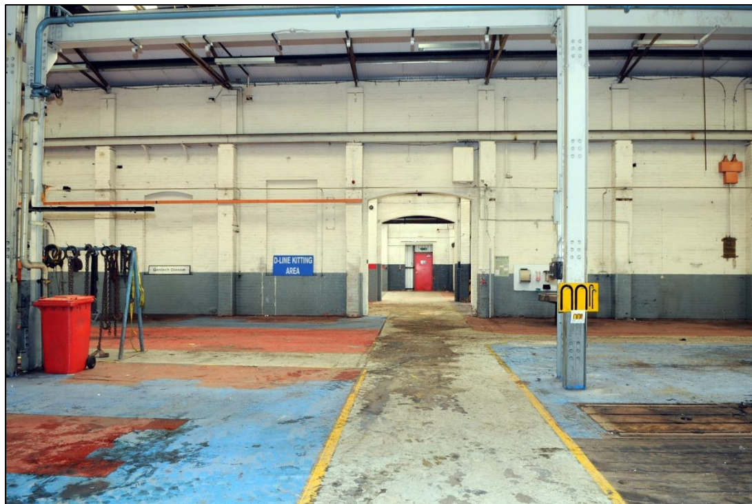
Plate 25: Detail of eastern wall of western range of Building 4 (image 0008).
