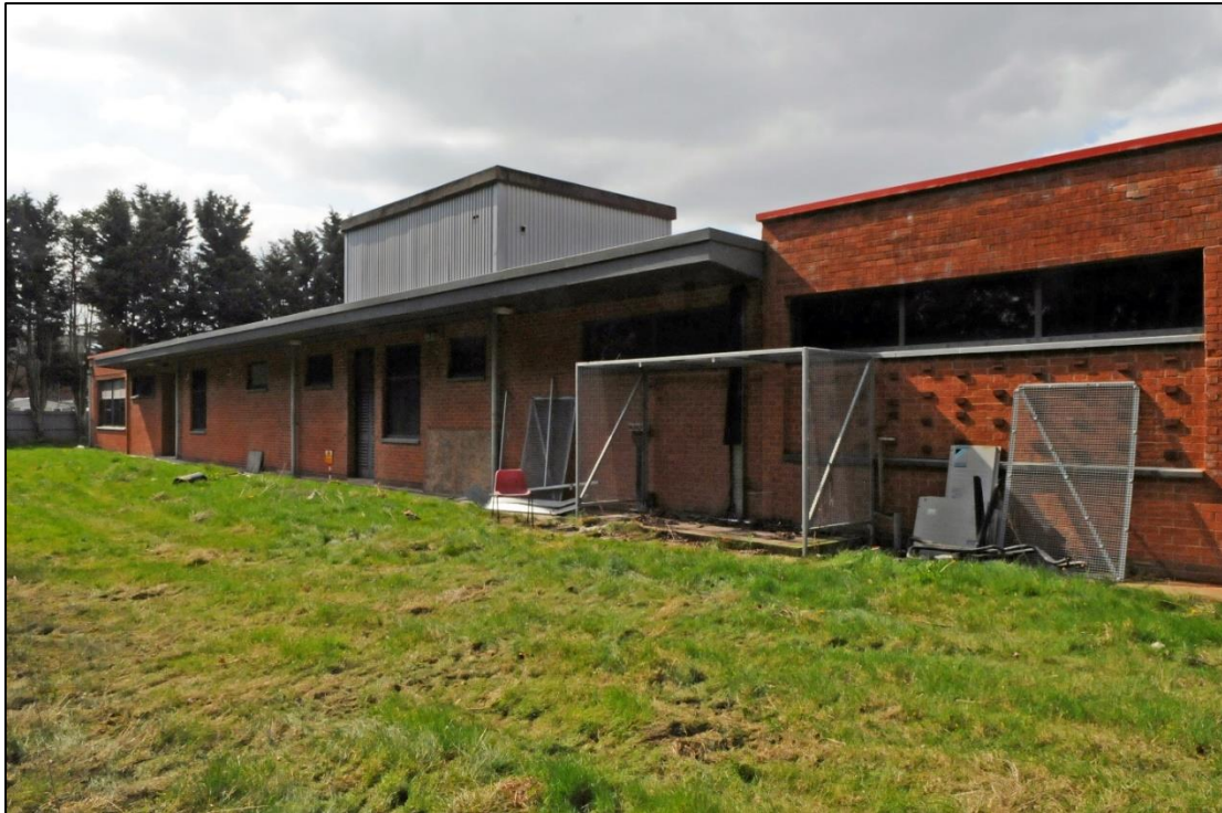
Plate 3: General view of the north facing elevation of Building 1 (image 0061).
