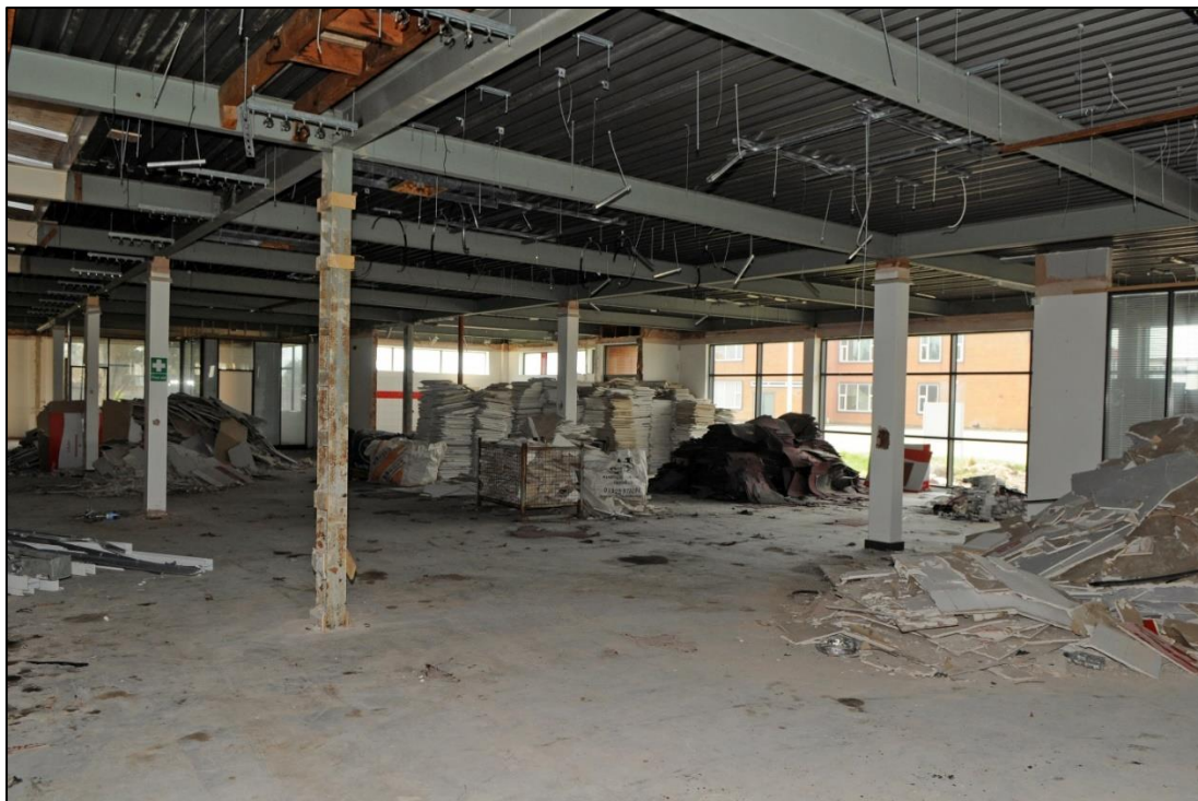
Plate 7: General view of the interior of Building 1 , facing south west (image 0073).
