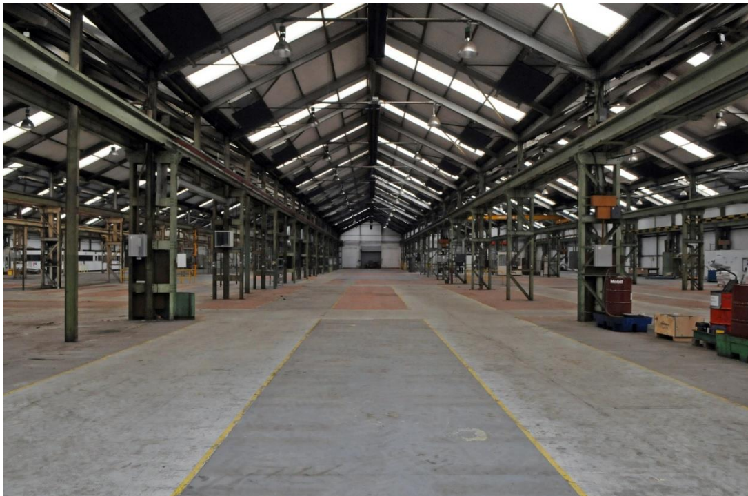
Plate 36: General view of eastern range, facing north (image 0020)
