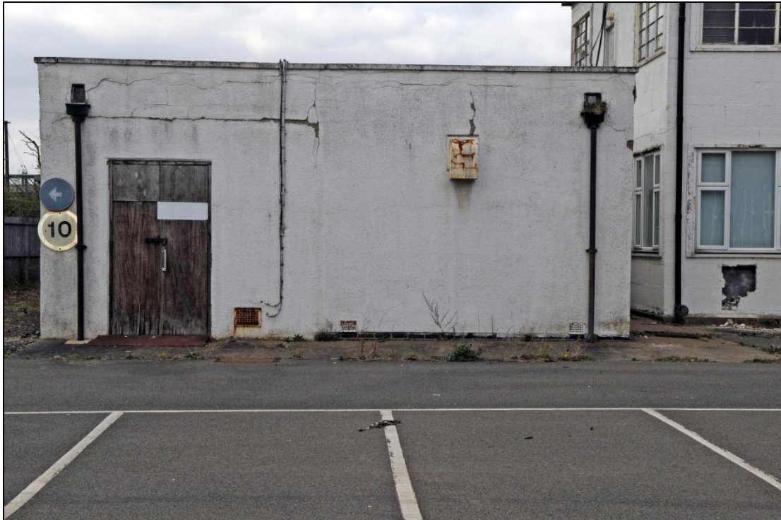
Plate 19: General view of the east facing elevation of Building 3 (image 0074).
