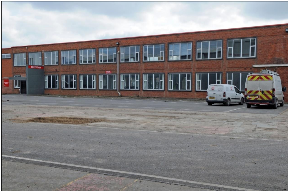
Plate 14: General view of the northern elevation of Building 2 (image 0083).
