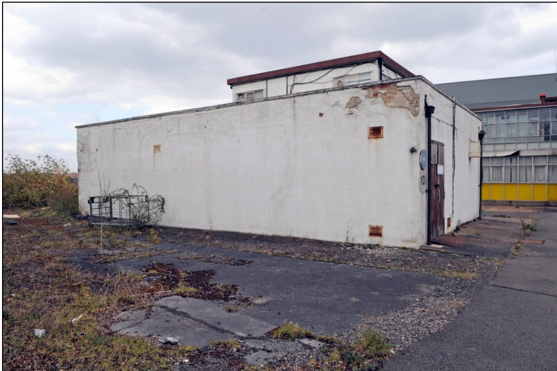
Plate 20: General view of the south facing elevation of Building 3 (image 0075).
