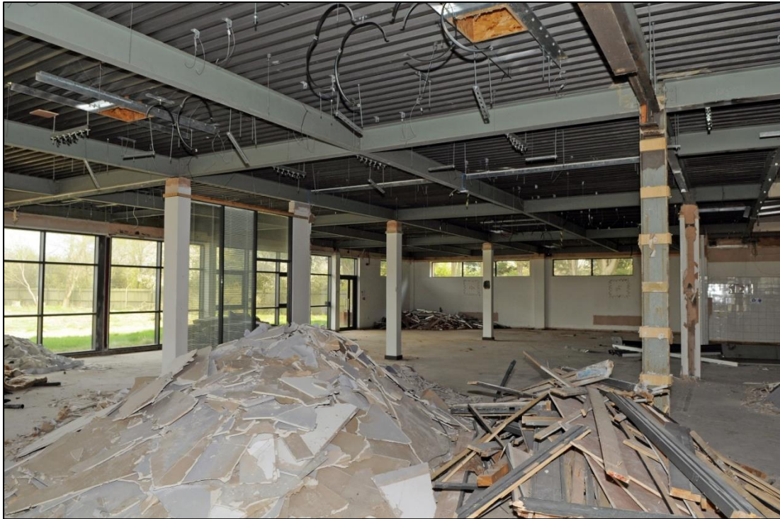
Plate 5: General view of the interior of Building 1 facing north west (image 0071).
