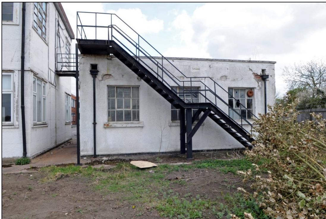
Plate 21: General view of the west facing elevation of Building 3 (image 0076).
