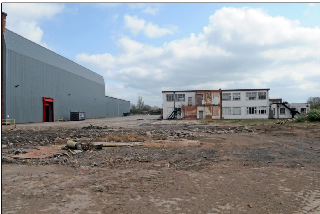
Plate 10: General view of west elevation of Building 2 (image 0045).
