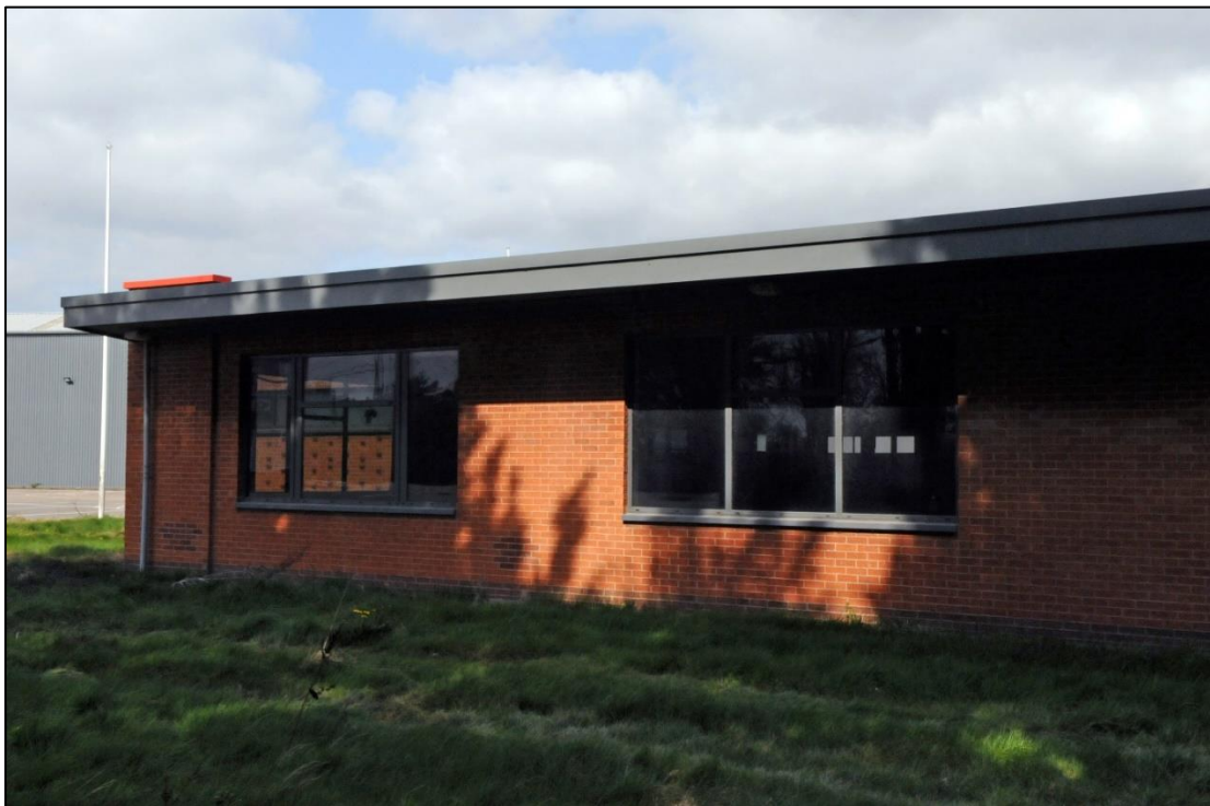
Plate 4: General view of south facing elevation of Building 1 (image 0064).
