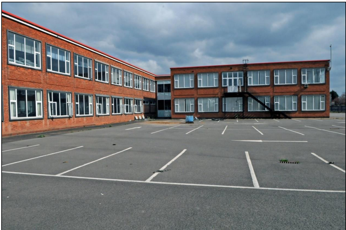
Plate 12: General view of the west facing elevation of the western block of Building 2 (image 0095).
