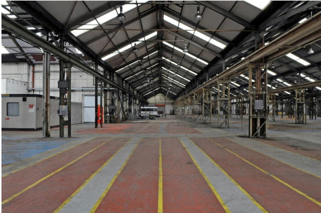
Plate 35: General view of eastern range, facing north (image 0017)
