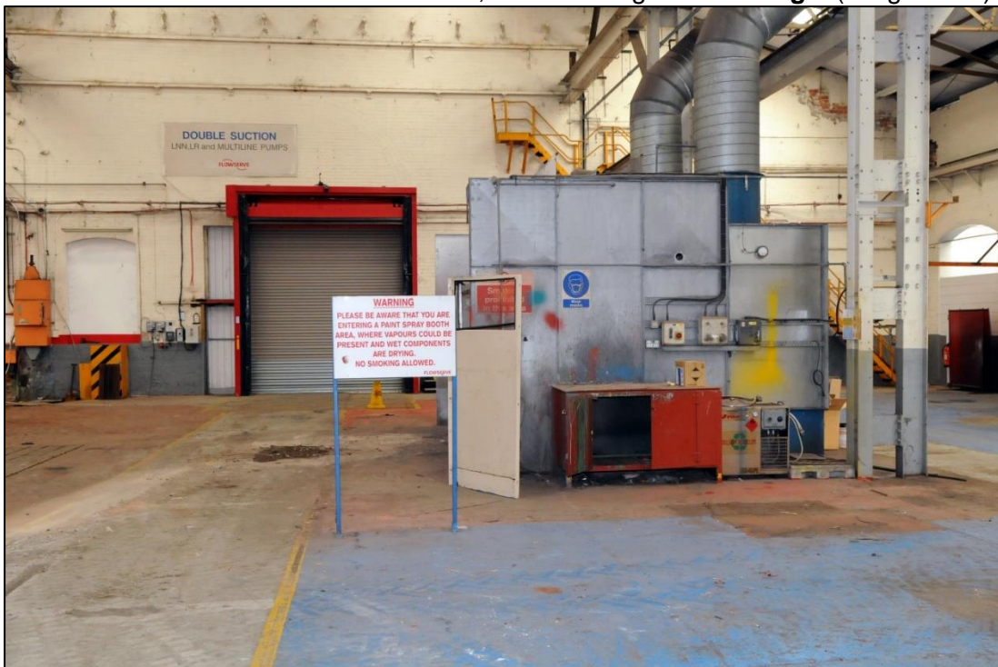
Plate 30: Detail of paint spraying station, Western range of Building 4 (image 0030).
