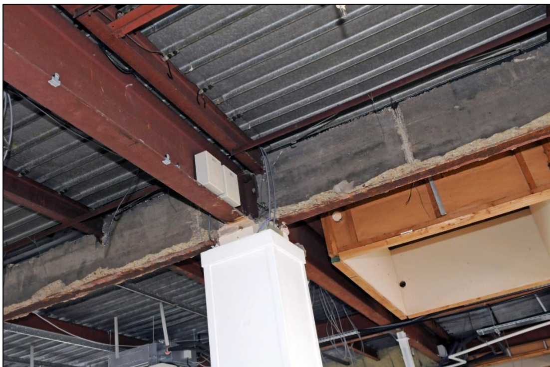
Plate 18: Detail of roof structure eastern block of Building 2 (image 0110).
