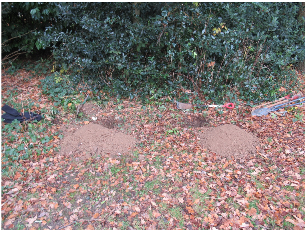
Plate 4: Sign installation pits following excavation
