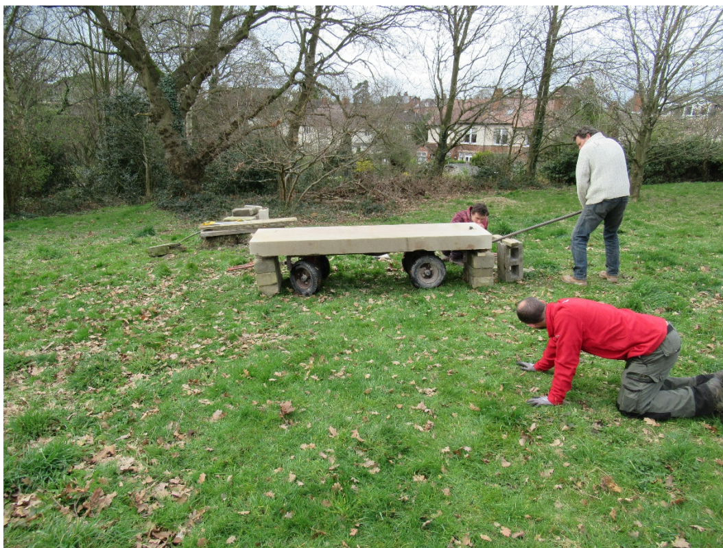
Plate 6: Working shot of stone slab being manoeuvred into place
