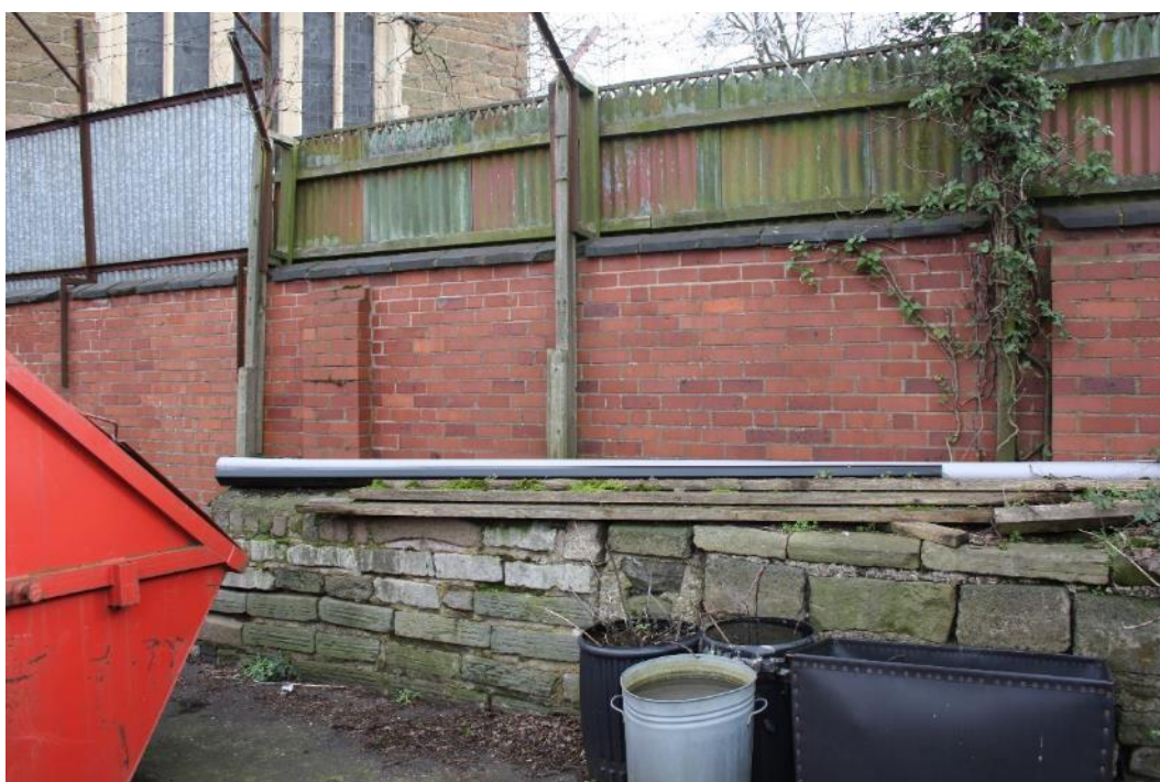
Plate 21: South western extent of boundary wall
