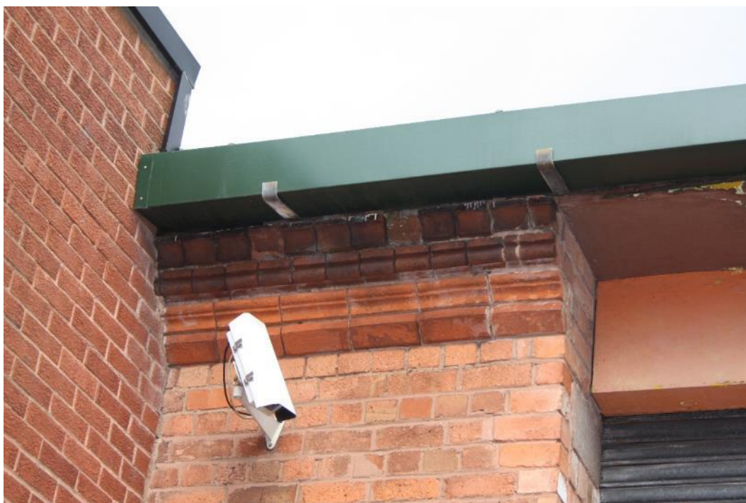
Plate 17: Sample of corbelling along the top section SW: 1
