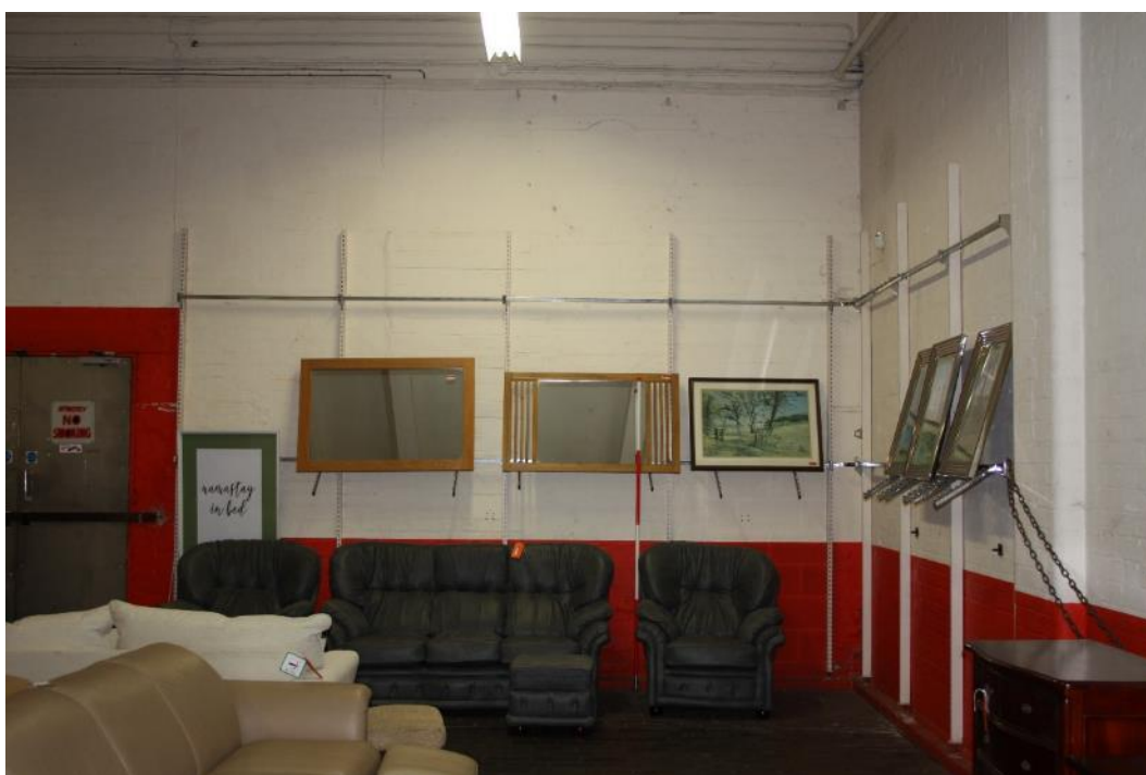
Plate 29: Blocked in openings in south west wall of Room 2
