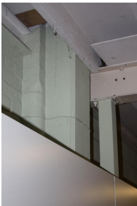
Plate 24: Sample of the chamfering detail on the columns along the wall of Room 1
