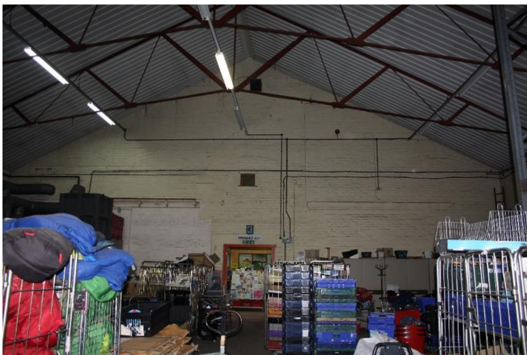
Plate 38: North west wall of Room 4
