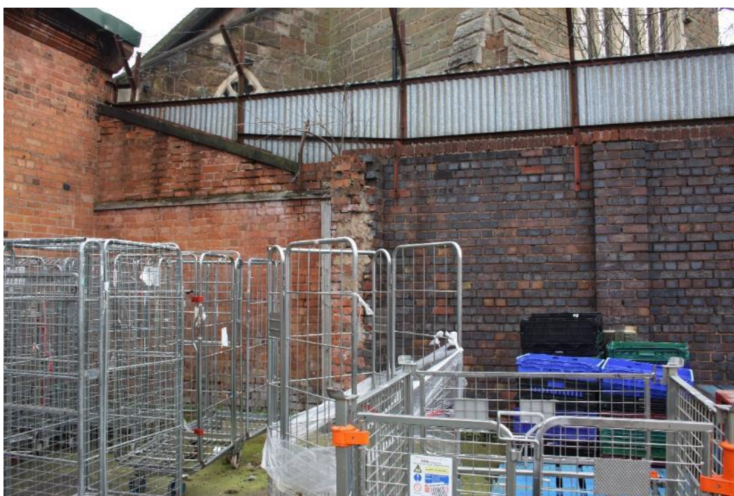
Plate 19: North eastern extent of boundary wall
