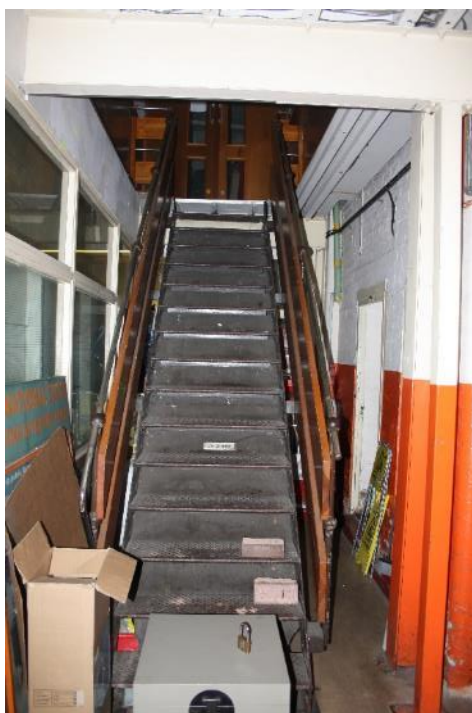
Plate 27: Stairs and doors in the north west wall of Room 1b
