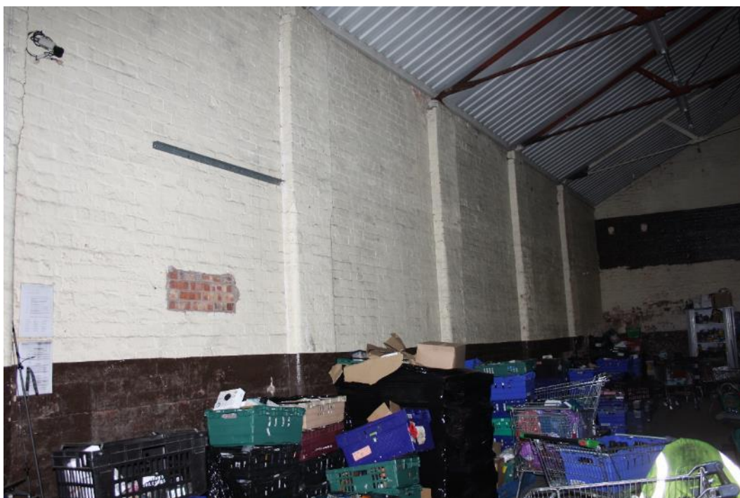
Plate 40: South eastern extent of the north east wall of Room 4
