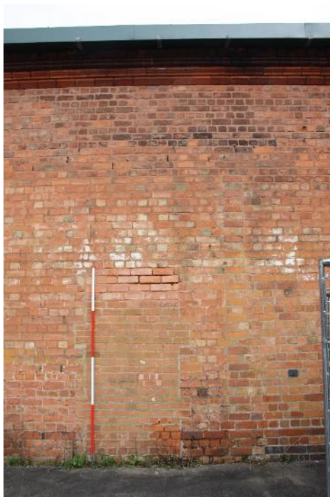
Plate 16: Blocked in doorway in centre of SW: 1
