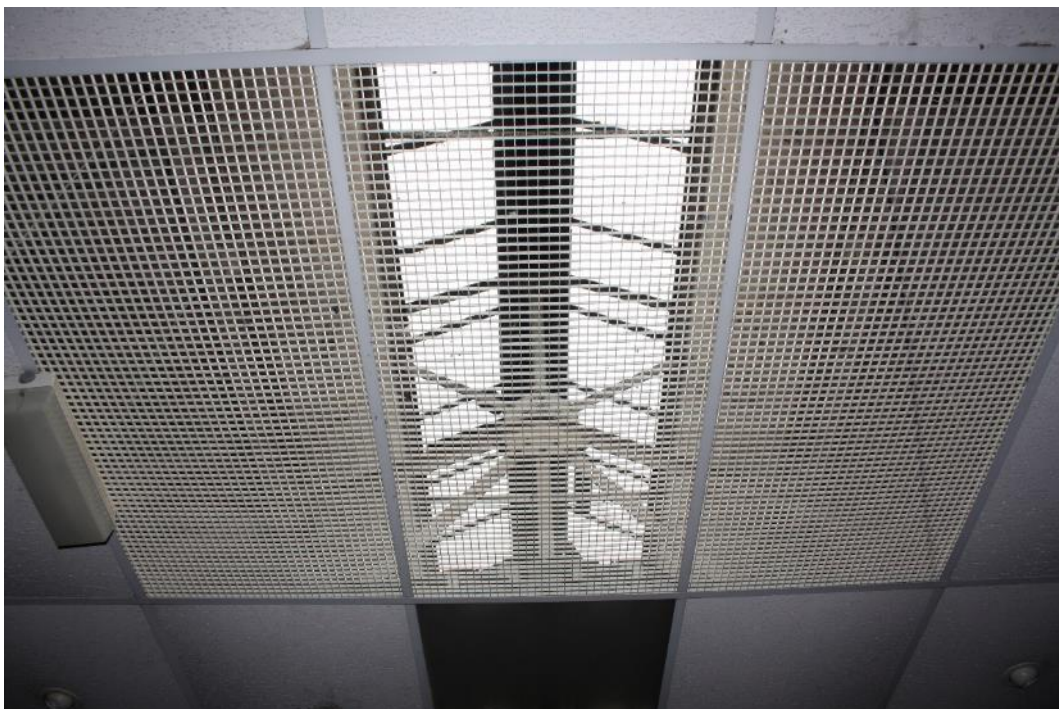
Plate 43: Sample of the roof structure of Room 6
