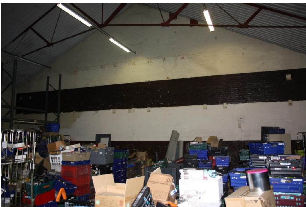
Plate 37: South east wall of Room 4
