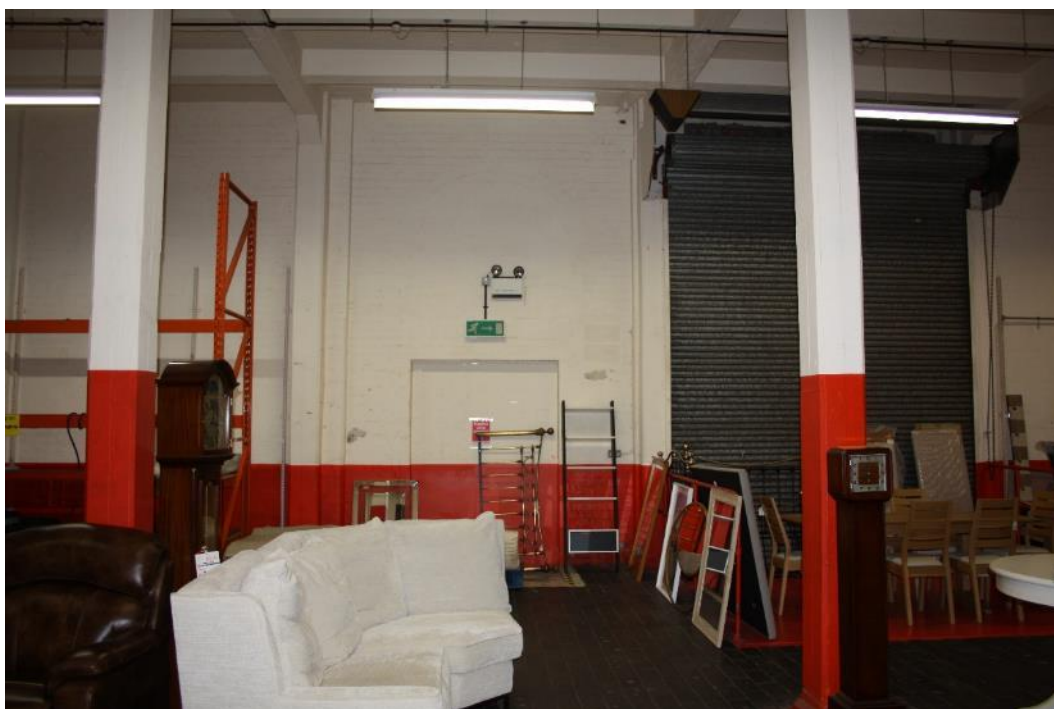
Plate 30: South east wall of Room 2 including a sample of the blocked in arch openings
