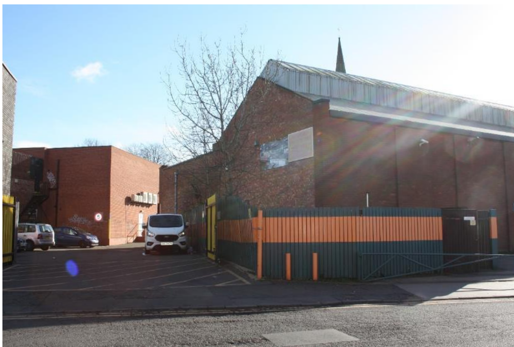
Plate 5: General view of the north east elevation as seen from Silver Street
