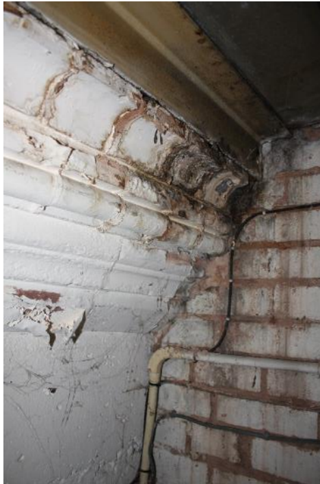
Plate 46: Detailed view of coving along the north east wall of Room 8
