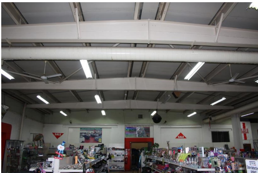
Plate 33: South east wall of Room 3
