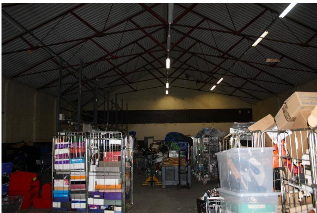
Plate 36: General view of Room 4 including the roof structure
