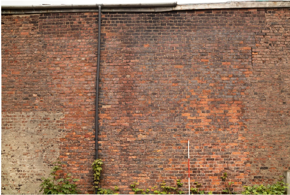
Plate 5: areas of patching and repair in the south-west elevation, facing north-east.
