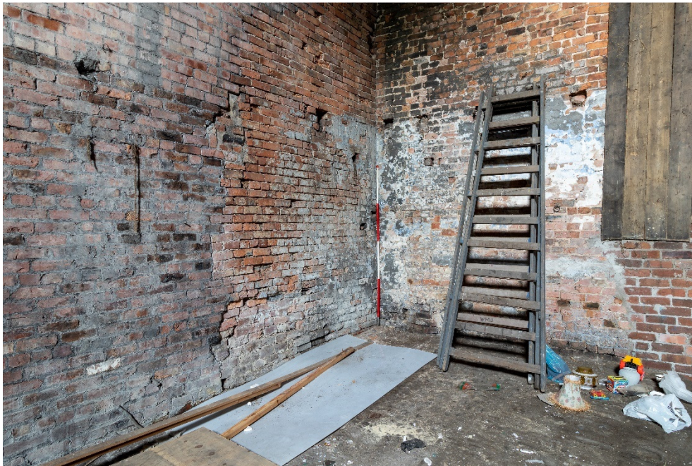
Plate 21: rebuilding and joist slots visible in the walls of Room 10b, facing west.
