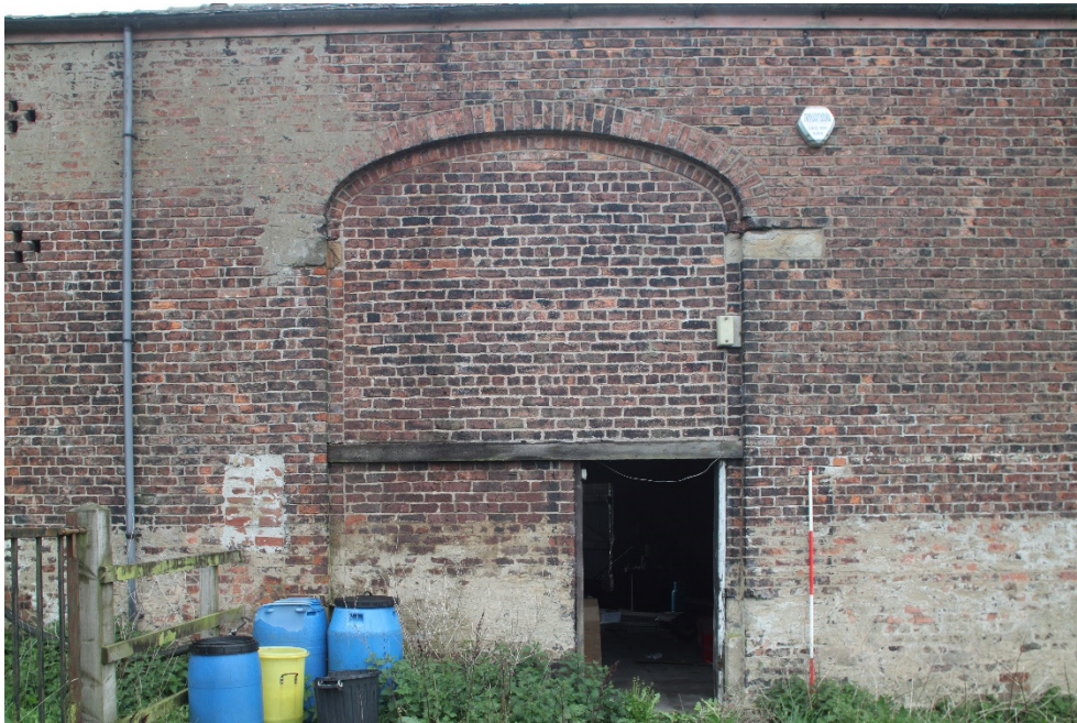
Plate 8: blocked barn door within the north-east elevation, facing south-west.
