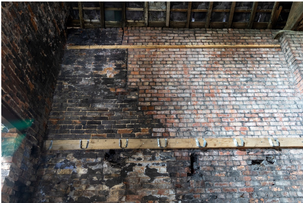
Plate 22: Rebuilding in the south-west wall of Room 10b, facing south-west
