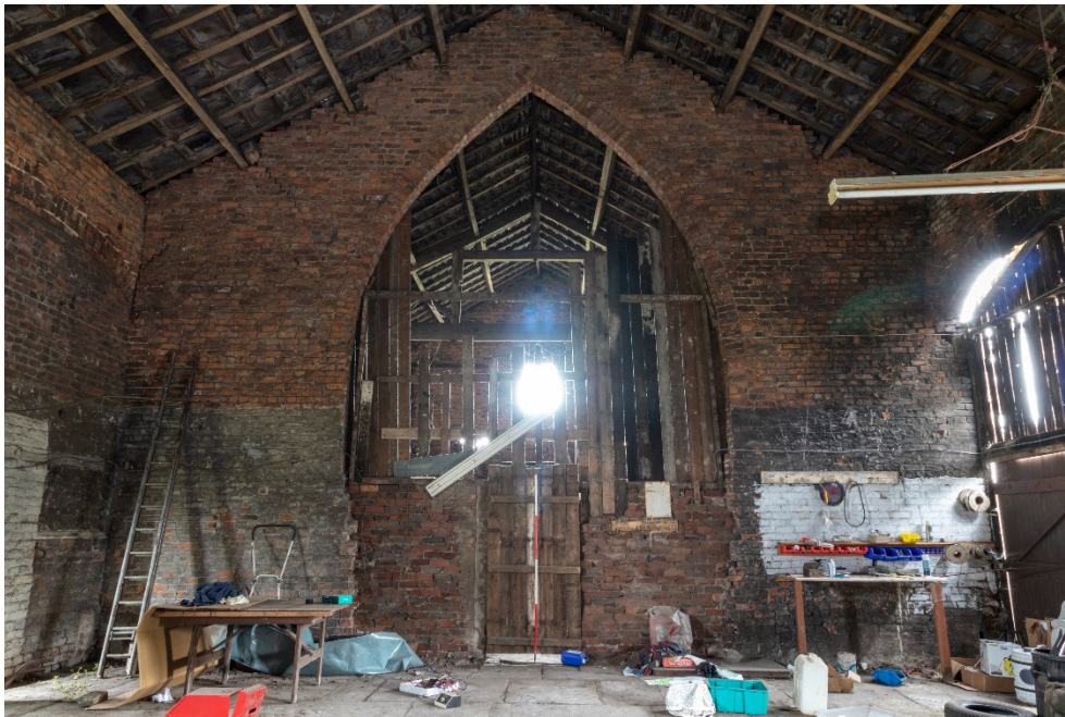
Plate 15: equilateral arch (Arch B) set into the wall dividing Room 9 from Room 10, facing south-east.
