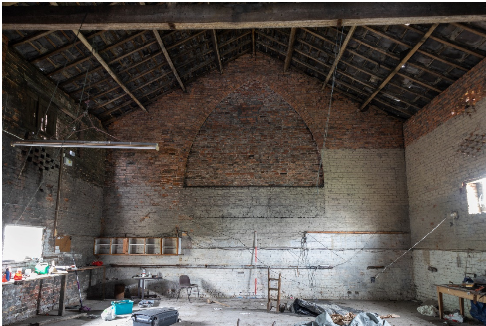
Plate 14: equilateral Arch A within the wall dividing the house from barn, facing north-west.
