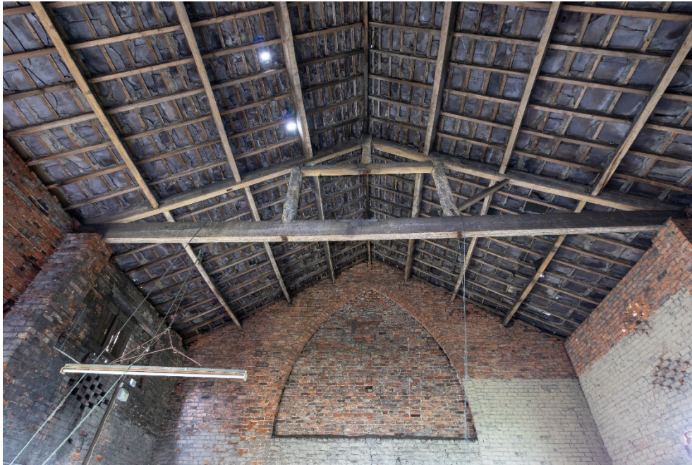
Plate 27: internal view of roof showing gradually narrowing slate battens towards the ridge, facing north-west.
