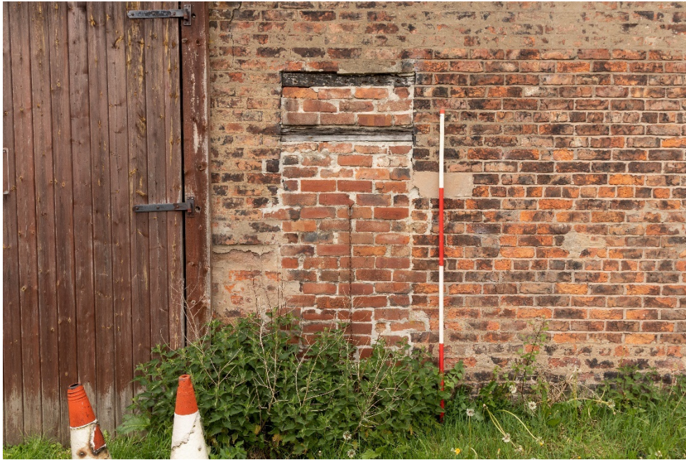
Plate 11: blocked door, south-east elevation, facing north-west.
