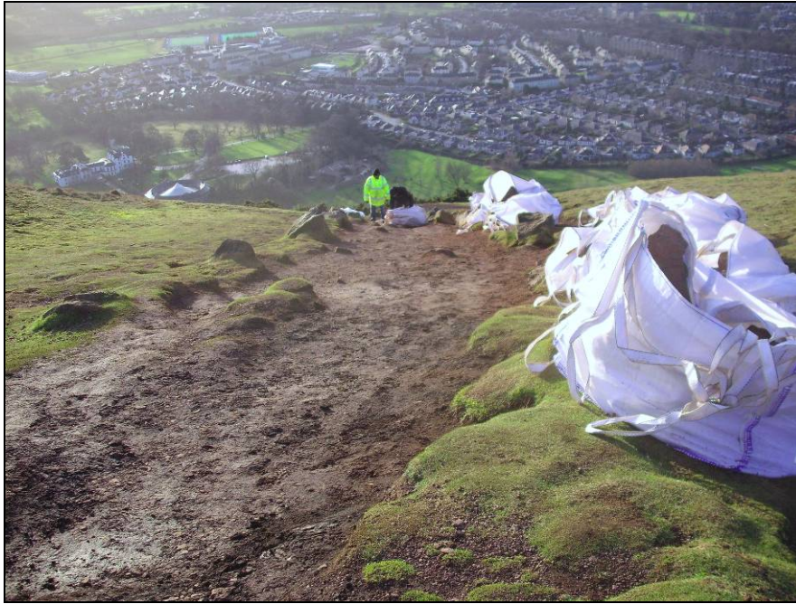
Figure 1: Nether Hill prior to new steps being laid.
