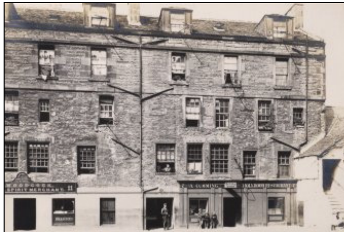
Figure 2-5: A view of the buildings at Abbey Strand in August 1903, before restoration (RCAHMS DP093672)
