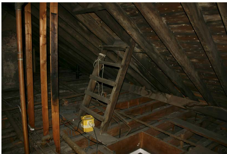
Fig. 128-44 View from south showing northern rafter (136) and northern collar-beam (138) of truss 33 (sevenths couple from right).
