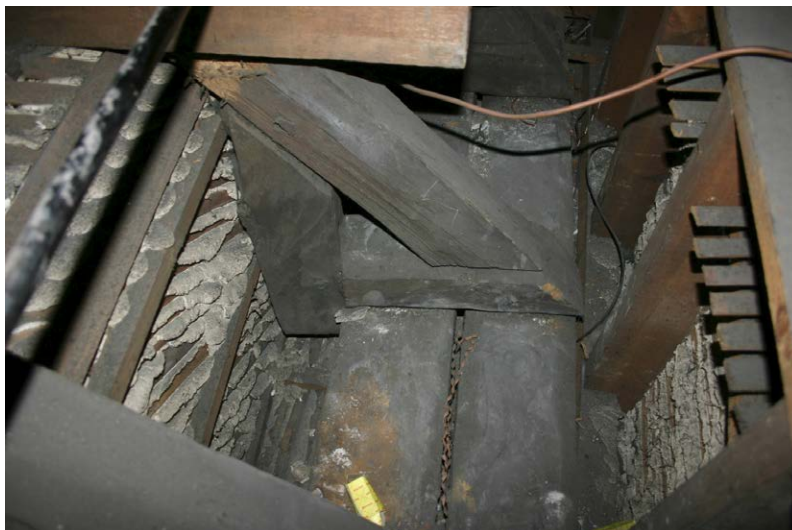
Fig. 131-11 View from west showing wall-plates 100 and 101 of trusses 1-7.
