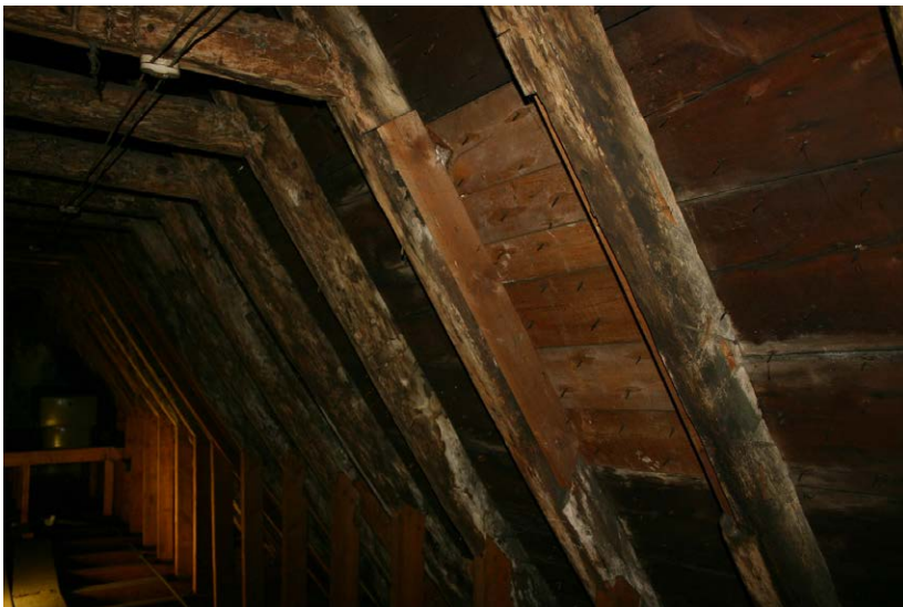
Fig. 130-18 View from south showing eastern rafter (179) and upper collar-beam (181) of truss 18.
