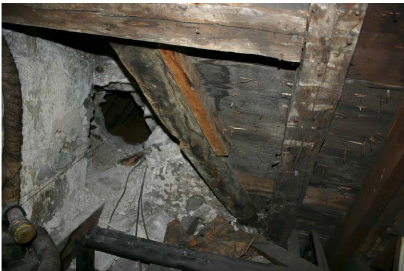
Fig. 131-23 View from north showing trimmer (154) and hip-rafter (155) of trusses 11-13.
