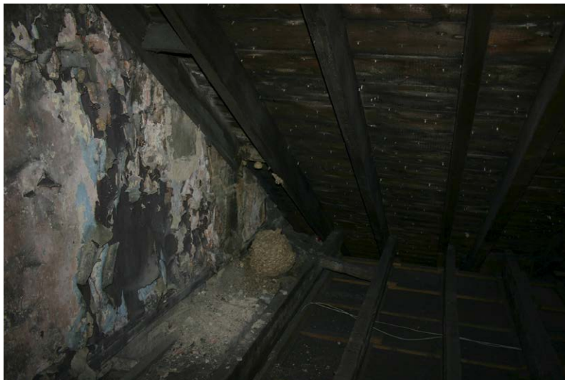
Fig. 128-1 View from northeast showing southern rafter (002) and southern collar-beam (004) of truss 1 (first couple from left).
