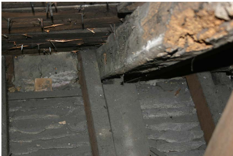
Fig. 130-3 View from west showing rafter 072, collar-beam 076 and auxiliary collar-beam 077 of truss 3.
