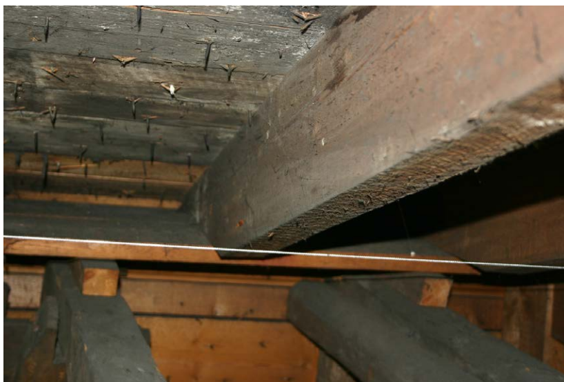
Fig. 132-18 View from west showing rafter 055.
