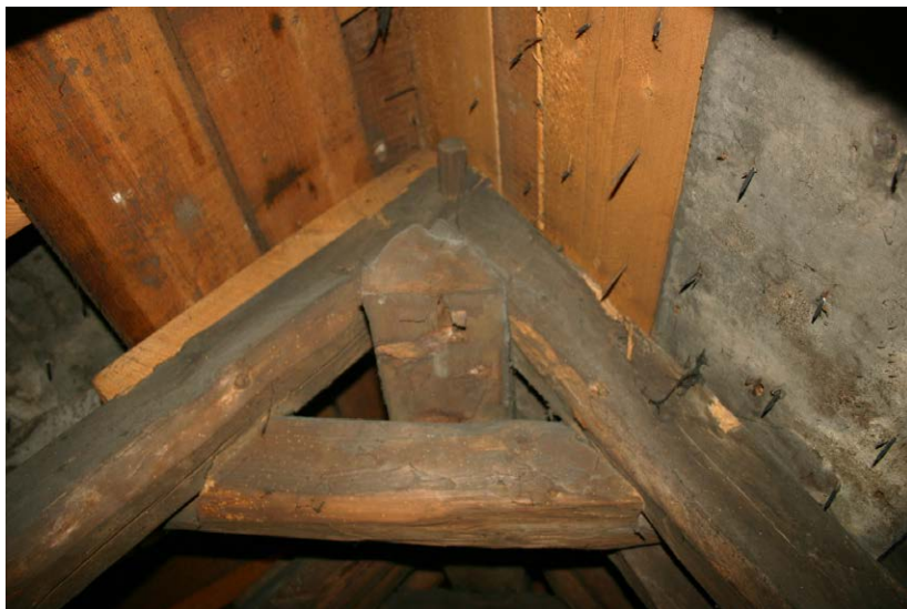
Fig. 132-11 View from south showing ridge-purlin 043.
