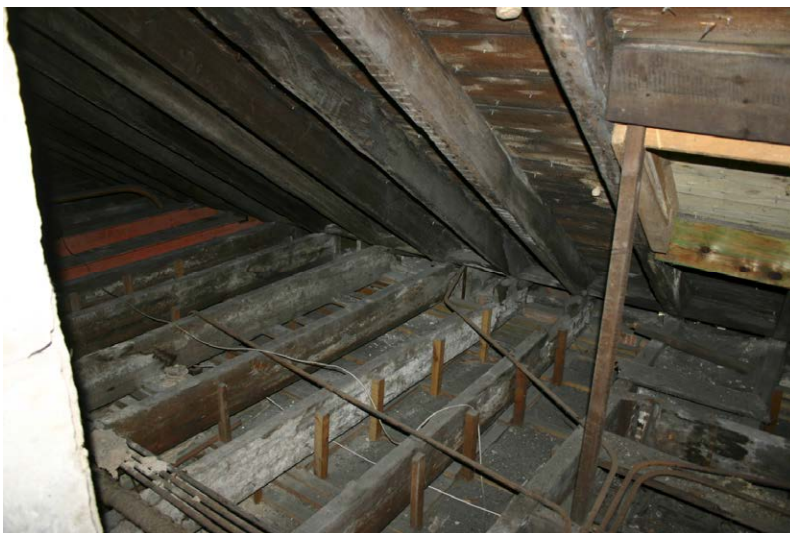
Fig. 128-23 View from southeast showing collar-beam (074) and northern rafter (073) of truss 13 (forth couple from right).
