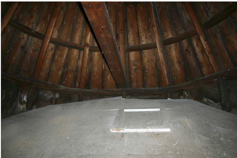
Fig. 136-18 View from north showing rafter 16 (third rafter from left).
