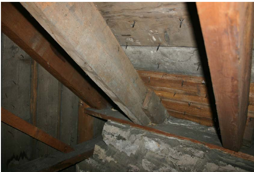
Fig. 132-15 View from northeast showing rafter 049 and board 050.
