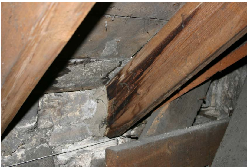
Fig. 132-23 View from southeast showing rafter 062.
