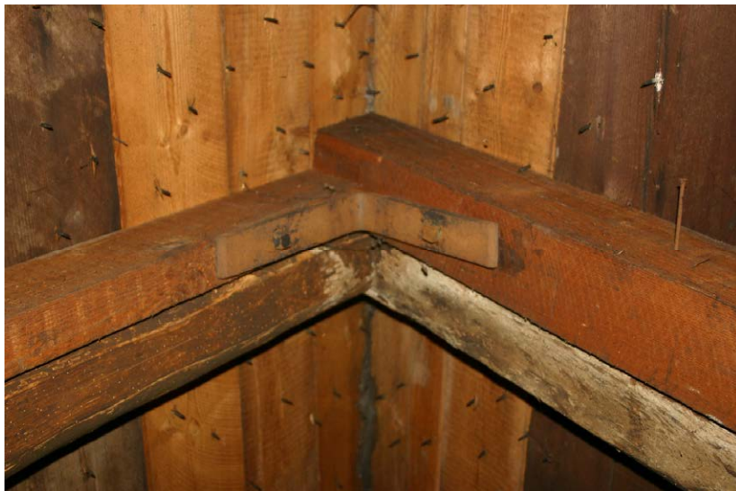
Fig. 130-20 View from southeast showing eastern and western rafters (193 and 195), eastern and western auxiliary rafters (194 and 196) and upper collar-beam (197) of truss 20.
