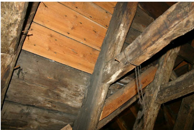
Fig. 130-13 View from east showing western rafter (146) and upper collar-beam (147) of truss 13.
