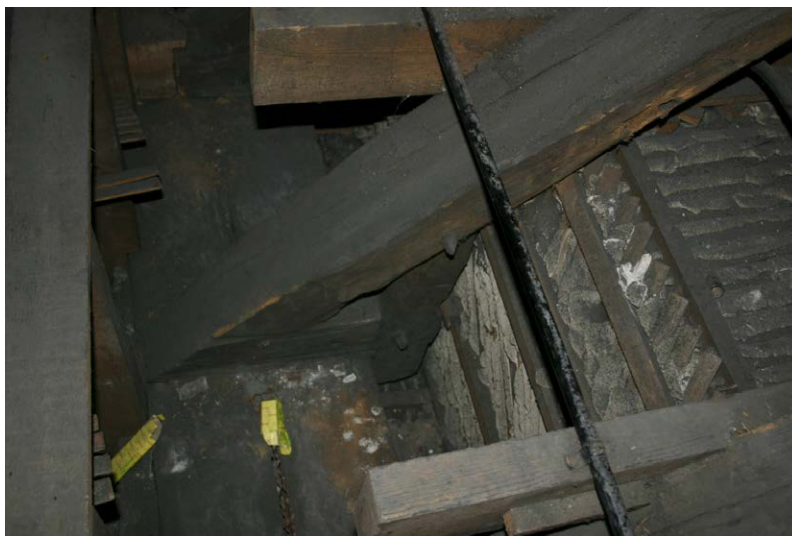
Fig. 131-6 View from west showing southern rafter (075), sole-piece (077) and ashlar-post (076) of truss 4.
