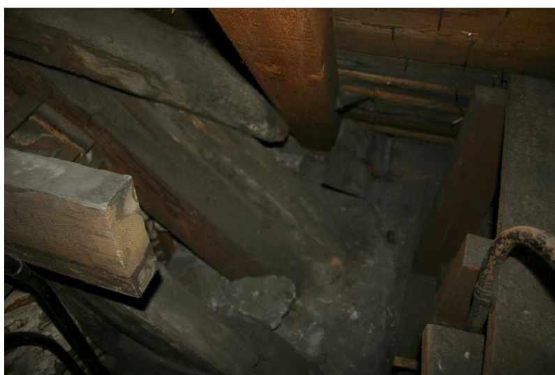
Fig. 131-13 View from west showing southern rafter (108) of truss 9.
