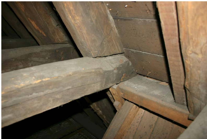
Fig. 131-12 View from south showing northern rafter (102) and upper collar-beam (106) of truss 8.
