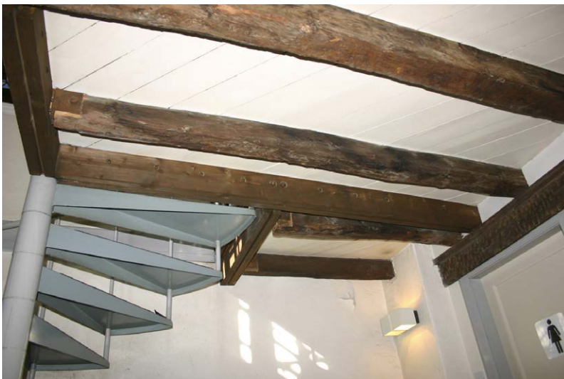
Fig. 028-8 View from east showing joist 069 (third joist in front of west-wall).
