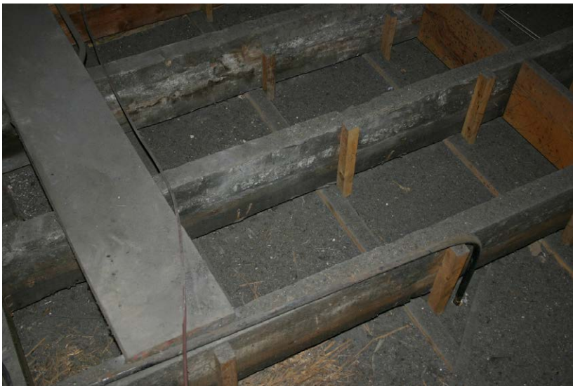
Fig. 128-18 View from west showing collar-beam (051) of truss 16 (second beam from bottom).
