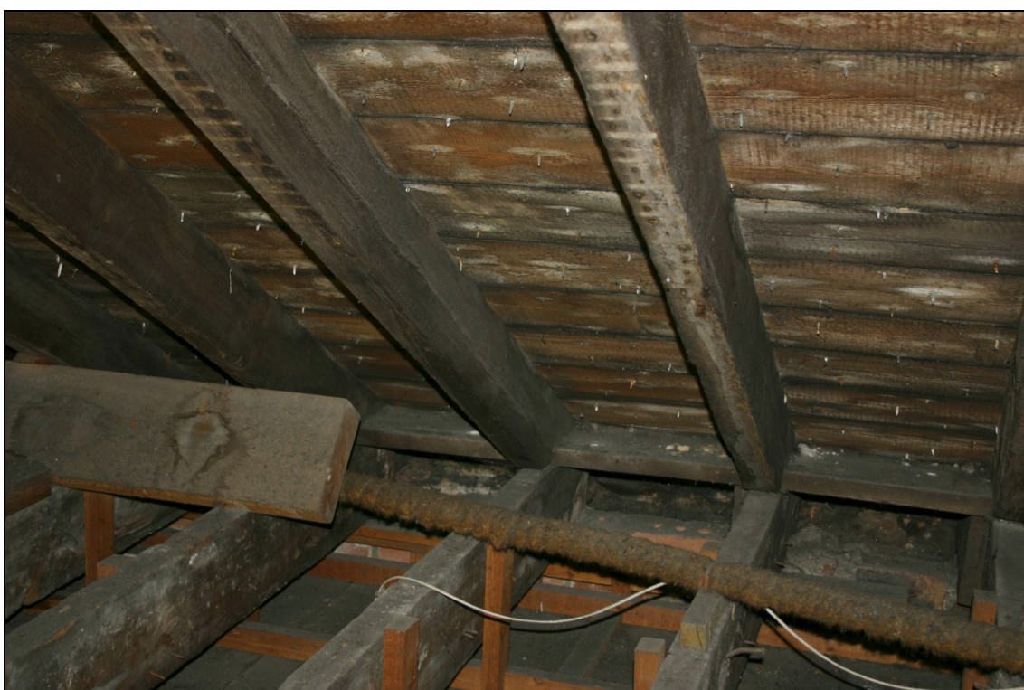
Figure A1-3: Joint between collarbeam and northern rafter over the main block. The collarbeam sits in the structural axis of the rafter, thus differing from the solution visible in Fig. 2.
