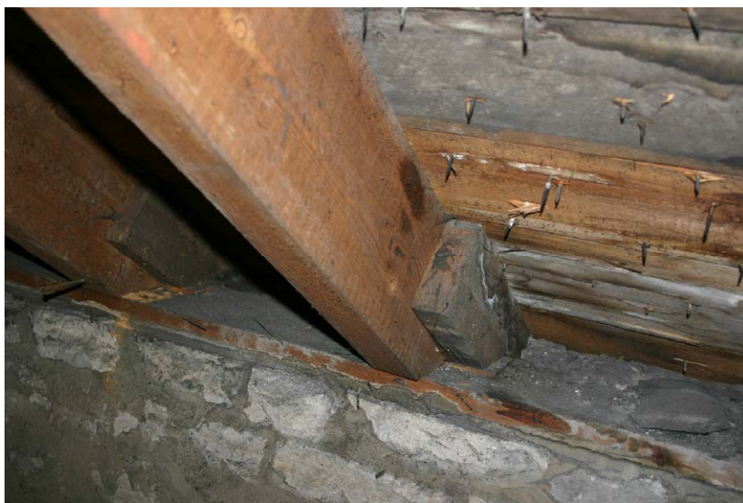
Fig. 132-19 View from northeast showing rafter 057 and board 058.
