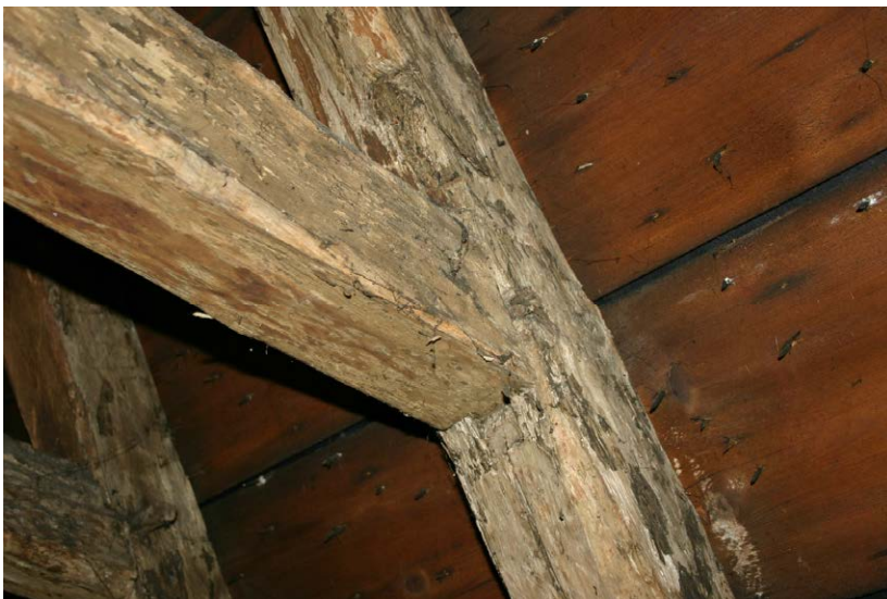
Fig. 130-5 View from southwest showing rafter 087 and collar-beam 089 of truss 5.
