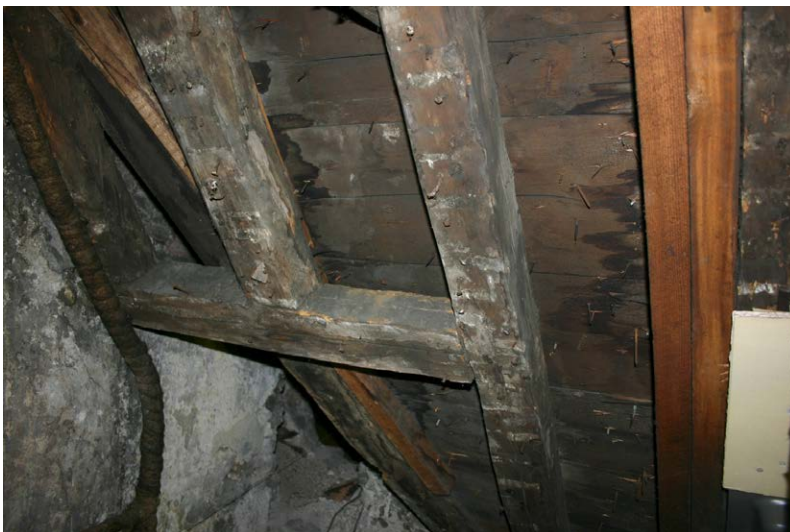
Fig. 131-19 View from north showing southern rafter (142) of truss 11.
