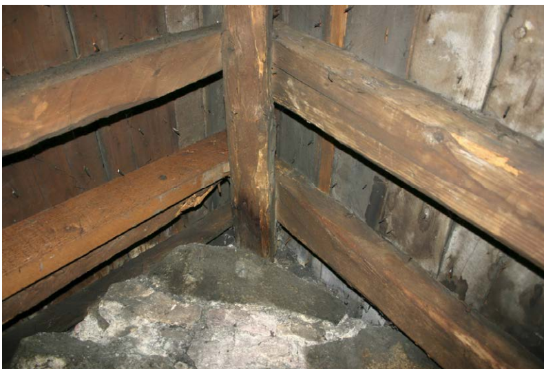
Fig. 131-21 View from west showing northern and southern rafter (148 and 149) of truss 13.
