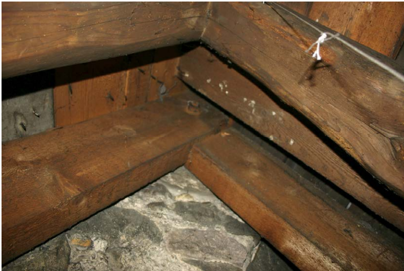
Fig. 132-1 View from north showing eastern and western rafters (001 and 002) of truss 1.
