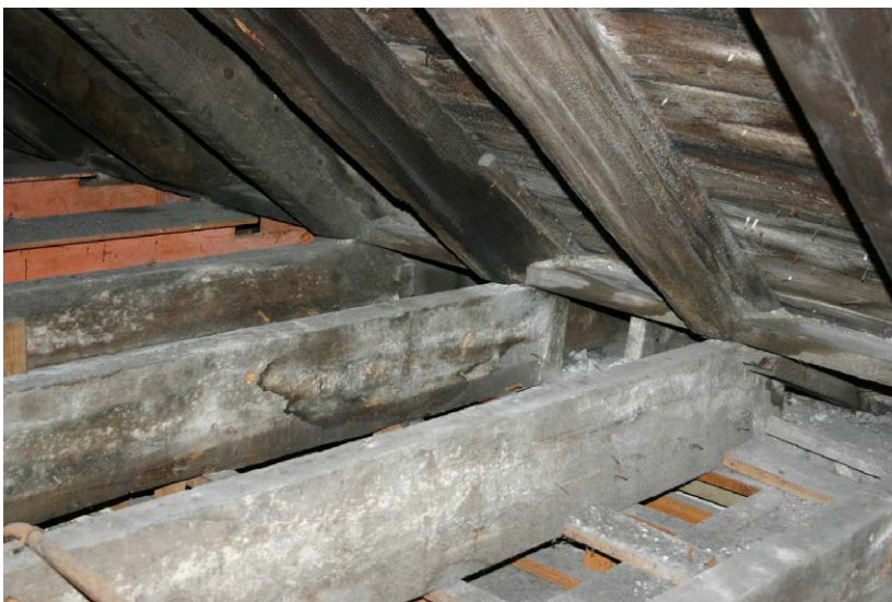
Fig. 128-26 View from southeast showing collar-beam (080) and northern rafter (079) of truss 16 (fourth couple from right).
