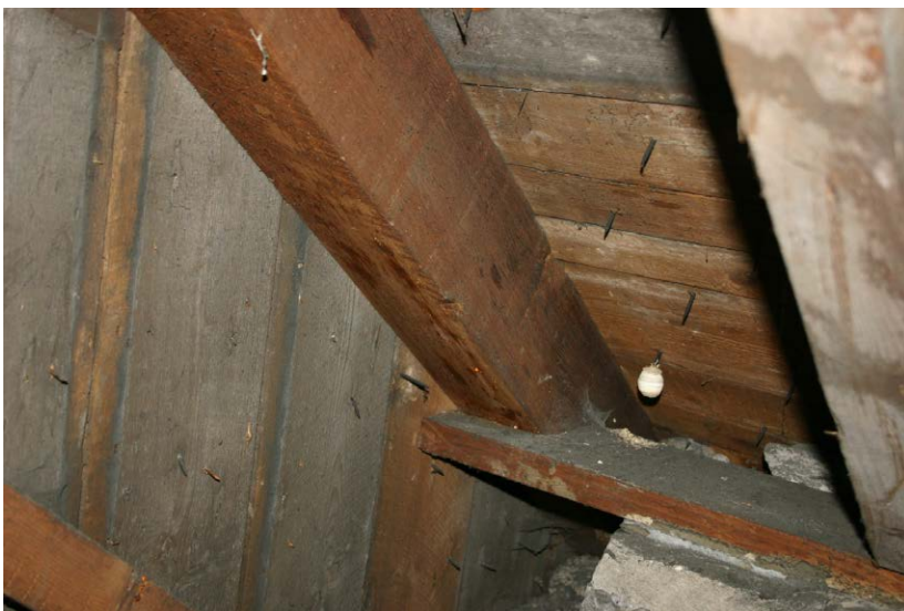
Fig. 132-14 View from northeast showing rafter 048
