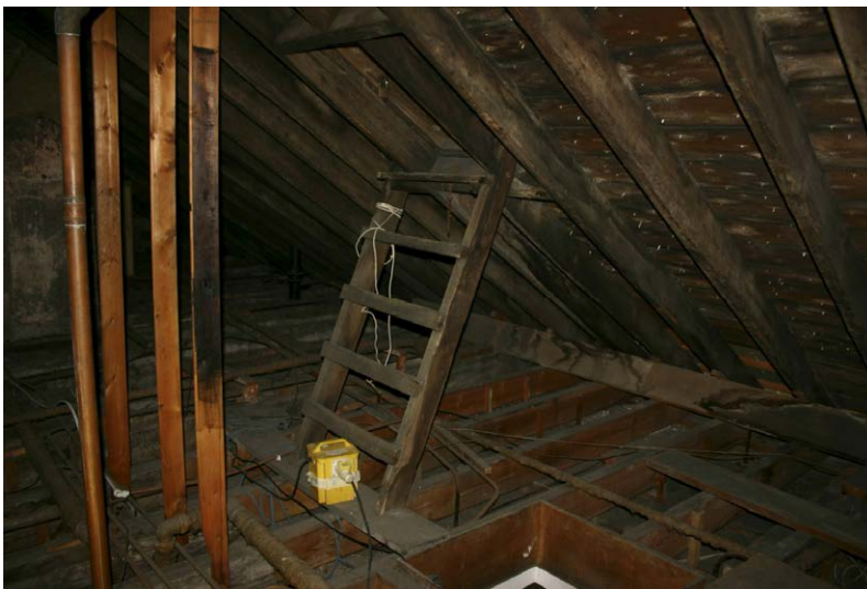
Fig. 128-43 View from south showing northern rafter (132) and northern collar-beam (134) of truss 32 (sixth couple from right).
