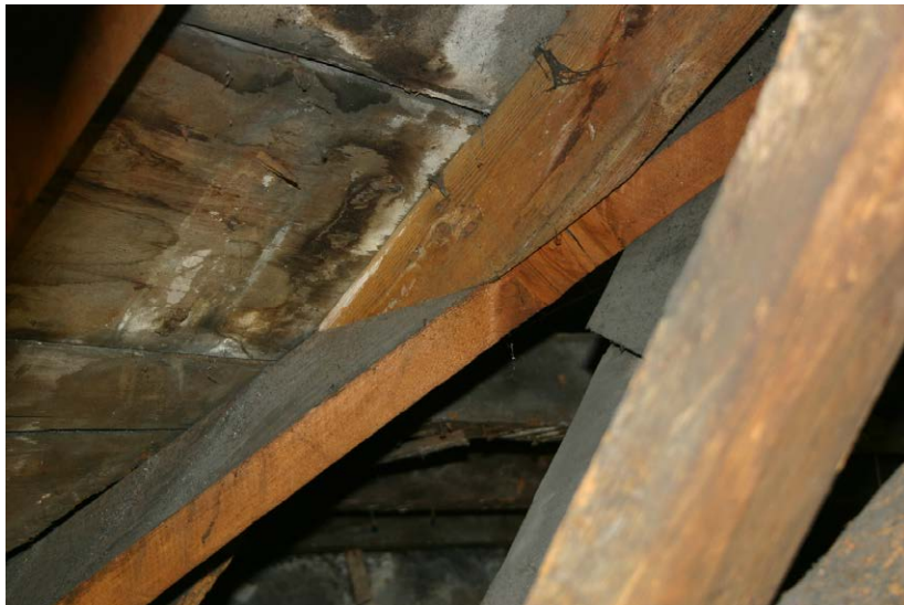
Fig. 132-24 View from southeast showing hip-rafter (063) and rafter (065).
