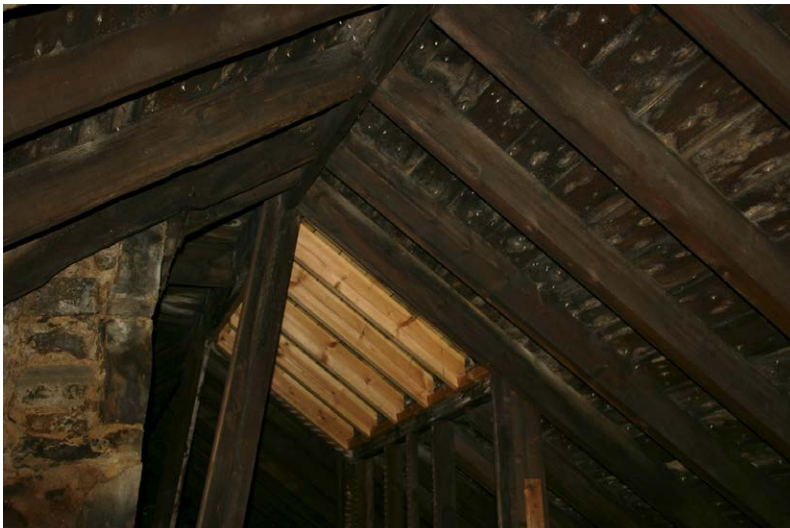
Fig. 128-19 View from west showing posts 052-060 and trimmer 061.
