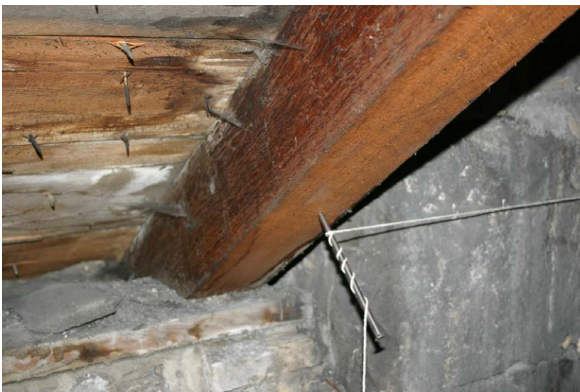
Fig. 132-20 View from southeast showing rafter 059.
