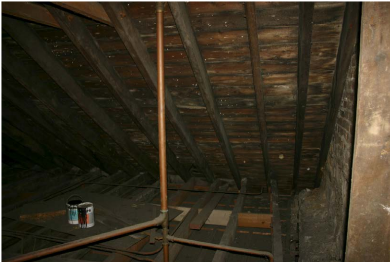
Fig. 128-63 View from north showing southern rafter and collar-beam of truss 46 (fourth rafter from right).
