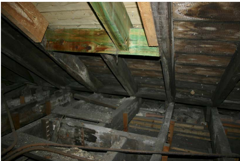
Fig. 128-12 View from south showing bottom trimmer 037 between rafters 025 and 032 and northern and southern trimmers (038 and 039) between collar-beams 027 and 034.
