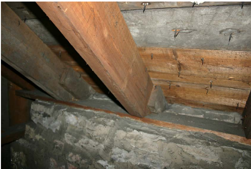
Fig. 132-16 View from northeast showing rafter 051 and board 052.
