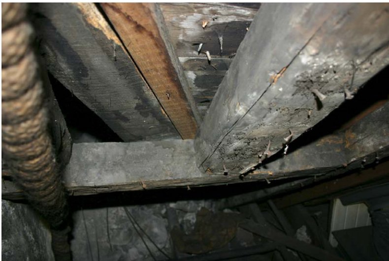
Fig. 131-20 View from north showing southern rafter (147) of truss 12.
