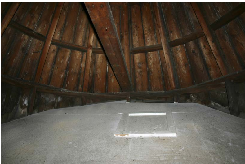
Fig. 136-17 View from north showing rafter 15 (second rafter from left).
