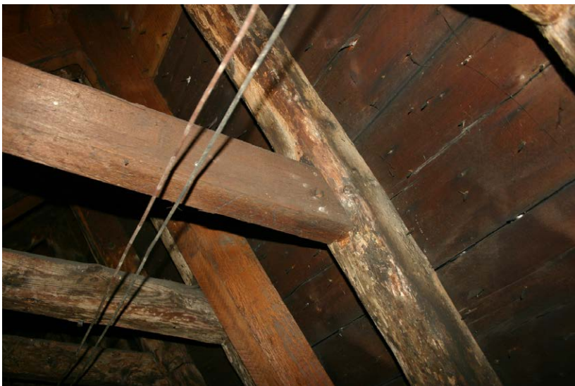
Fig. 130-21 View from south showing eastern rafter (202) and upper collar-beam (204) of truss 21.
