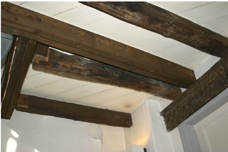
Fig. 028-9 View from east showing joist 070 (second joist in front of west-wall).
