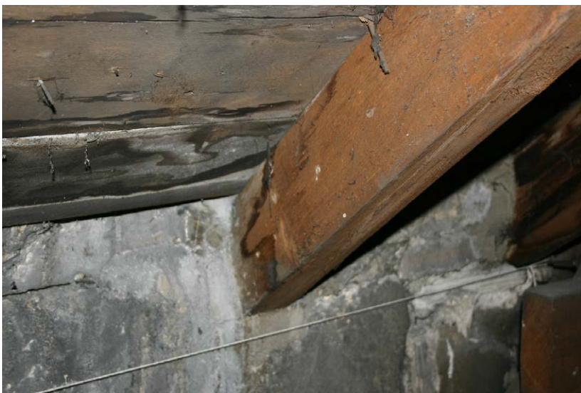
Fig. 132-22 View from southeast showing rafter 061.
