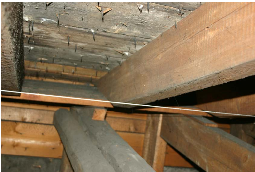
Fig. 132-17 View from west showing rafter 053.
