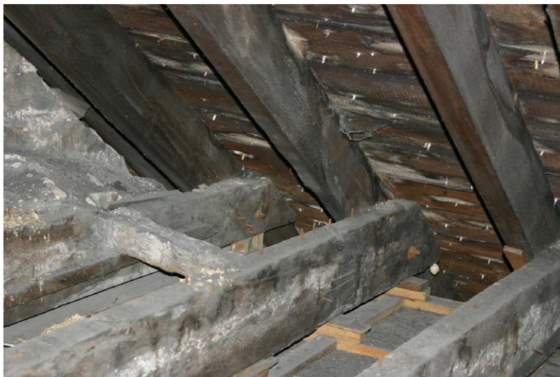
Fig. 128-2 View from northeast showing southern rafter (005) and collar-beam (006) of truss 2 (third couple from right).
