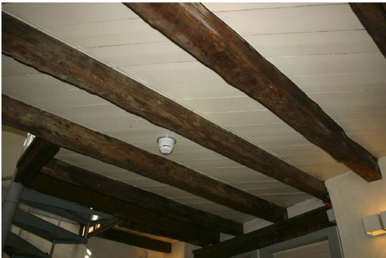
Fig. 028-5 View from southeast showing joist 066 (second joist from right).
