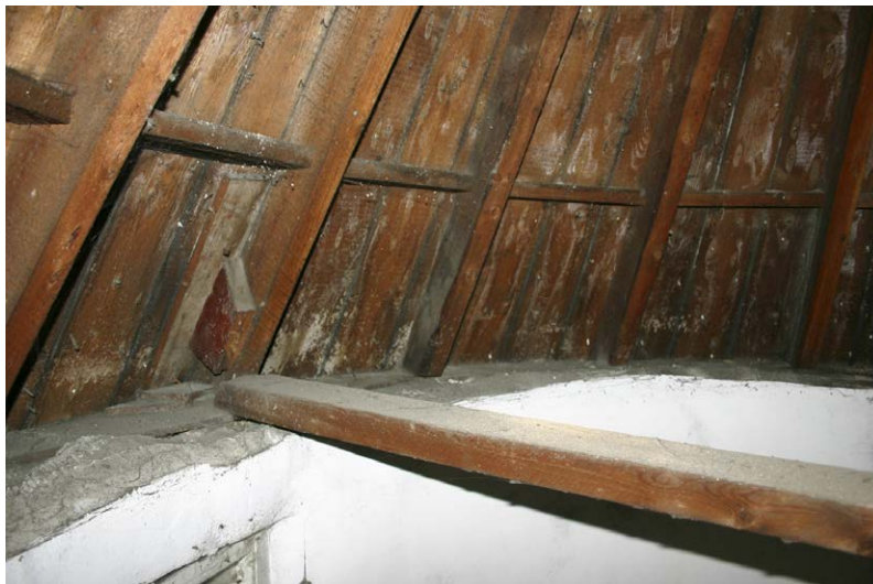
Fig. 136-15 View from north showing rafter 13 (fifth rafter from left).
