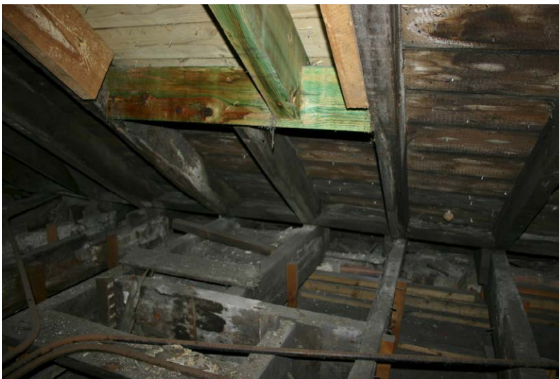
Fig. 128-11 View from south showing northern rafter (032) and northern collar-beam (034) of truss 10 (fourth couple from right).
