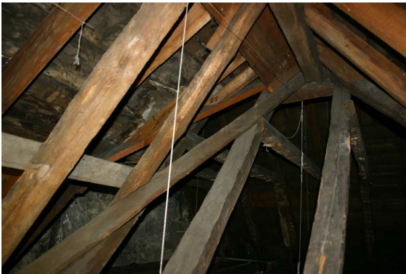
Fig. 132-10 View from south showing western hip-rafter (039) and rafters 041 and 042.
