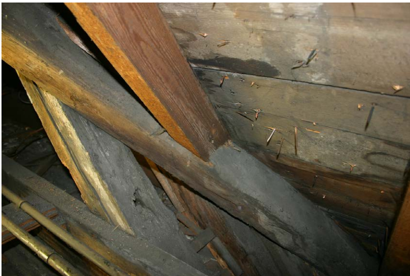
Fig. 132-9 View from south showing eastern hip-rafter (033) and rafter (034)
