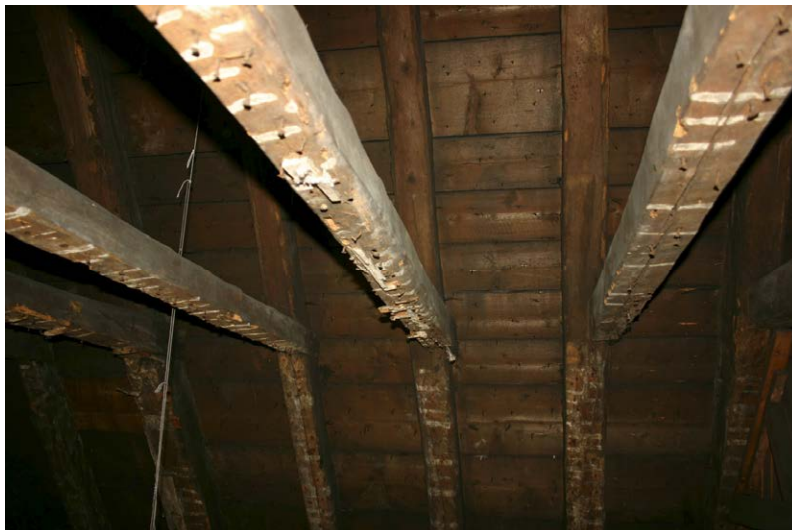
Fig. 131-8 View from south showing northern rafter (086) and upper collar-beam (090) of truss 6.
