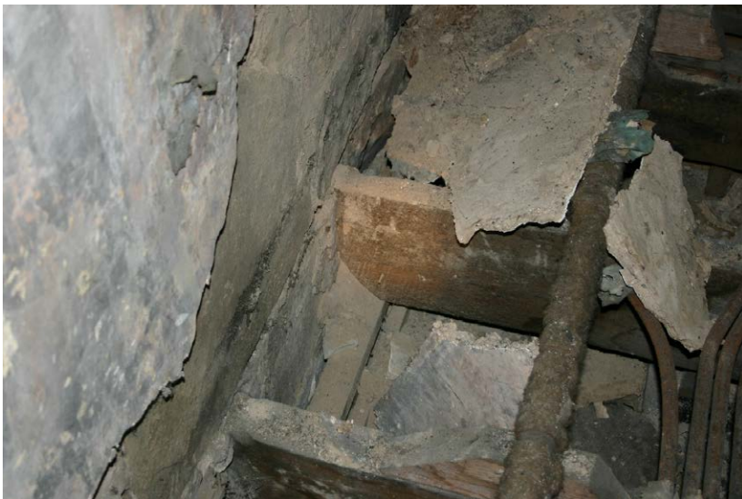
Fig. 128-24 View from east showing collar-beam (076) of truss 14 (second beam from bottom).
