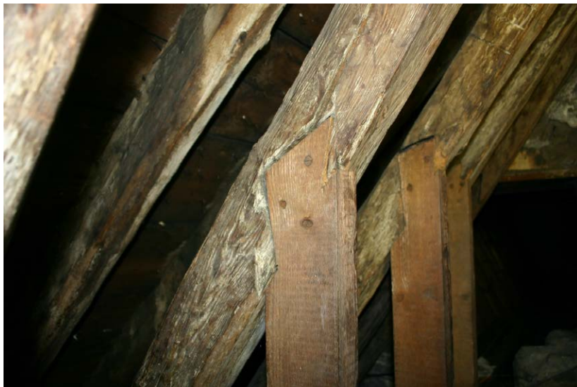
Fig. 130-4 View from south showing rafter 081 and strut 086 of truss 4.
