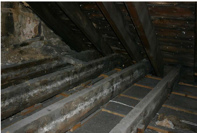
Fig. 128-6 View from northeast showing collar-beam (017) and southern rafter (016) of truss 5 (first couple from right).
