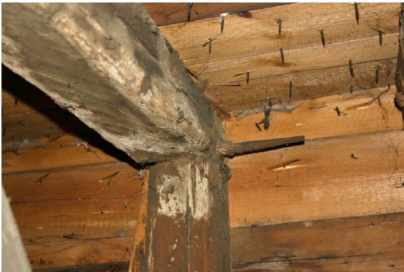
Fig. 130-11 View from west showing eastern and western rafter (129 and 130) of truss 11.
