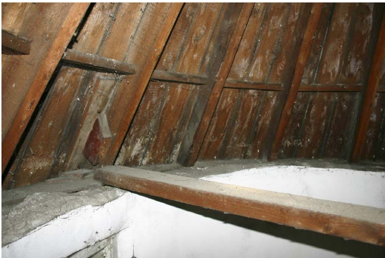
Fig. 136-12 View from north showing rafter 10 (third rafter from left).
