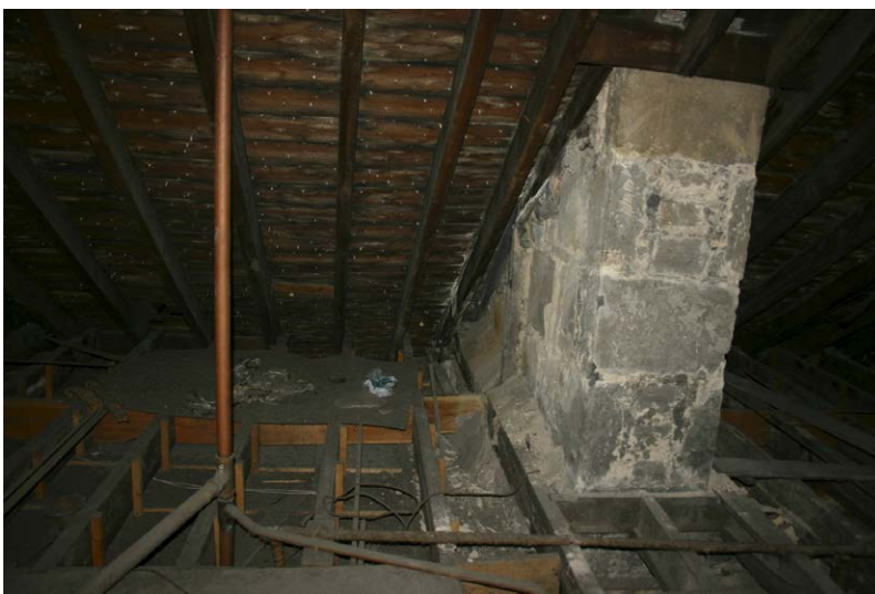
Fig. 128-31 View from north showing southern rafter (094) and collar-beam (095) of truss 21 (fifth couple from chimney).
