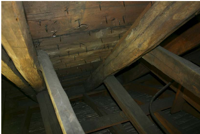
Fig. 132-5 View from west showing eastern rafter (013) and high and low collar-beams (015 and 016) of truss 5.
