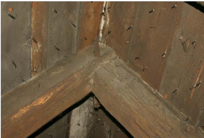
Fig. 131-7 View from east showing northern (080) and southern (081) rafter of truss 5.
