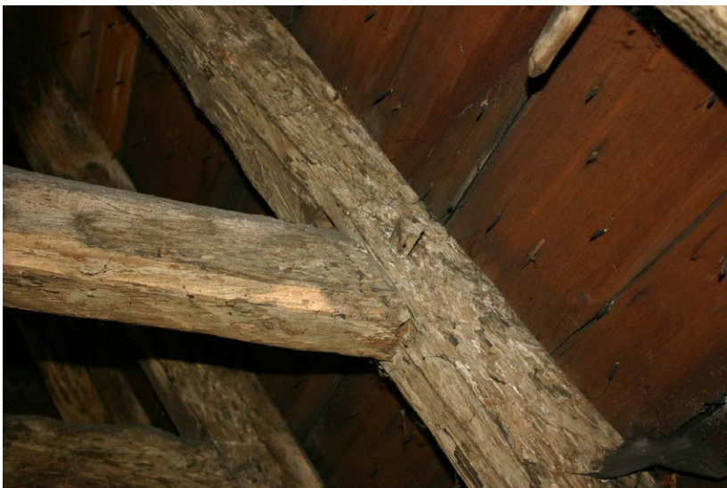
Fig. 130-10 View from south showing eastern rafter (122) and upper collar-beam (124) of truss 10.
