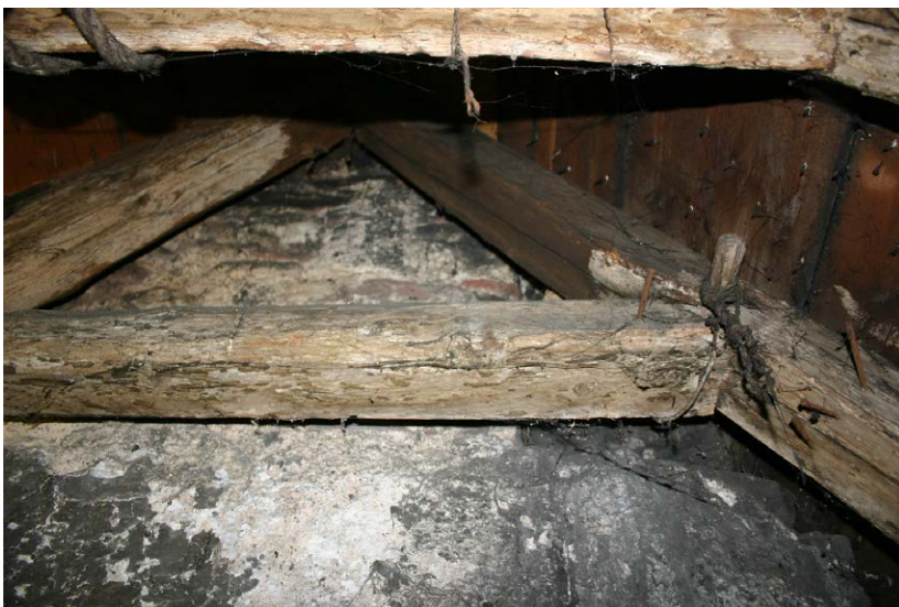
Fig. 130-1 View from South showing rafters 060 and 061 and collar-beam 062 of truss 1.
