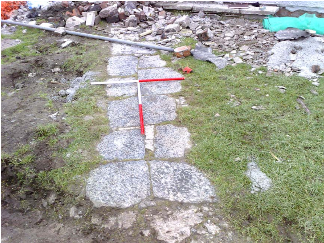
Plate 1: The existing path to the SE door prior to excavation
