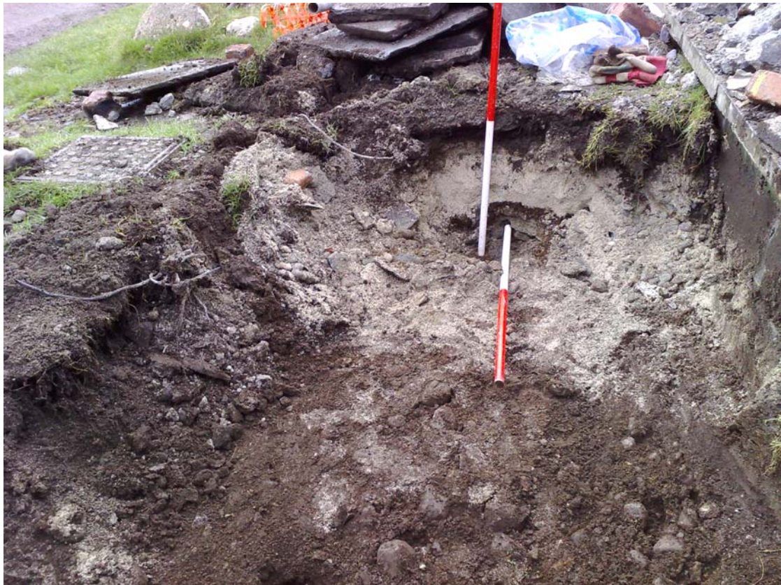
Plate 2: Looking S pipe cut F304 and backfill F303
