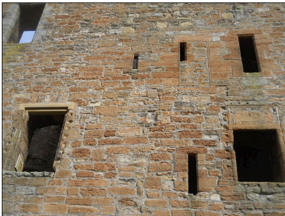
Fig. 3: Features 100-103 at the W-wall of the SW-Tower.
