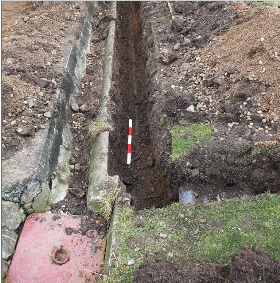
Plate 1: The work in progress.
