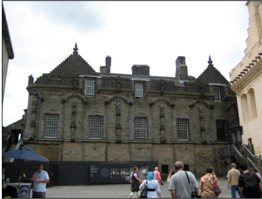
Figure 13: The E-façade of Stirling Palace (c.1538). James V's elevation, employing two crow-stepped gables at the northern and southern ends of the E-range, implies that the original roof over the S-range resembled the current roof-architecture. This can be assumed because the gable-triangle ultimately defines the pitch, height and width of the roof. It is therefore highly likely that the U20 arch was created by James V's craftsmen.
