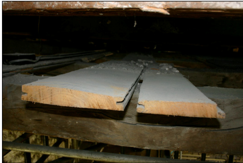
Figure 3: Floorboards (1538d) and joists (1538d) over the Queen's Bedchamber.
