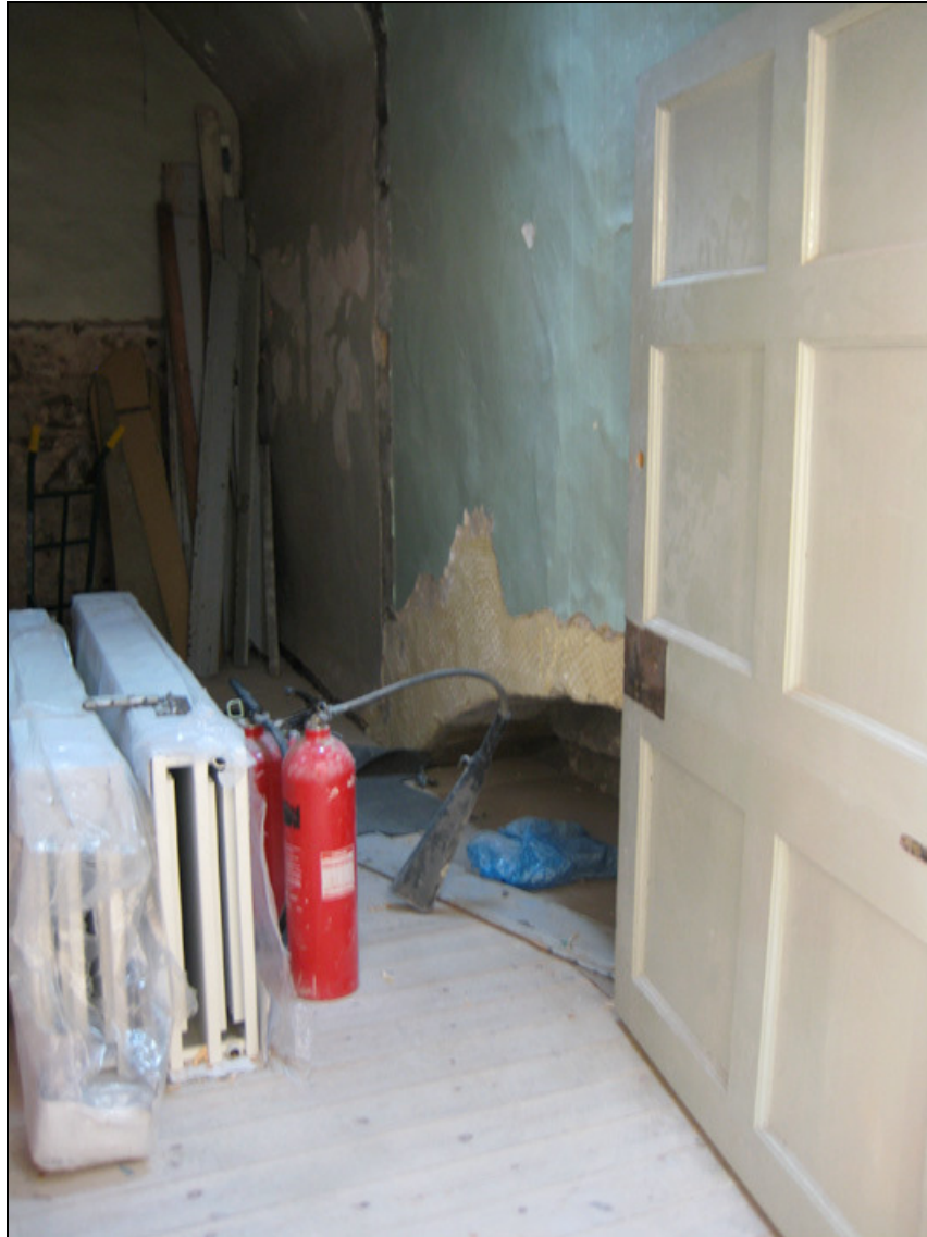
Figure 16: The eastern part of the relieving arch in U19, U21 and U22 (probably c.1538).
