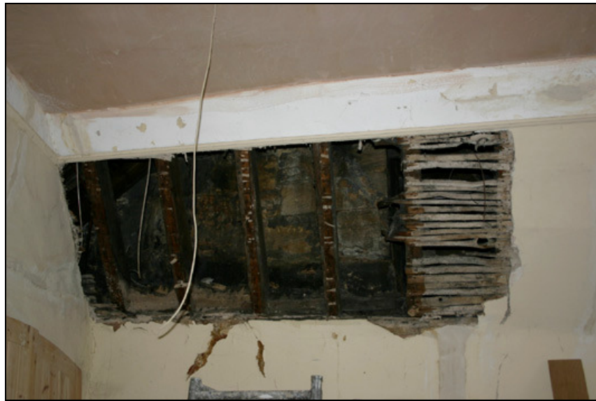
Figure 5: The chimney inside the N-wall of U20 (probably c.1538).
