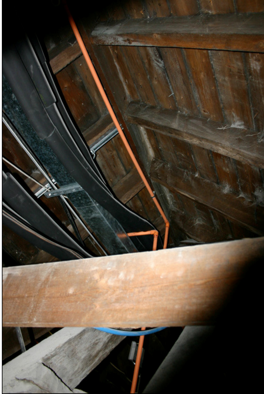
Figure 12: The roof R05 over U20 (post-C17).
