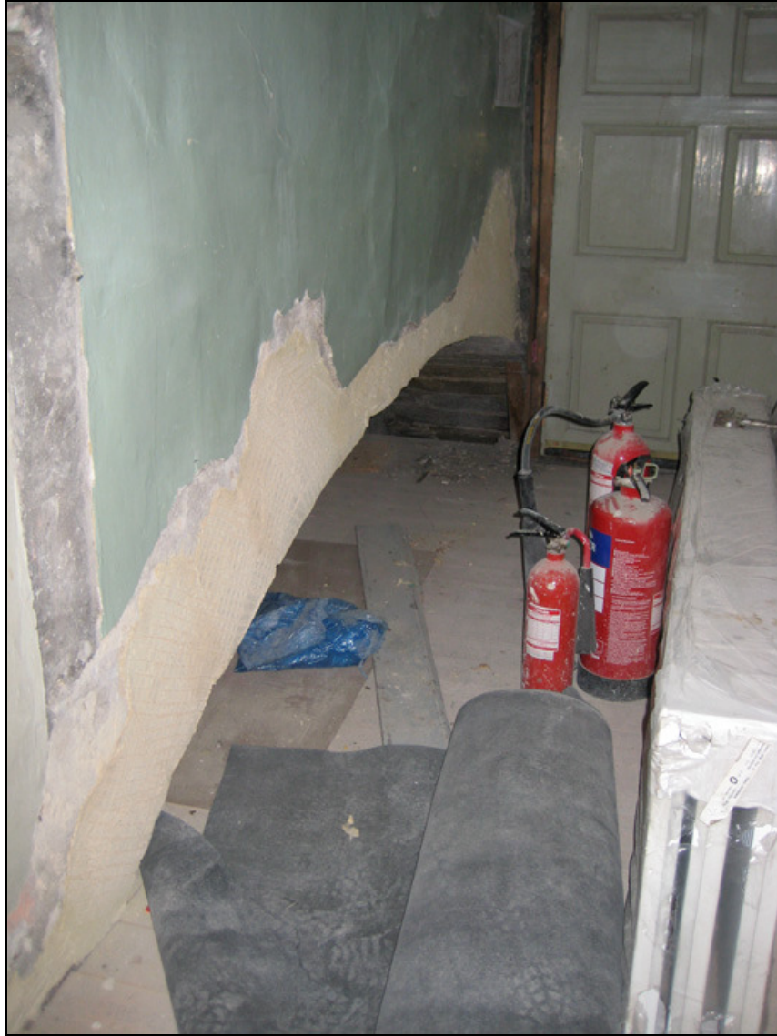
Figure 15: The relieving arch in U19, U21 and U22 (probably c.1538).
