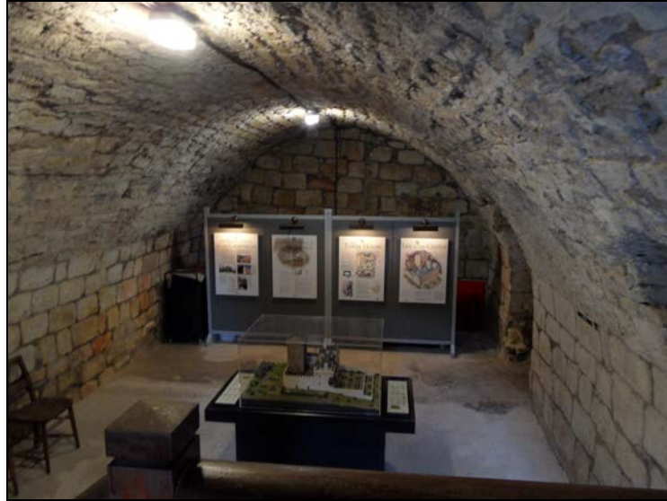
Plate 2.3: The undisturbed masonry of the ground floor cellar vault.
