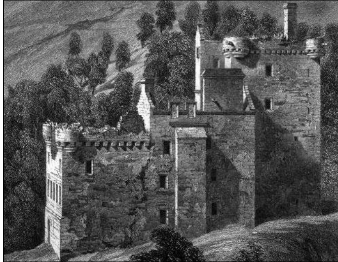
Figure 3.1: Robert Billings' 1847 illustration of the east elevation shows a much squatter chimney crowning the south gable of the east range – this was altered in the late-19 th century. The chimney on the east wall has a large chamfered crown which has been removed.
