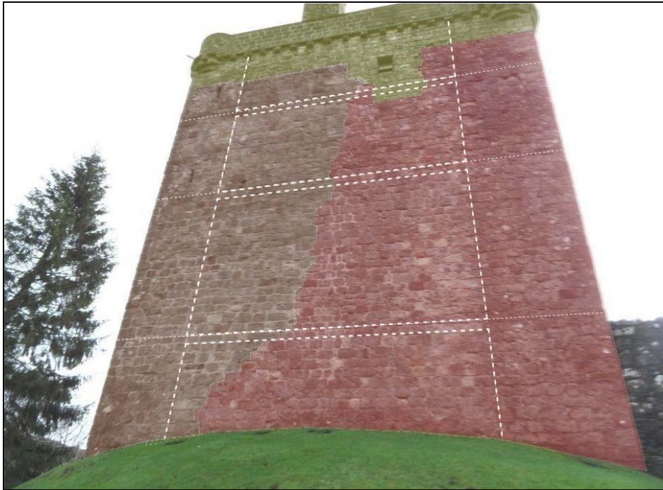
Plate 2.1: The external north wall with room limits and floors imposed. The red build is original, the brown build was added, and the yellow build represents the insertion of the new 3 rd floor vault along with upper wall courses and parapet. At ground level it can be seen that internally the vault could have been preserved while externally portions of the original masonry were lost.
