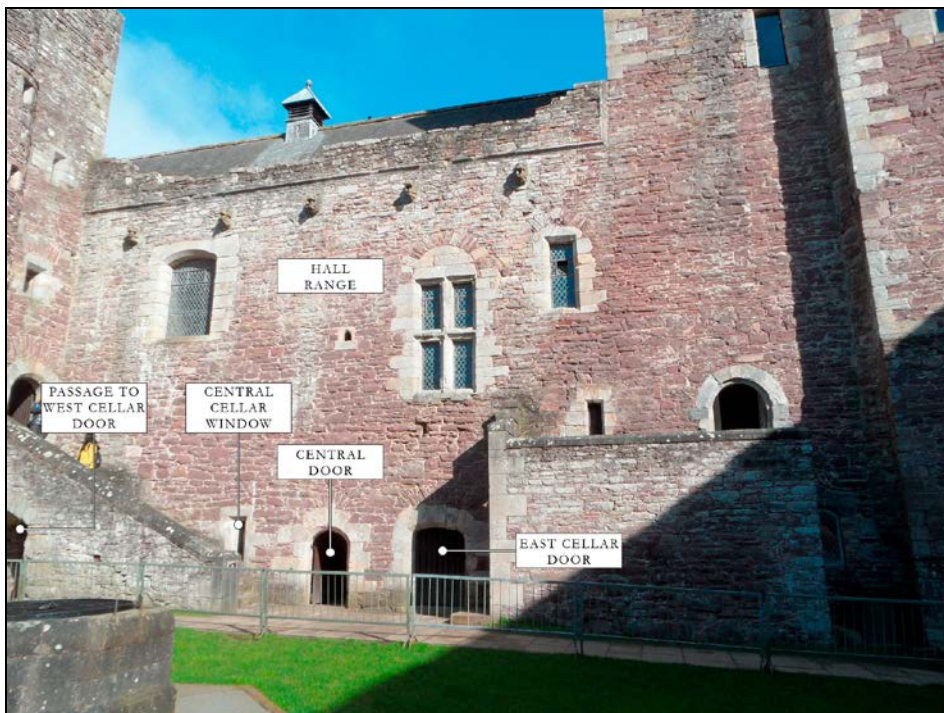
Plate 1: Looking north from the courtyard, showing the layout of the ground floor cellars of the hall range.
