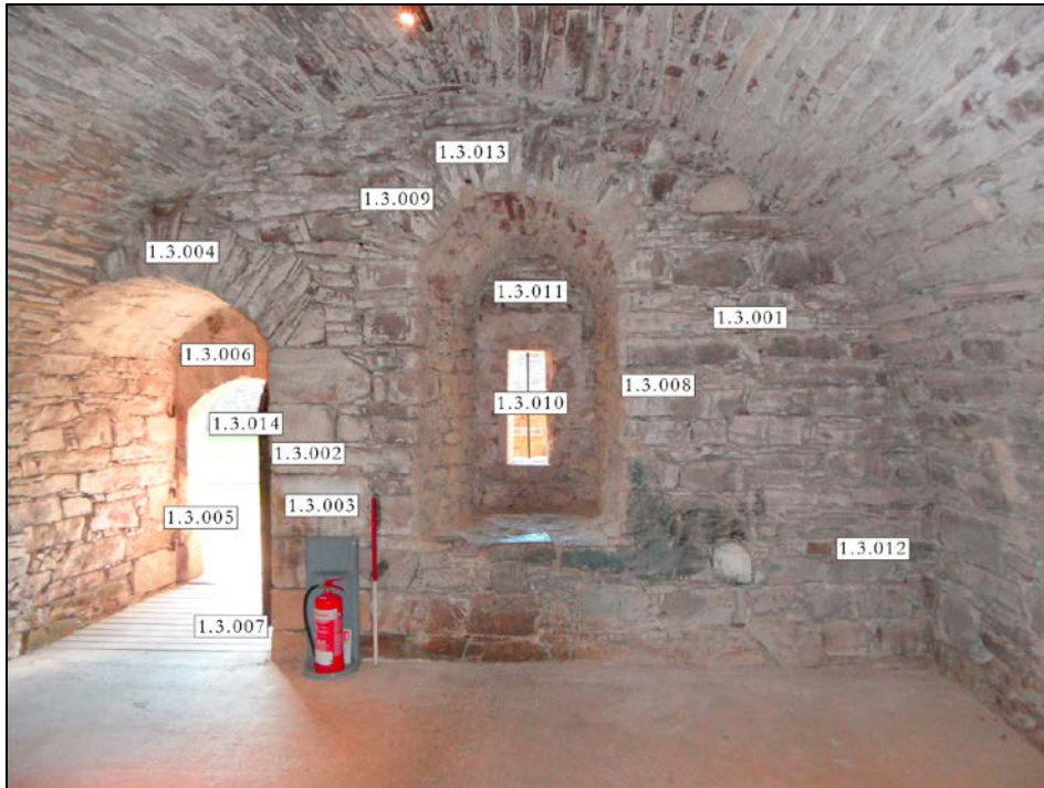
Plate 4: Features on the south wall.
