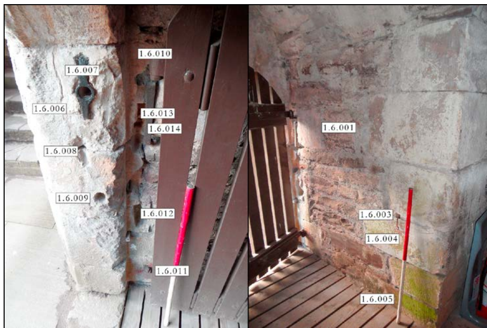
Plate 7: Features on the west wall of the door lobby.
