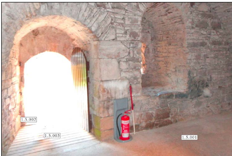
Plate 6: Features on the cellar floor.
