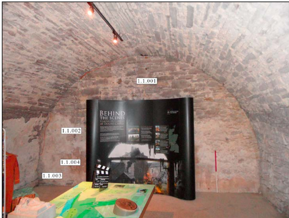
Plate 2: Features on the north wall.
