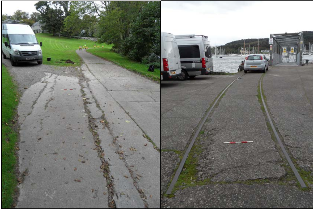
Plate 2: Backfilled rail tracks in the vicinity of the trench (left) and in-situ steel rails at the pier (right).
