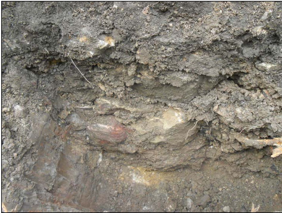
Plate 3: The western end of Trench 3, showing wall 305.
