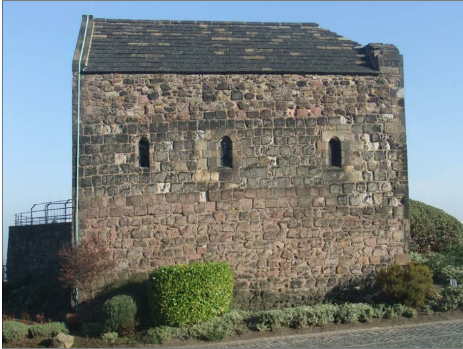
Plate 3: General view of the chapel south wall.
