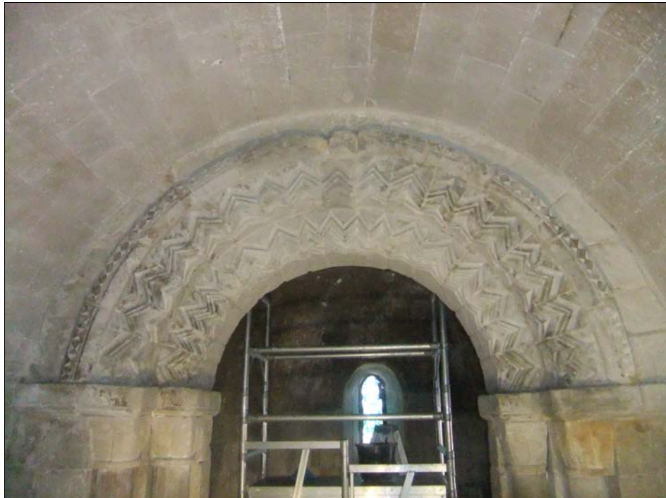
Plate 5: East wall of the nave, detail of upper part.
