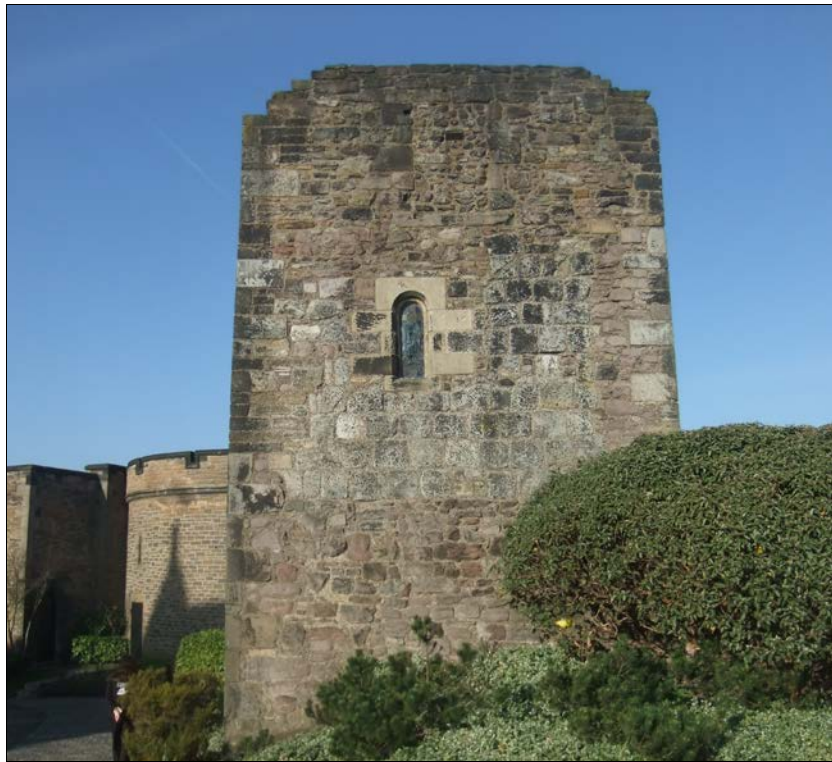
Plate 4: General view of the east wall.
