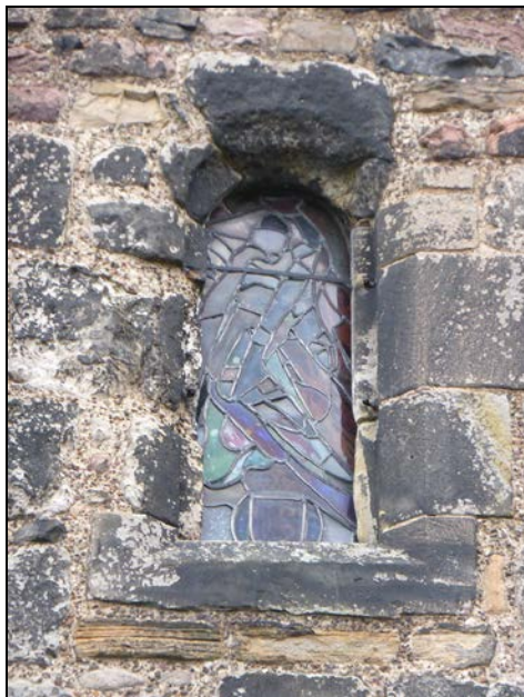
Plate 2: West window exterior.
