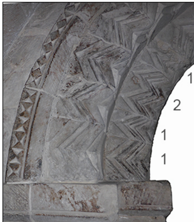
Plate 11: The north side of the chancel arch showing the irregularity of the chevron ornament (numbers indicates the number of chevrons per stone) and the change in the decoration of the label.
