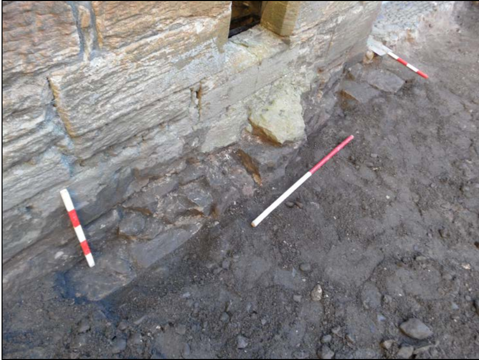
Plate 6: Looking south-east at the foundation course 306 and the ragged foundation course 307 of the east wall at the east door.
