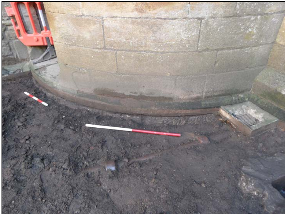
Plate 3: Looking south-east at the foundation course 206 of the south-east stair tower.
