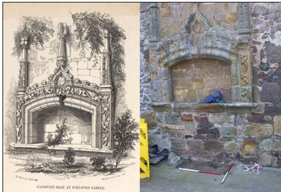
Figure 2: Robert Billings' drawing of the 'canopied seat' (left) alongside a current view, showing the dramatically altered level of the floor
