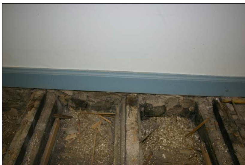
Nos. 078 and 079: View from north showing joist-stumps 078 and 079.
