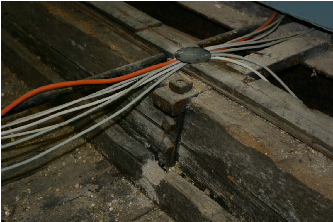
Figure 10: Iron bracket and partition at joist 050 (detail).
