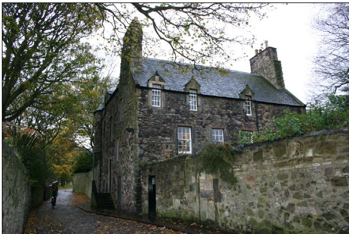
Figure 2: The North-Range of Croft-an-Righ House.
