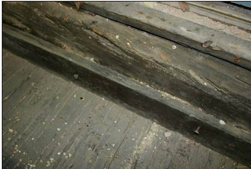
No. 081: View from northeast showing lathwork 081 at axis 16.
