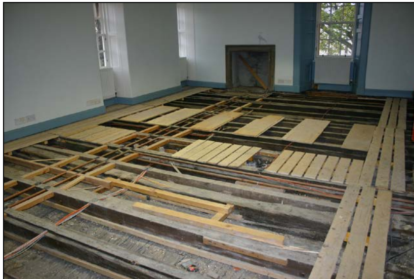
No. 030: View from northwest showing joist 030 (second axis from left).
