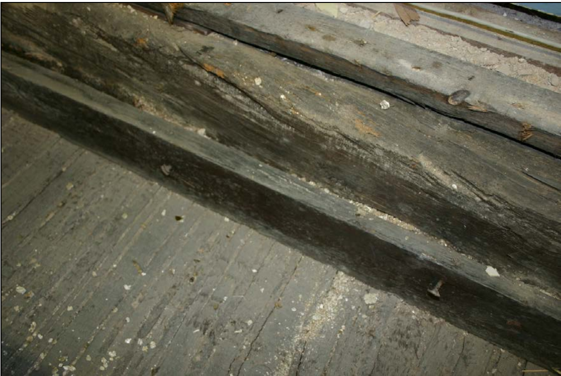
Figure 7: Auxiliary board, hand-made nails and lathwork at joist 057.
