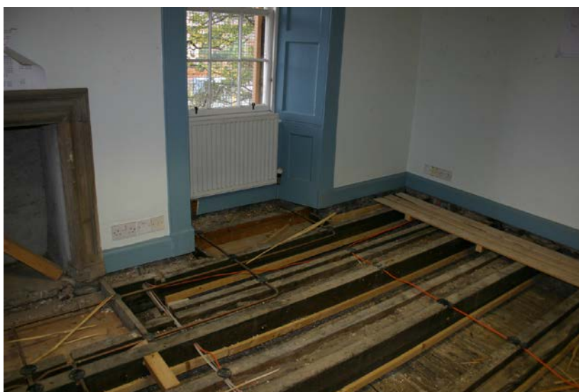
No.001: View from northwest showing auxiliary joist 001 (axis within window-bay).
