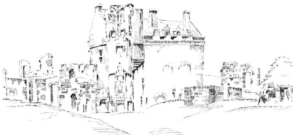
Figure 12: Nattes' view from the north-east, showing the intact roof of the Palace and the ruined range to the east.
