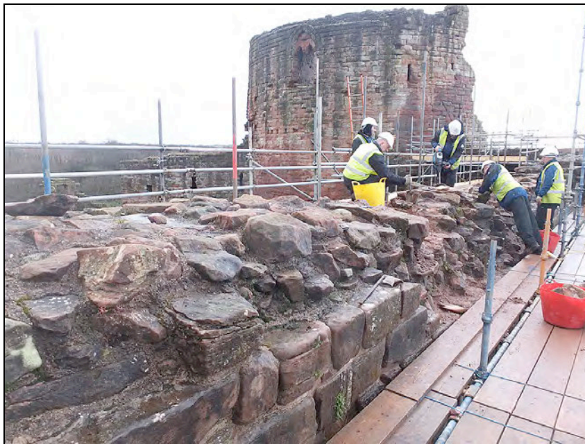
Plate 1: The exposed wall core
