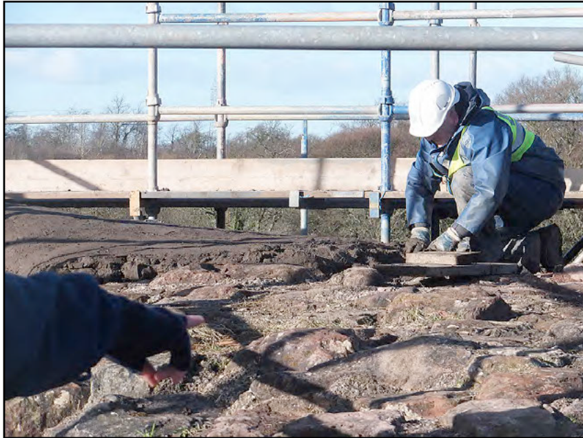
Plate 3: The installation of the soft clay
