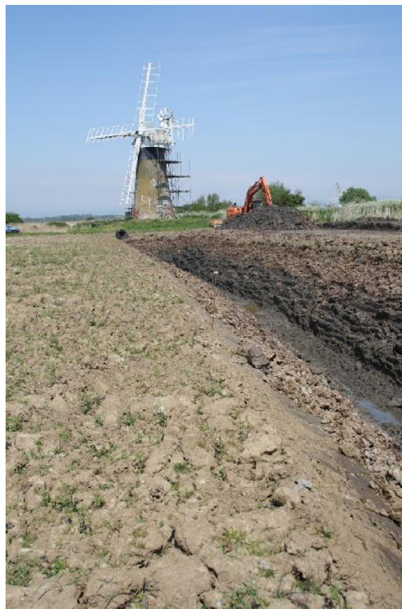
View of works
