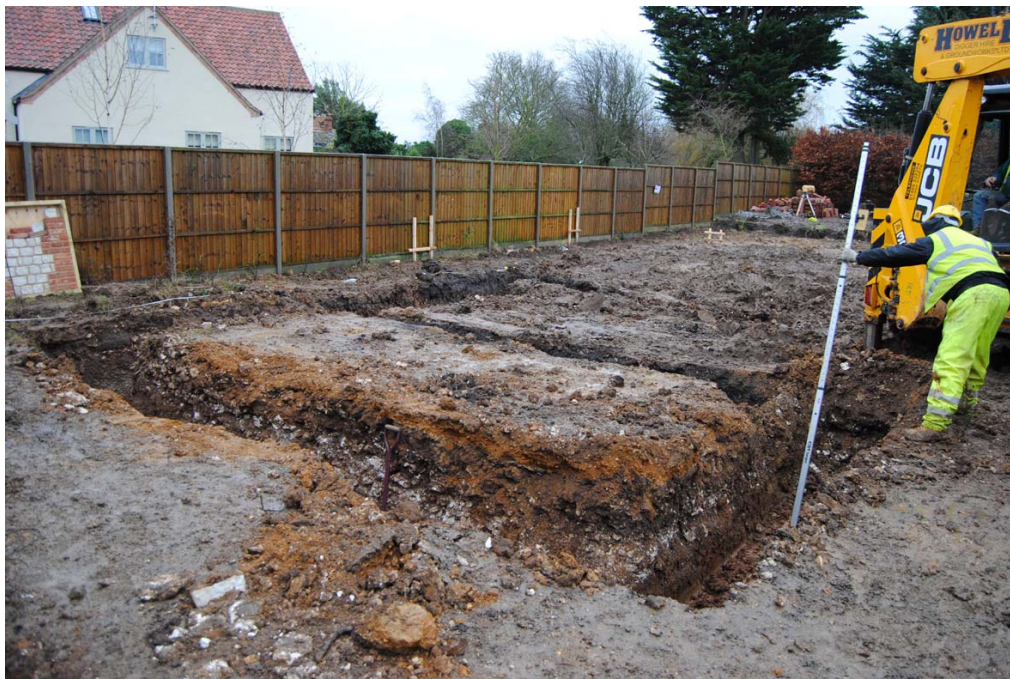
Plate 2. Showing chalk rubble make-up for driveway, looking south-east.
