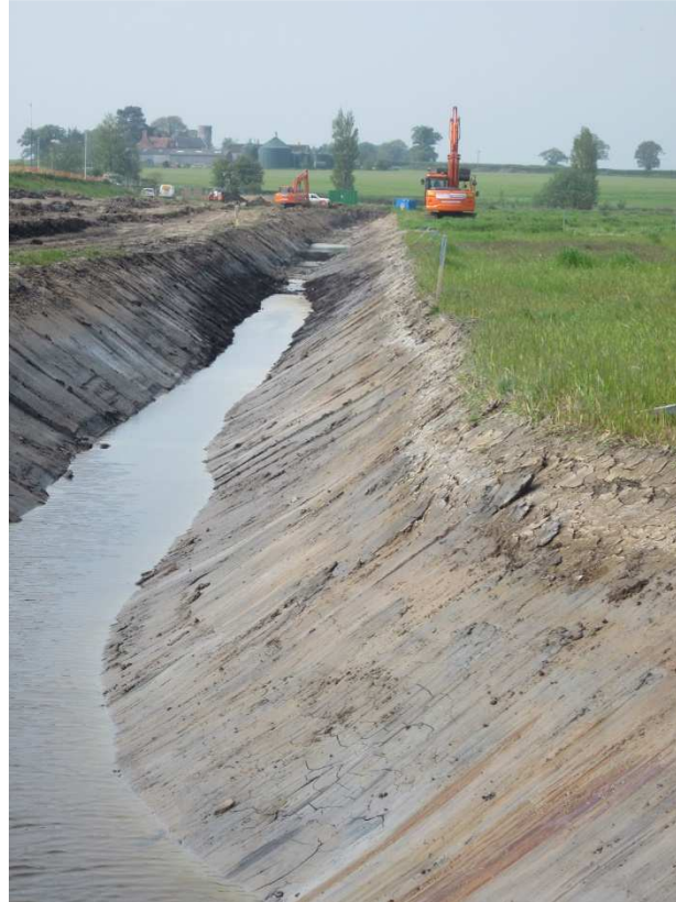
Plate 2. Showing unusual convex peat deposit. Looking south-west along new dyke parallel to Hardley Dyke.
